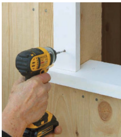
Trim the barn-sash opening with PVC. Install the angled sill first, followed by the casing legs. The casing overlaps the opening by \frac{3}{4} in.
