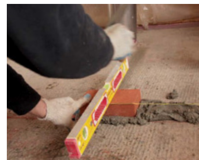
Work from the center out. Lay the end of the first brick for the hearth on the centerline, and level it both along its length and width.
