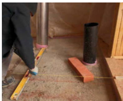
Mark the center. Measure off of the adjacent subfloor and mark the centerline of the firebox perpendicular to its front edge.
