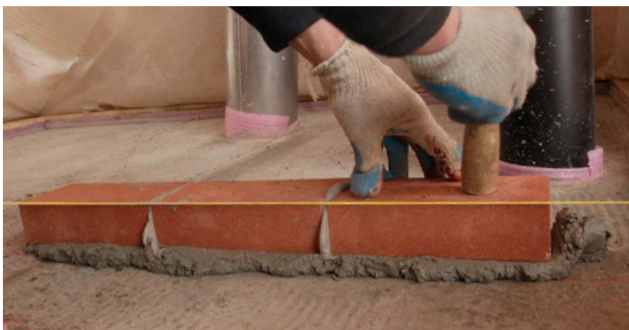
Line and stick. Use a stringline as a guide to keep the bricks in line and in plane as they're tapped down to the proper elevation.
