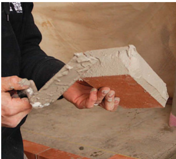
Don't get sloppy. Trowel on enough mortar to fill the joints—roughly \frac{1}{8} -in. thick—and bevel the edges to avoid excess squeeze-out.
