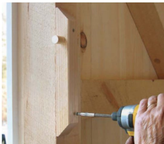
Install the barn-sash keepers. Screw foot-long pieces of 2-in.-thick pine, with \frac{3}{4} -in. dowels installed in them, to the inside of the posts. This provides a stop for the window sash when open.
