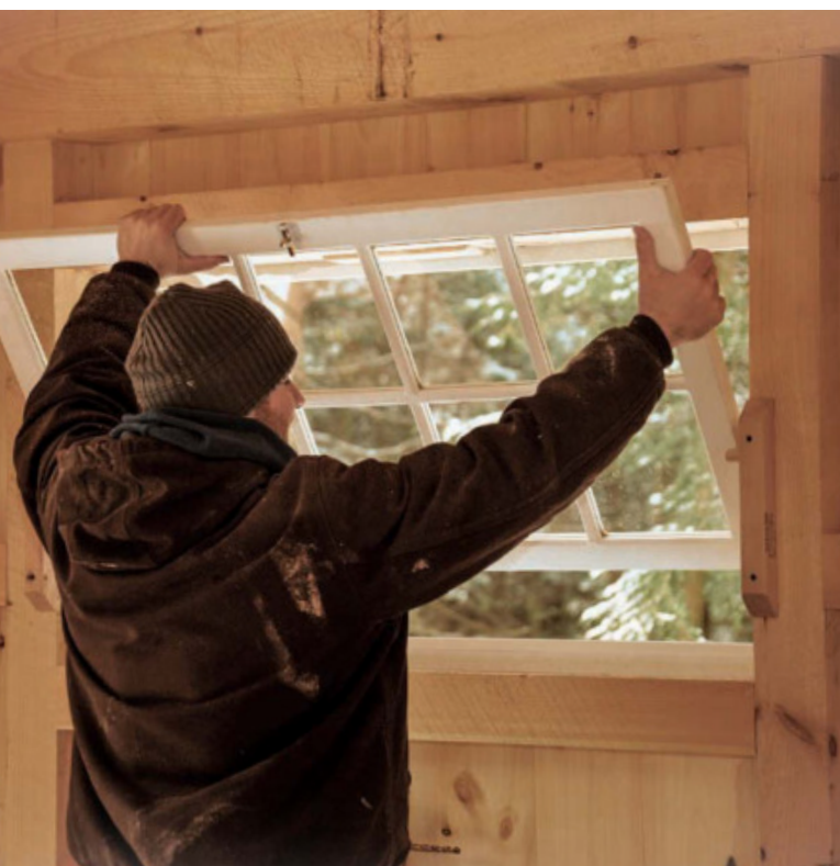
Set the sash. The barn sashes simply slip into place. A small barrel bolt at the top of each sash keeps it closed.
