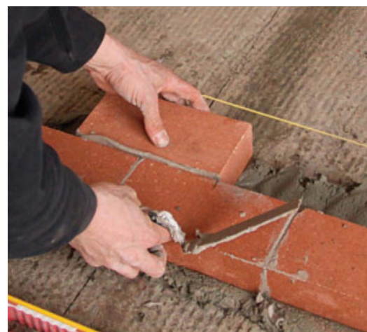
Stay on bond. Mark the center of a brick in the preceding course to help keep the bond pattern perfect. Keep joints tight at about \frac{1}{16} in.
