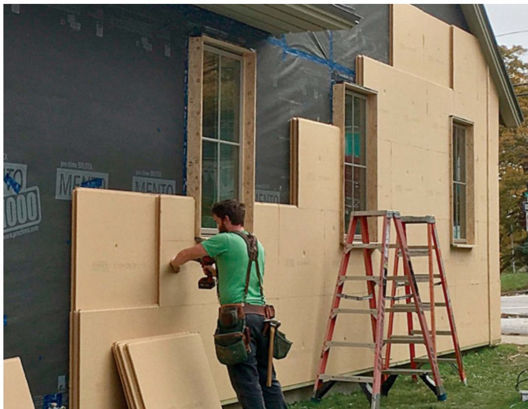
Dry board. Wood-fiber insulation is suitable for roof and wall assemblies. The two layers of 1 9 / 16 in. (R-11.6) Gutex Multitherm shown here are vapor-open and waterproof.
