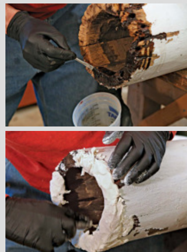
Two-step repair. Epoxy putty is typically applied after a soaking coat of wood consolidant, which reinforces damaged wood.
