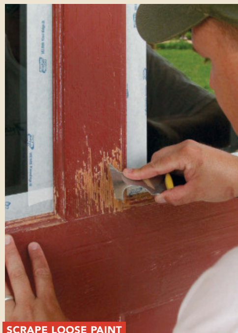
SCRAPE LOOSE PAINT
