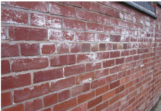
Fig. 264 Efflorescence.
