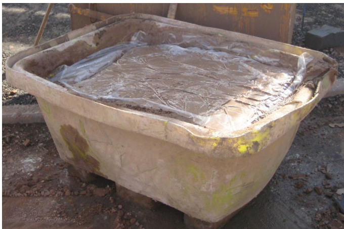
Fig. 24 Ready-mix mortar delivered to site.
