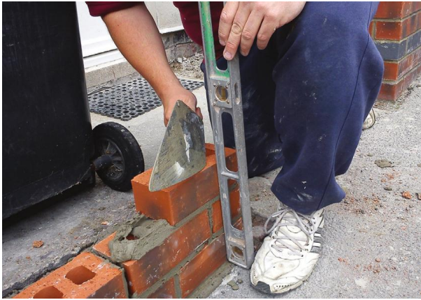
Fig. 129 It is important to spend enough time getting the first three courses spot on for plumb.
