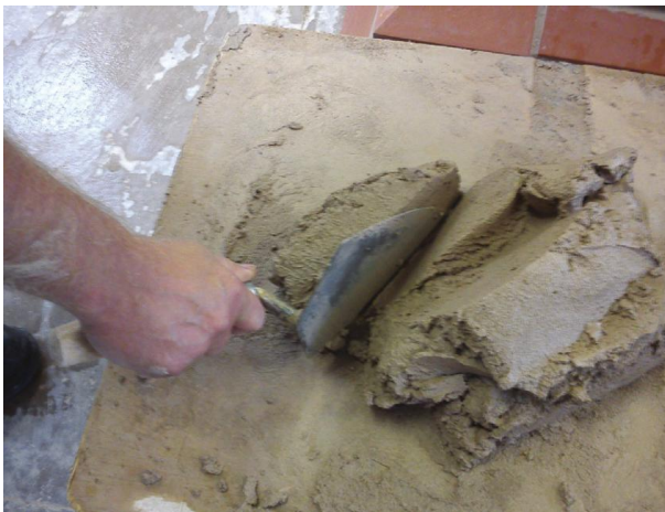
Fig. 107 Cutting mortar.
