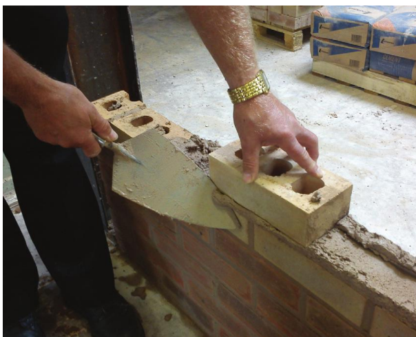
Fig. 116 Trimming off excess mortar from the bed joint.
