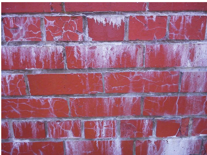
Fig. 265 Lime staining.
