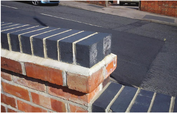
Fig. 223 An oversailing course can be extended to provide a weathering at a stopped-end.
