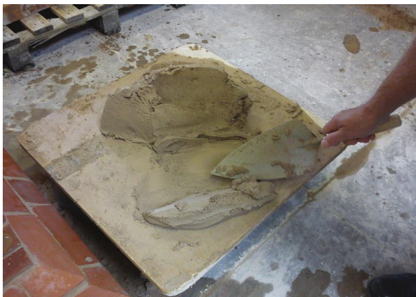
Fig. 109 Preparation for picking up the mortar.
