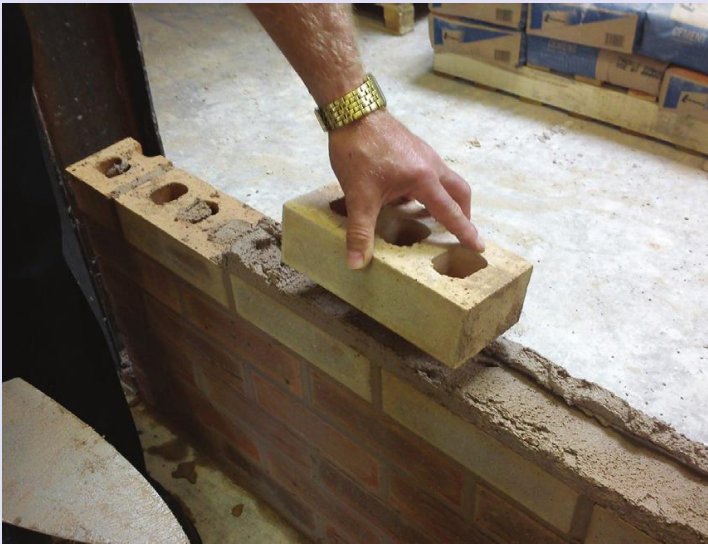
Fig. 114 The correct way to hold a brick.
