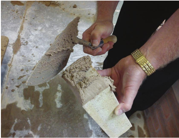
Fig. 120 Completing the cross-joint.
