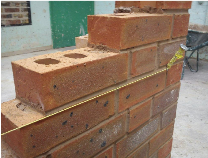
Fig. 134 Lines and pins in use.
