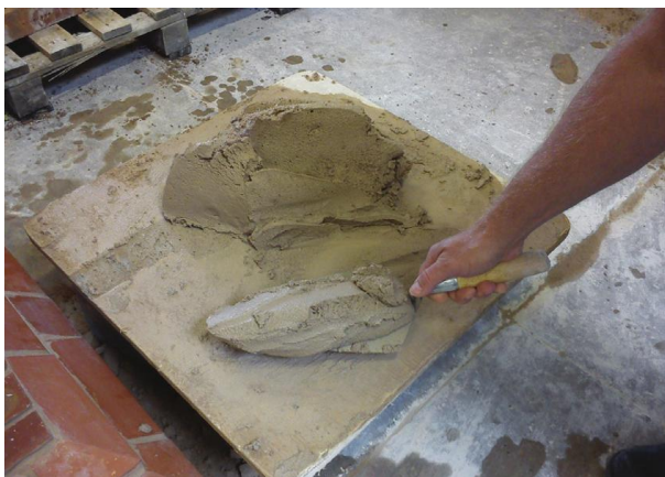
Fig. 110 Picking up the mortar.
