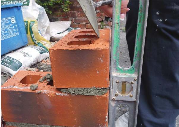
Fig. 130 A lining the quoin brick to plumb.
