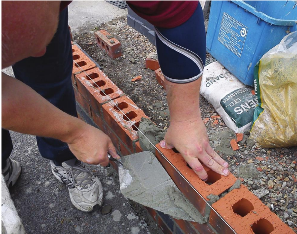
Fig. 133 Laying bricks to a string-line – ‘feeling’ with the trowel blade whether the brick is flush with the course below.
