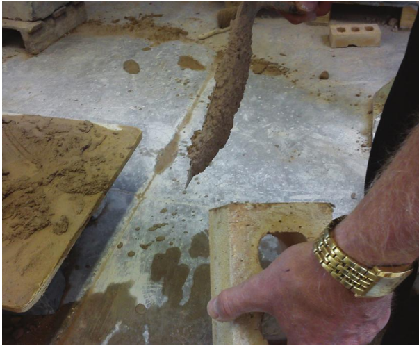
Fig. 117 Preparing to apply a cross-joint.
