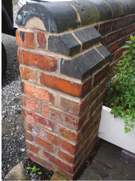
Fig. 234 Pier terminated below the top of an old wall using plinth bricks to form a ‘tumbling in’.
