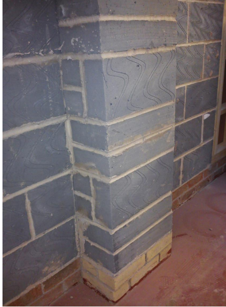
Fig. 104 Attached pier in blockwork.
