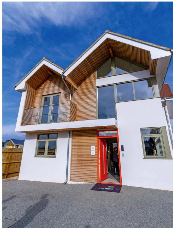
Left: A joint project, Build It's Self Build Education House also doubles up as the Marketing Suite for Graven Hill
