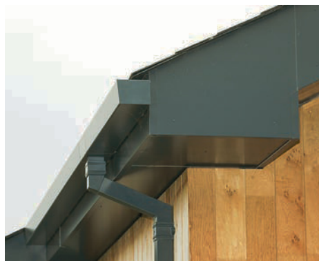
Images show Marley Alutec's Evoke fascia & soffit system and Alligator Boxer at Chapel View in Goudhurst, Kent
