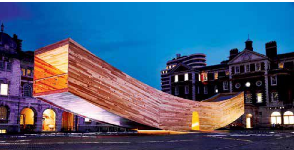
'The Smile' (left) is the first project in the world to use large hardwood CLT panels. A cross-section of the Tulipwood CLT (right).
