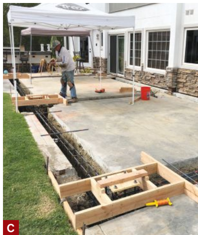
Figure 1. A 12-inch-wide slot was cut through the concrete patio for the new grade-beam footing engineered to provide lateral support for the freestanding deck (A). The rebar cages were partially assembled, then delivered to the site (B), where the crew finished tying them together after the steel reinforcement was placed in the 24-inch-deep trenches. The crew carefully formed up the piers for the deck's steel support columns to ensure that the deck ended up at the proper elevation (C). Rebar dowels were added to the cut edges of the patio to tie the concrete slab to the grade beam after the new concrete was poured (D). Before the steel columns were installed, nuts were threaded onto each of the pier's four anchor bolts, which would later be used to fine-tune the height of the columns and adjust them for plumb (E).
