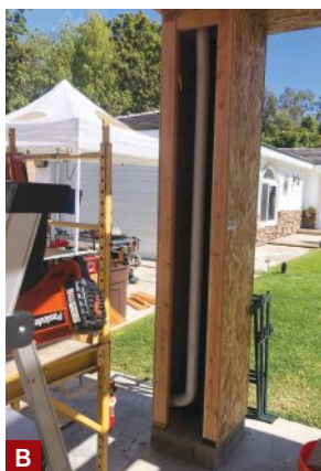
Figure 4. Water collected by the under-deck drain system flows toward the outside edge of the deck, where it empties into a one-piece gutter (A). The gutter slopes toward a corner column, where it is drained by a 3-inch-diameter downspout concealed within the boxed column (B). Trex RainEscape downspouts (C) empty the water collected by the troughs, which are draped over the tops of the joists (D). At the house, a custom-fabricated flashing and weep screed tie the WRB behind the stucco to the deck waterproofing system.
