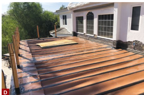
Figure 4. Water collected by the under-deck drain system flows toward the outside edge of the deck, where it empties into a one-piece gutter (A). The gutter slopes toward a corner column, where it is drained by a 3-inch-diameter downspout concealed within the boxed column (B). Trex RainEscape downspouts (C) empty the water collected by the troughs, which are draped over the tops of the joists (D). At the house, a custom-fabricated flashing and weep screed tie the WRB behind the stucco to the deck waterproofing system.
