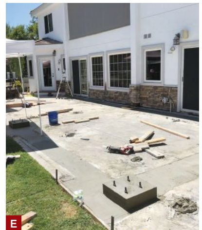
Figure 1. A 12-inch-wide slot was cut through the concrete patio for the new grade-beam footing engineered to provide lateral support for the freestanding deck (A). The rebar cages were partially assembled, then delivered to the site (B), where the crew finished tying them together after the steel reinforcement was placed in the 24-inch-deep trenches. The crew carefully formed up the piers for the deck's steel support columns to ensure that the deck ended up at the proper elevation (C). Rebar dowels were added to the cut edges of the patio to tie the concrete slab to the grade beam after the new concrete was poured (D). Before the steel columns were installed, nuts were threaded onto each of the pier's four anchor bolts, which would later be used to fine-tune the height of the columns and adjust them for plumb (E).
