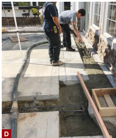
Figure 1. A 12-inch-wide slot was cut through the concrete patio for the new grade-beam footing engineered to provide lateral support for the freestanding deck (A). The rebar cages were partially assembled, then delivered to the site (B), where the crew finished tying them together after the steel reinforcement was placed in the 24-inch-deep trenches. The crew carefully formed up the piers for the deck's steel support columns to ensure that the deck ended up at the proper elevation (C). Rebar dowels were added to the cut edges of the patio to tie the concrete slab to the grade beam after the new concrete was poured (D). Before the steel columns were installed, nuts were threaded onto each of the pier's four anchor bolts, which would later be used to fine-tune the height of the columns and adjust them for plumb (E).
