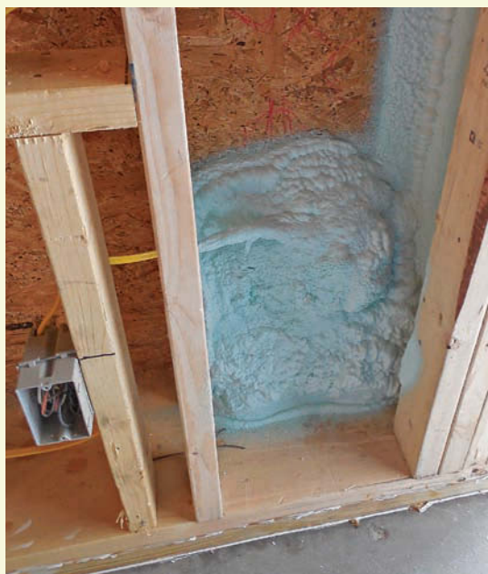
Cellulose belt, spray-foam suspenders. Although primarily insulated with dense-pack cellulose, all penetrations are coated first with spray polyurethane foam, and all seams in wall plates are sealed with a bead of caulk.
