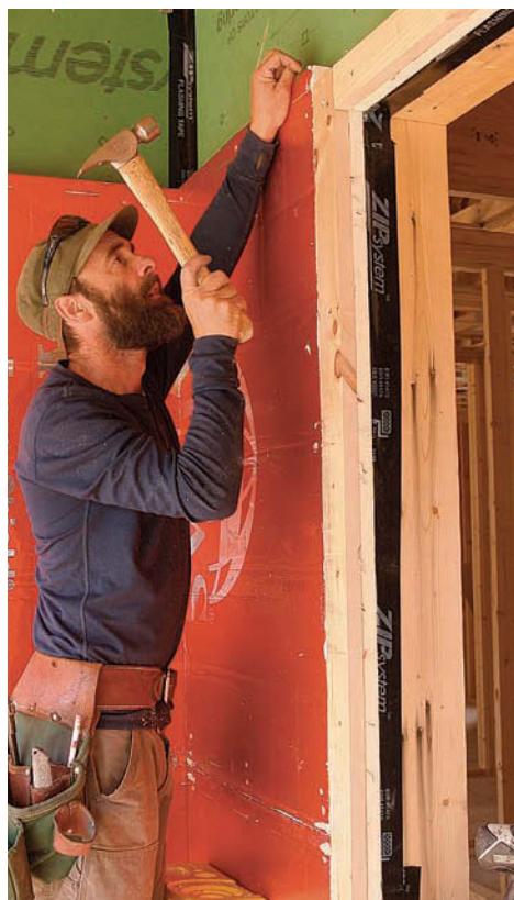
Butt the wall foam to the build-out. Installation of the rest of the insulation is simply a matter of cutting to fit and fastening with 2½-in. roofing nails.
