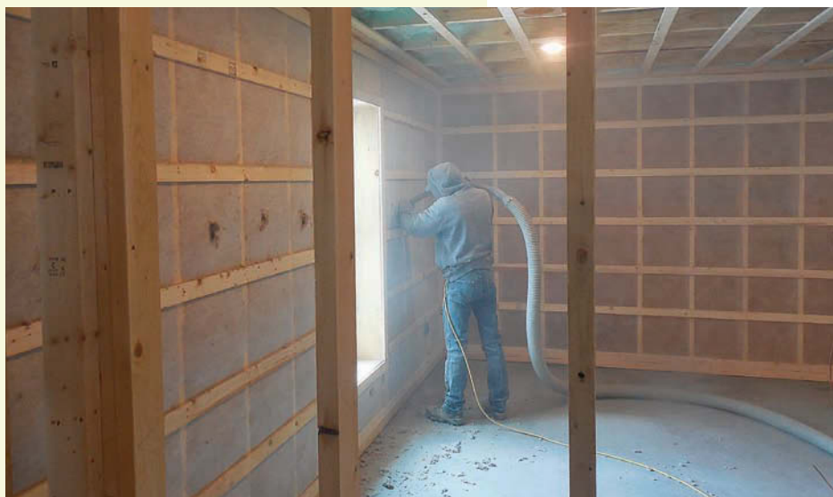
Cellulose belt, spray-foam suspenders. Although primarily insulated with dense-pack cellulose, all penetrations are coated first with spray polyurethane foam, and all seams in wall plates are sealed with a bead of caulk.
