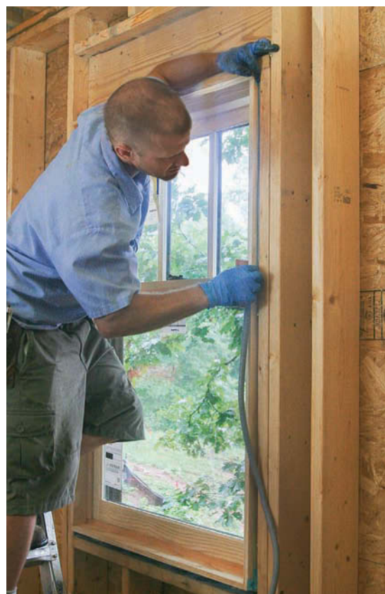
A caulk joint that will last. Foam backer rod cut and pressed in around the window jamb creates a flexible base for the bead of caulk that follows it. Use a wet finger to smooth the bead against the backer rod, creating the ideal hour-glass shape that allows the sealant to expand and contract without cracking or debonding.
