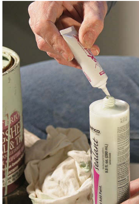
Add activator to the tube and shake. The activator causes the caulk, which is very liquid until now, to thicken.
