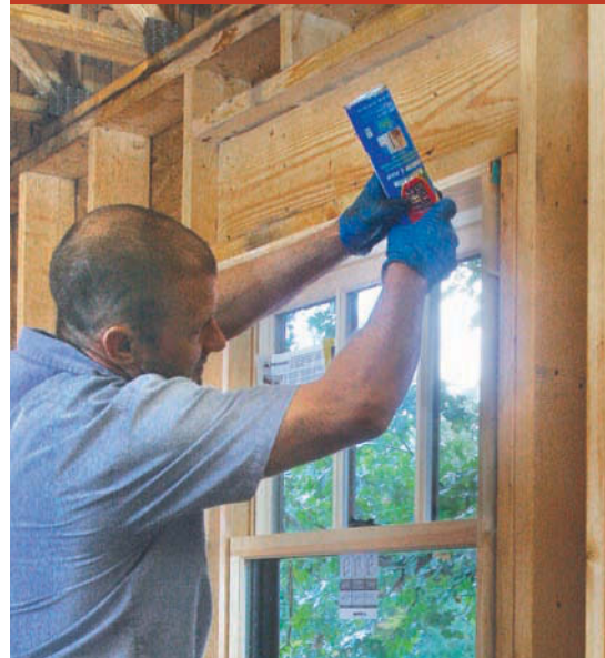
A conservative bead of foam. A thin bead of low-expansion spray foam offers limited air-sealing and insulation, but avoid filling the entire cavity, especially toward the bottom, to allow for drainage in the case of water entry.
