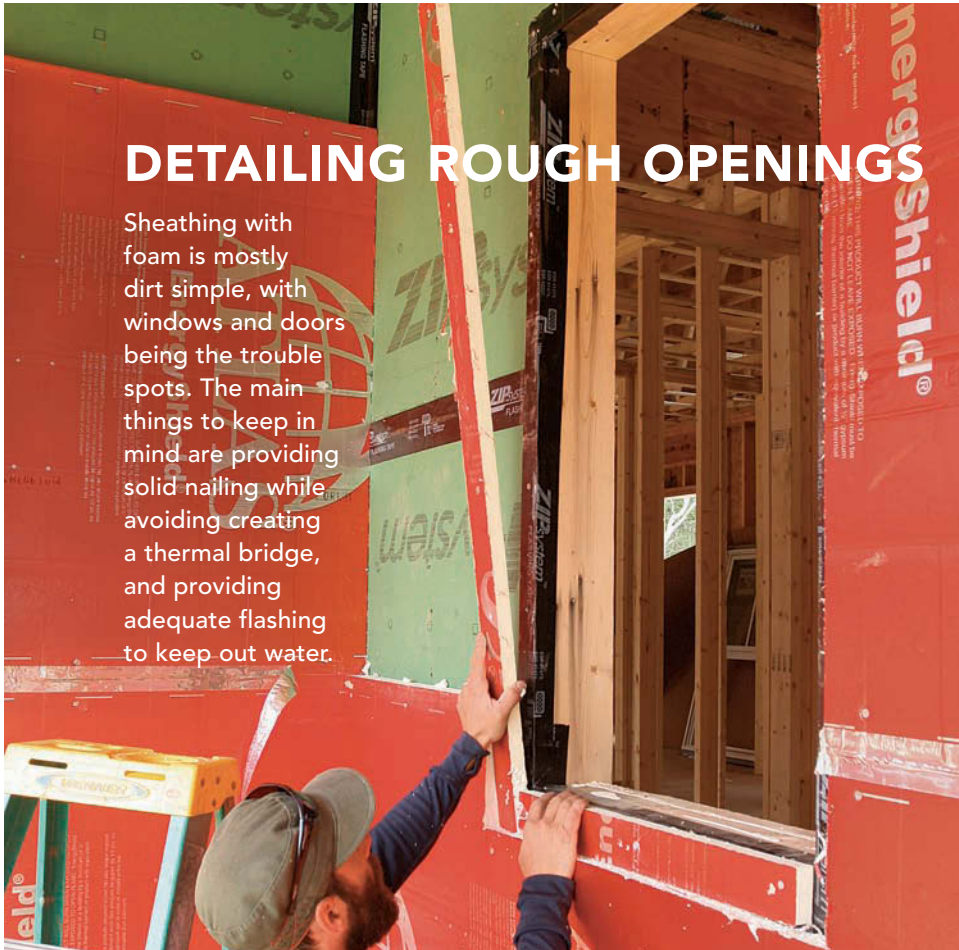
Create a thermal break. Nail foam strips 1 in. thick and 3½ in. wide around the opening.
