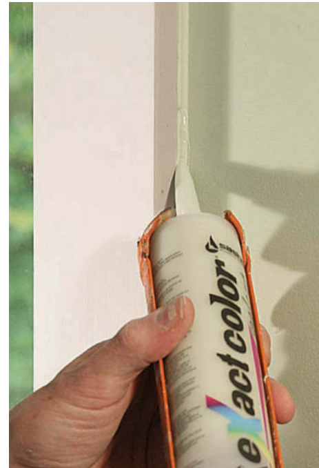
Caulk neatly. After allowing 30 minutes for the activator to thicken the caulk to a normal consistency, fill the joint.
