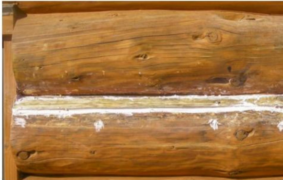
Decay removed and replaced with sound timber.
