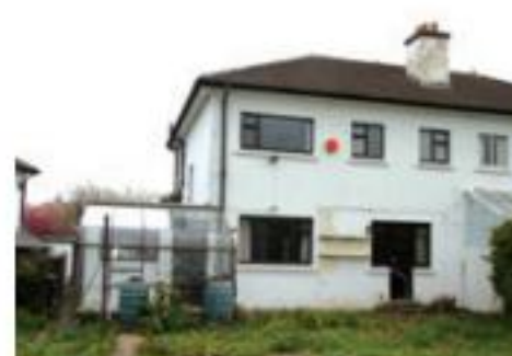
Above: Front of house before, below: back of house before
