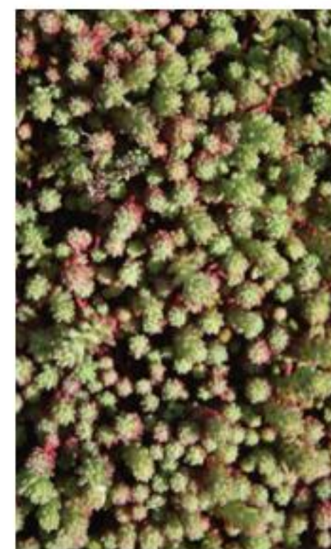
Sedum is a type of succulent used on extensive roofs.
