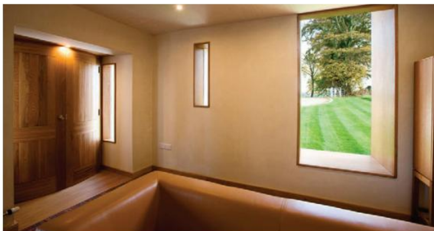
Birch faced paneling was used on some of the ceilings.
