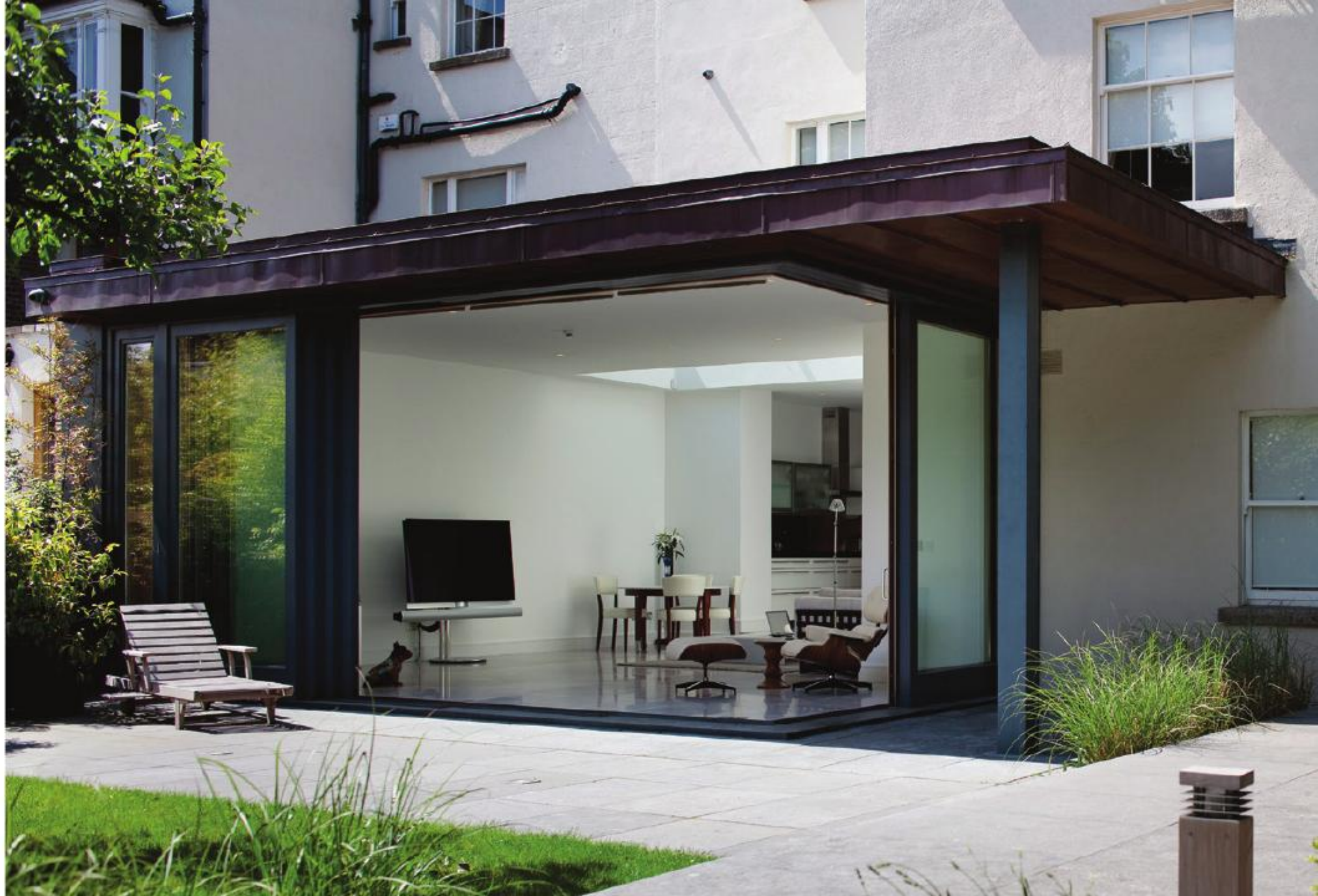
Connection between existing house and new extension with a lightbox located at the junction of the two spaces drawing in natural light
