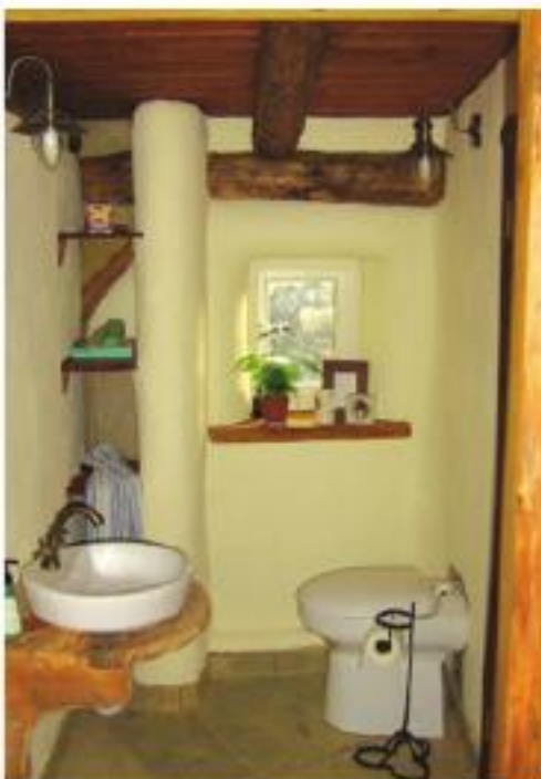
Dry toilet positioned over collection chamber
