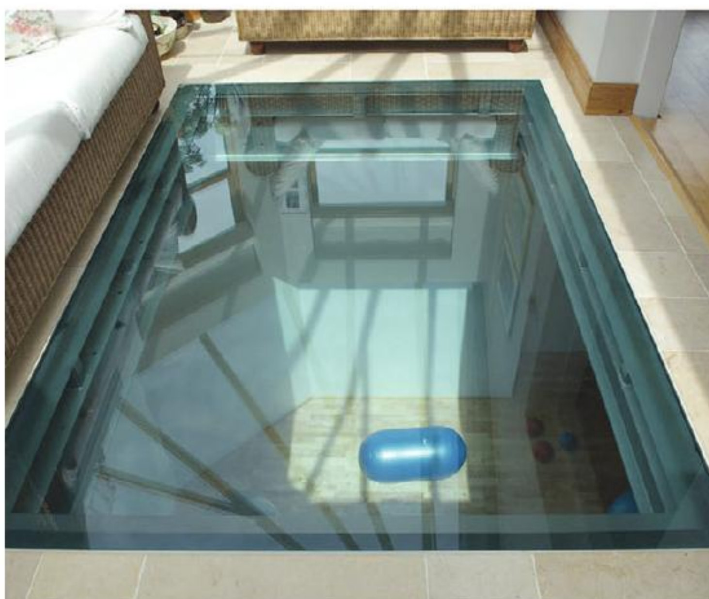
Glass floor looking down into converted basement (above left) Therm onex Ltd
