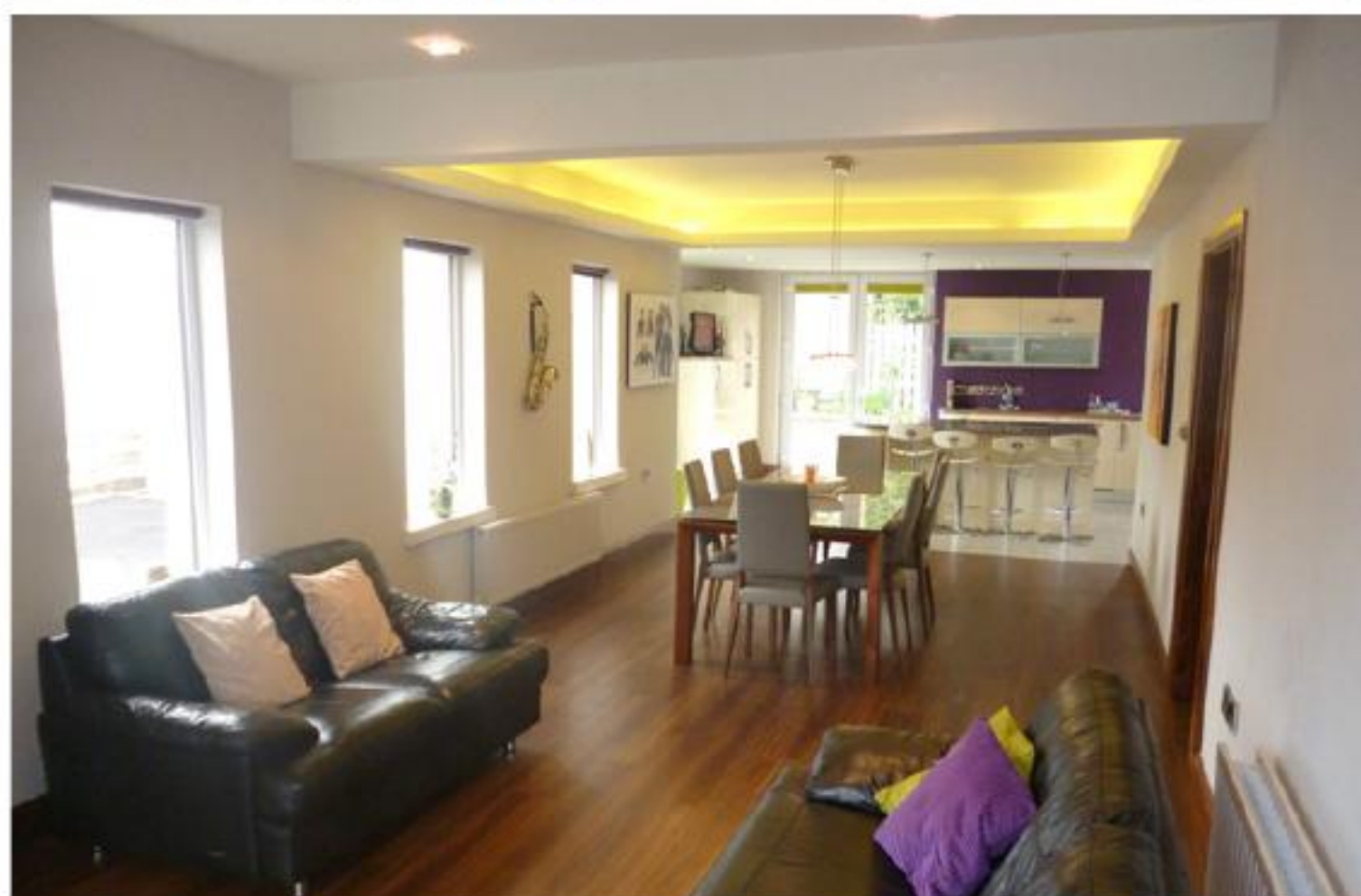
Opening made at the steel juncture; lowered ceiling provides separation and hides the beam.
