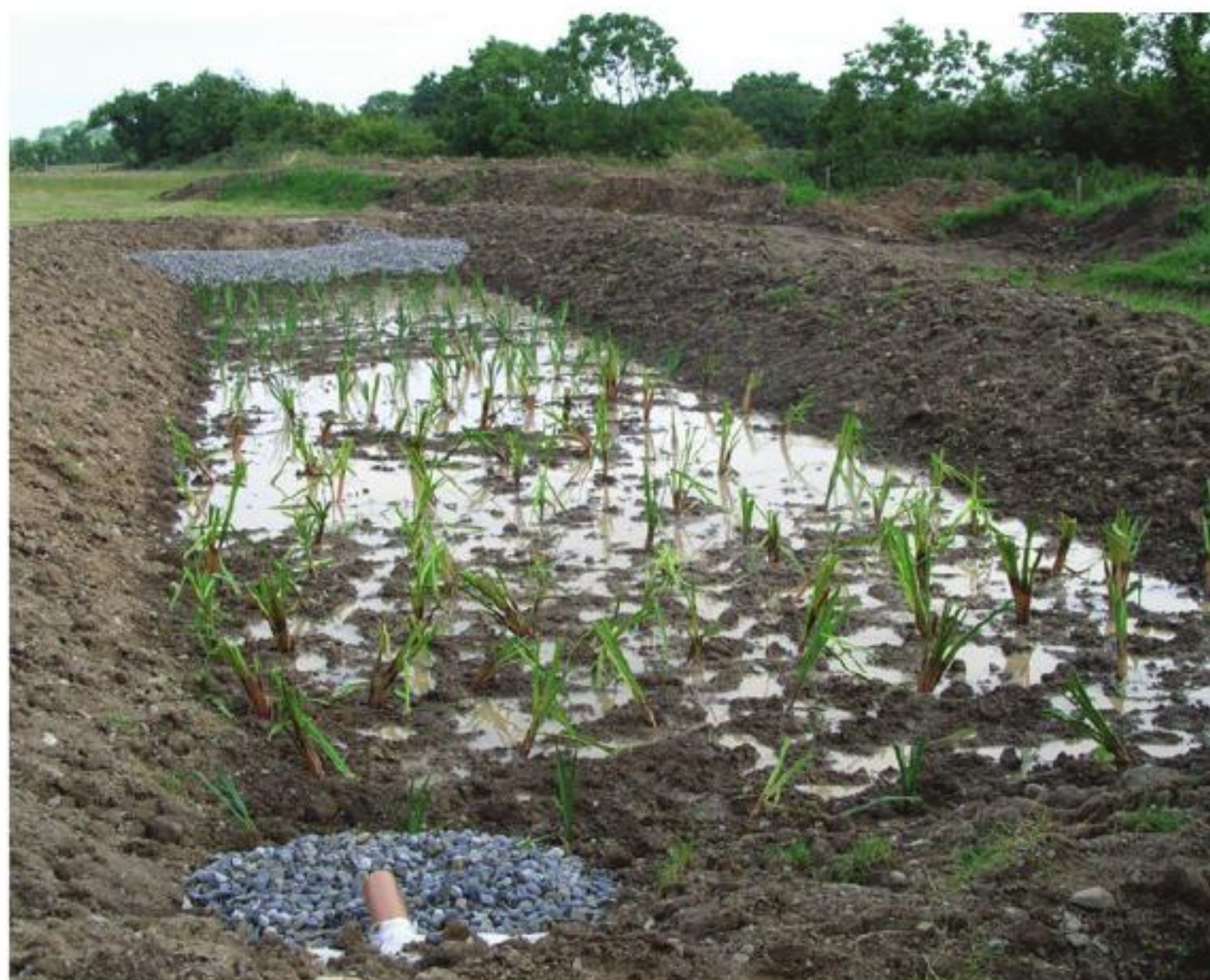
Newly planted constructed wetland
