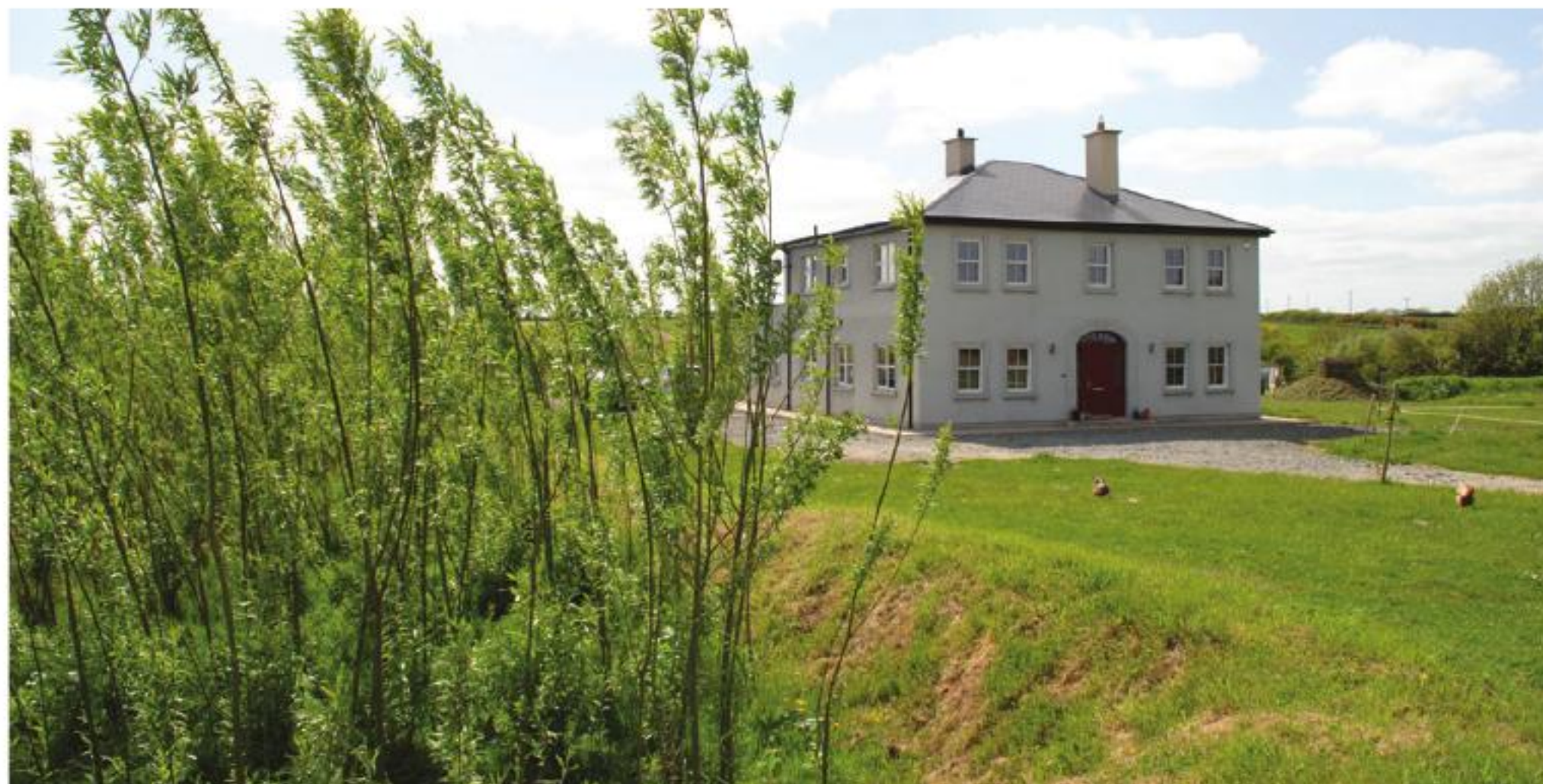
The land provided no percolation to speak of and we were miles away from mains waste removal
