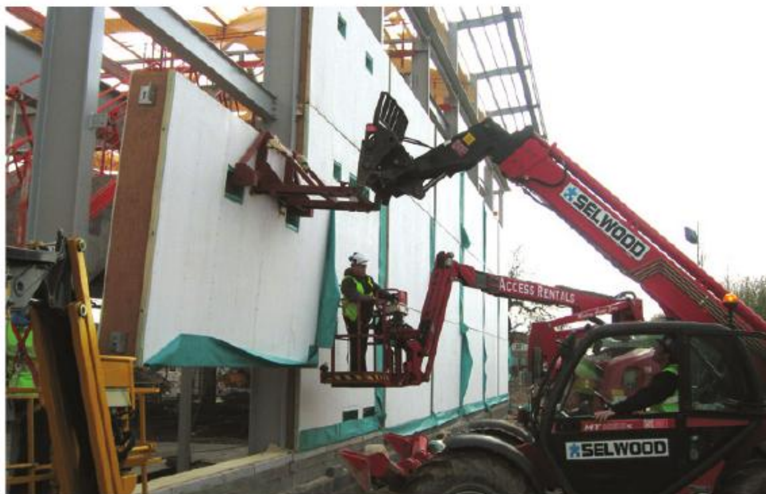
Hemclad panels installed, Cheshire Oaks, Ellesmere Port, UK.
