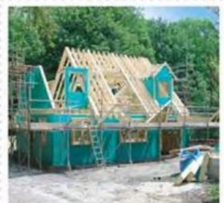
Watertight Frame Erection
