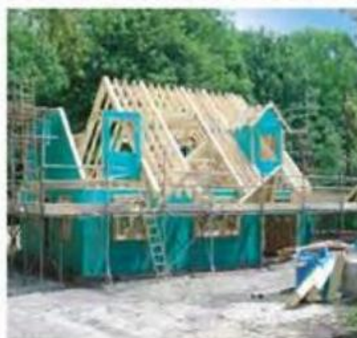
Watertight Frame Erection
