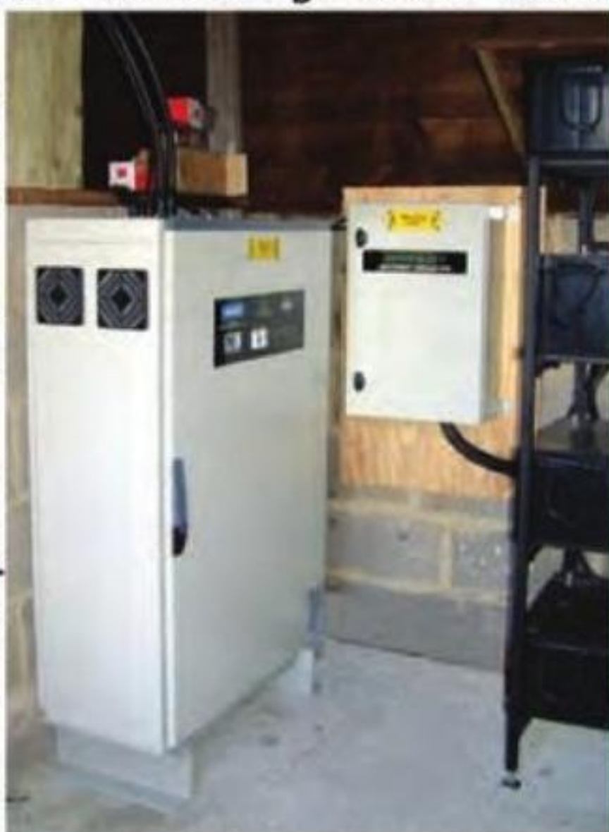
PS SYSTEM INSTALLATION
