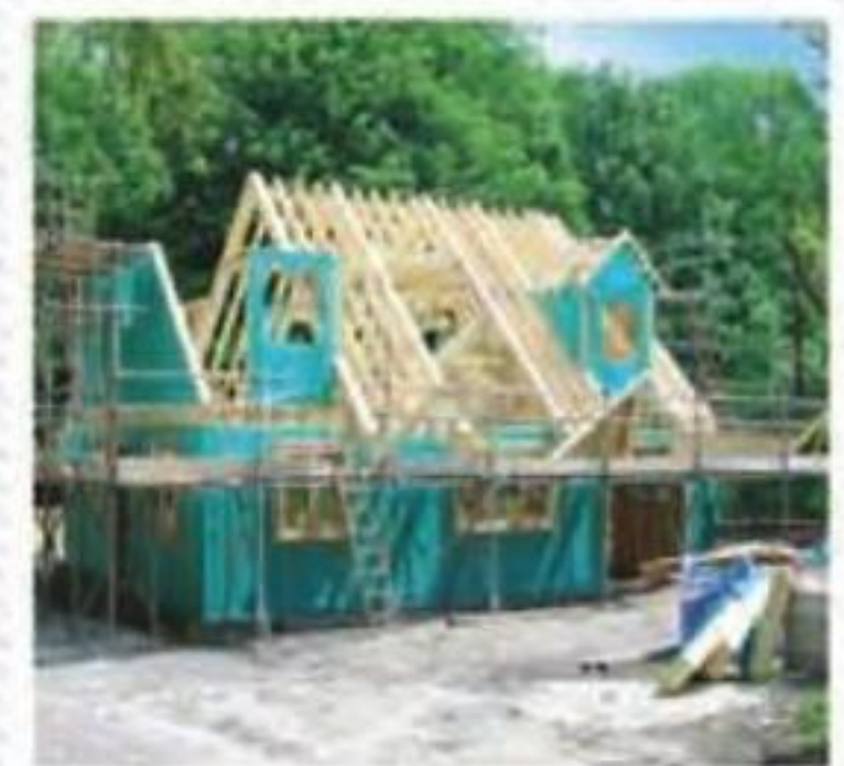
Watertight Frame Erection
