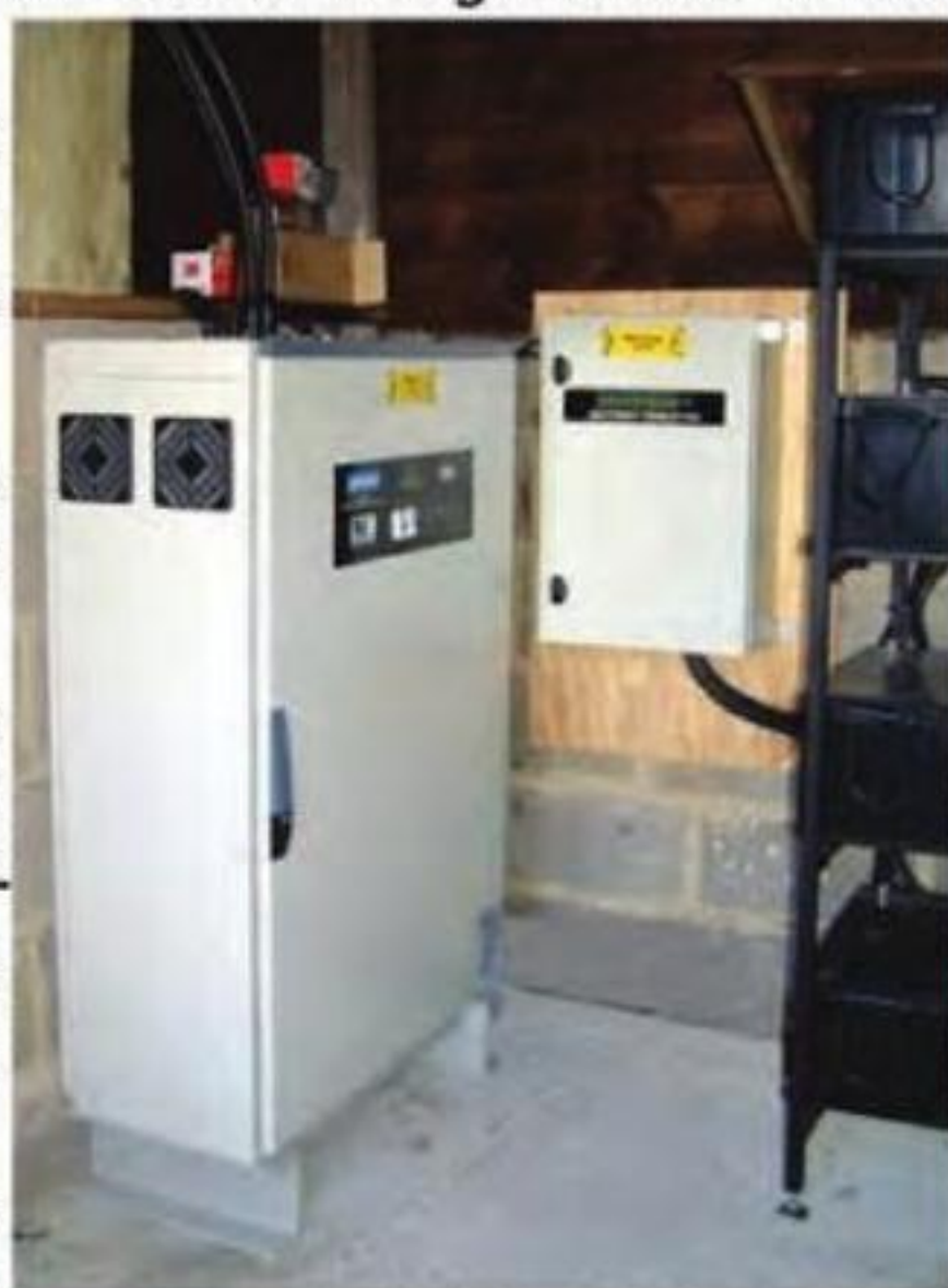
PS SYSTEM INSTALLATION
