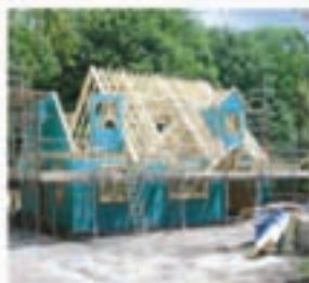
Watertight Frame Erection
