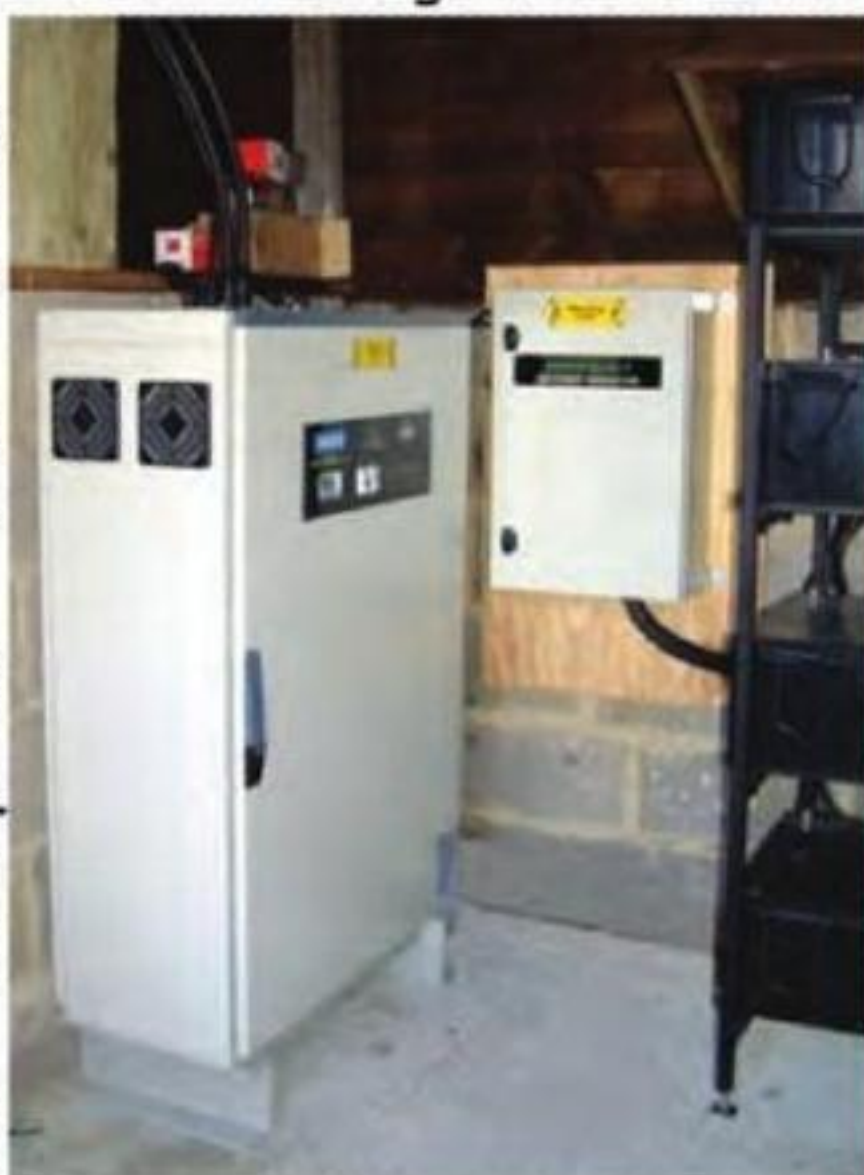
PS SYSTEM INSTALLATION
