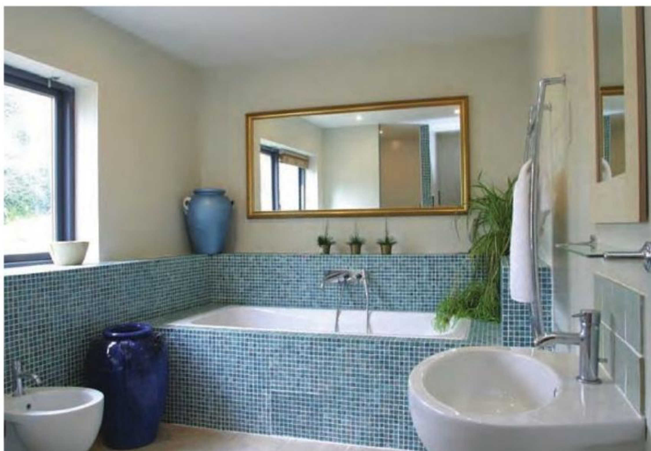
Passive stack ventilation extracts the humidity from the wet bathrooms.
