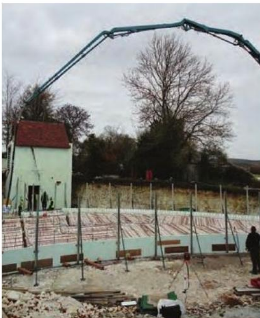
Pouring the concrete for the foundations.
