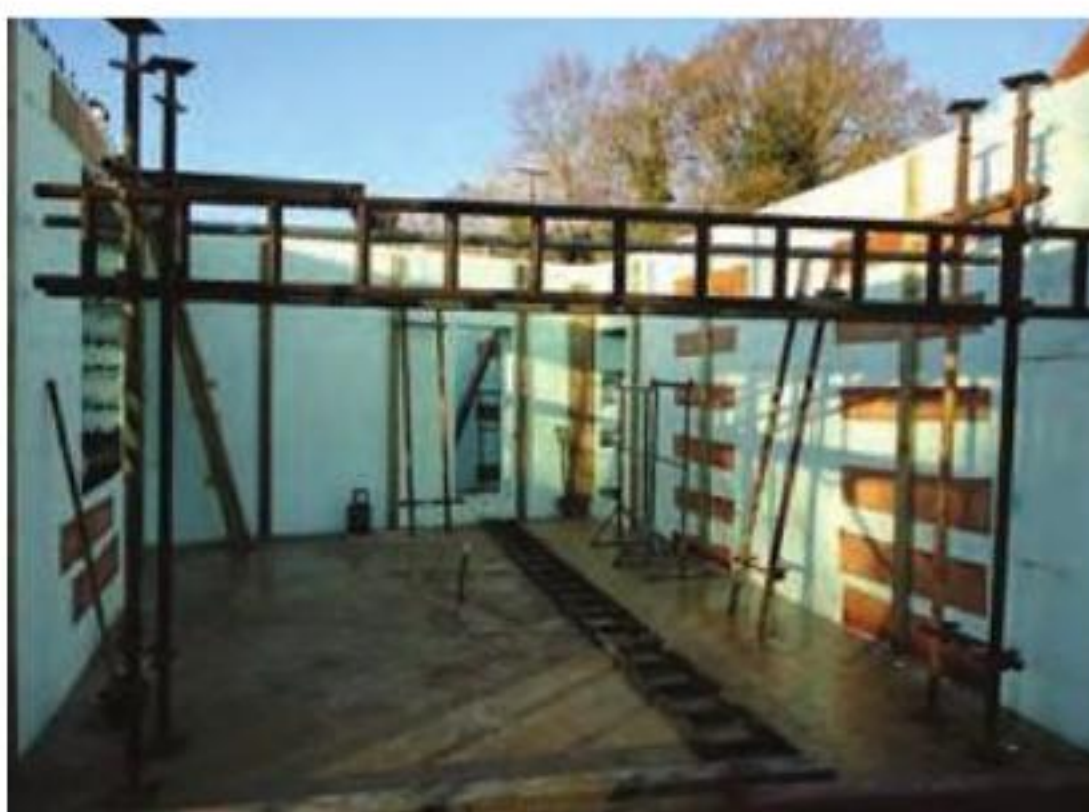
Plywood gussets can be clearly seen strengthening the joints.
