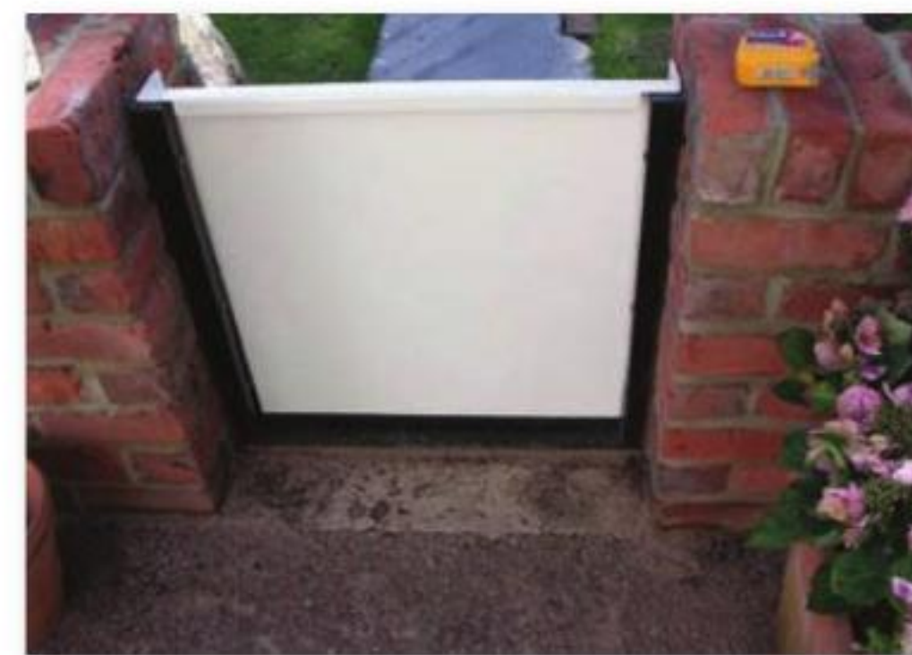
REMOVABLE FLOOD DOOR BUILT INTO GARDEN WALL GATEWAY
