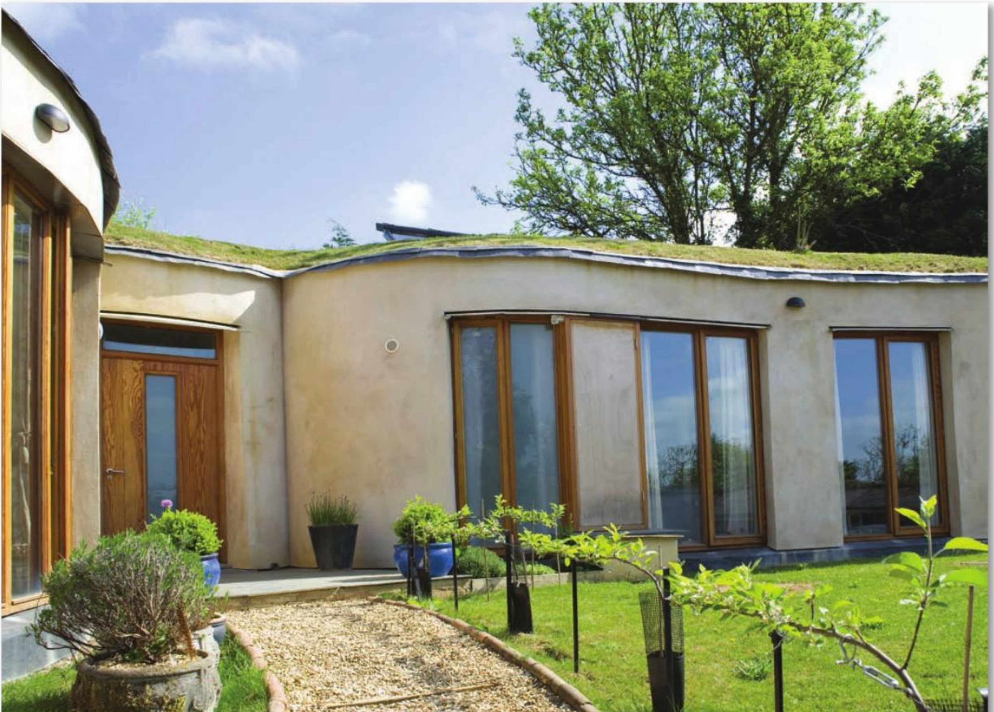
THE CURVED WALLS HAVE A RENDERED, 'FLOATING' INSULATION LAYER
