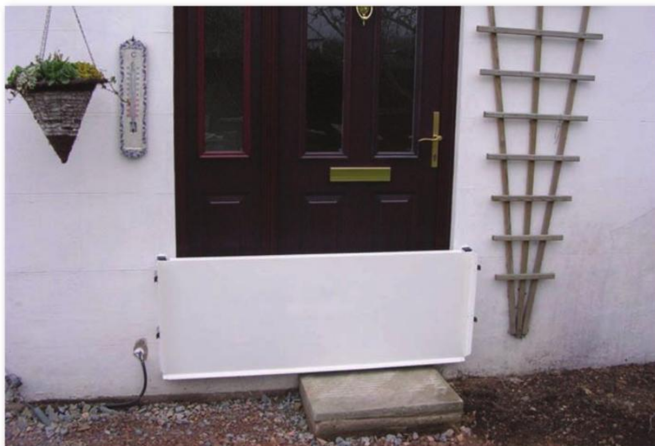
REMOVABLE FLOOD DOOR CLIPPED ONTO A PERMANENTLY INSTALLED FRAME PROTECTING A FRONT DOOR
