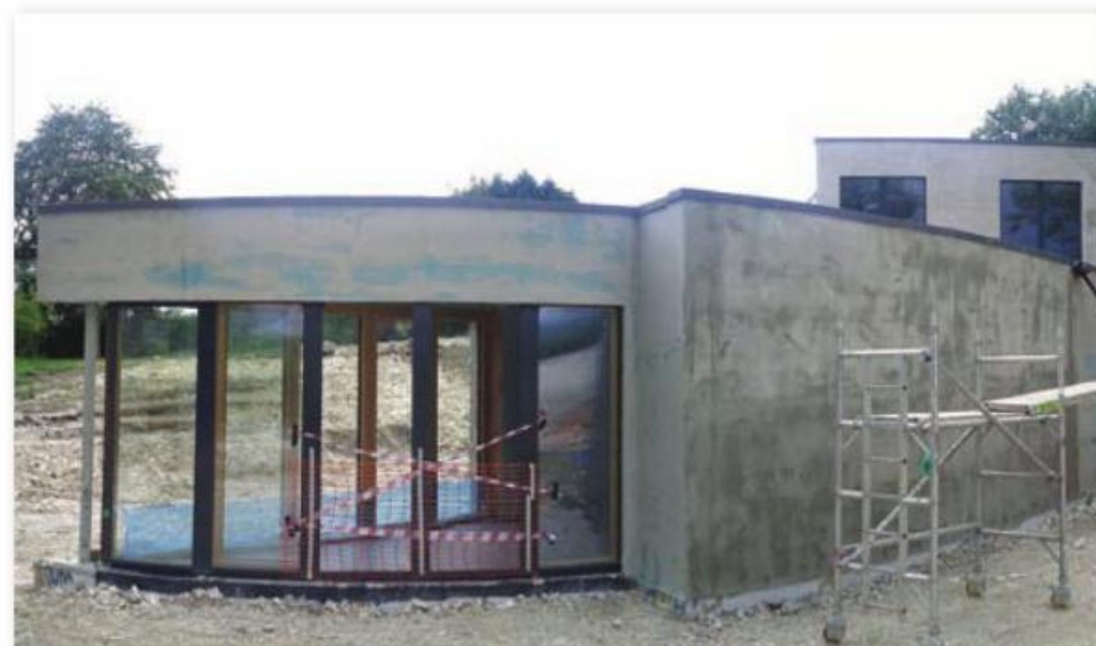
FIRST COAT OF RENDER APPLIED TO THE EXTERIOR
