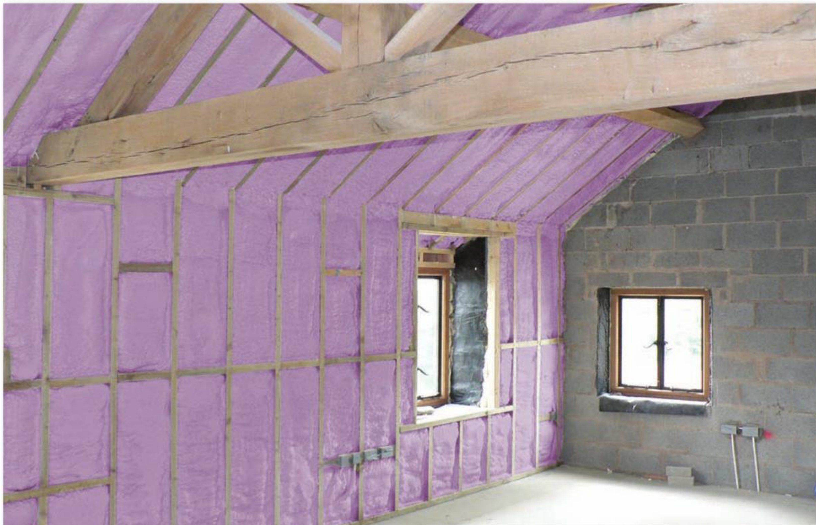
INTERNAL ROOF AND WALLS - TYN Y DDOL RUTHIN
