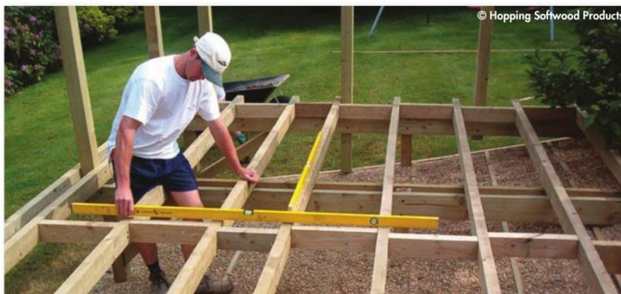
CHECKING LEVEL ON JOISTS
