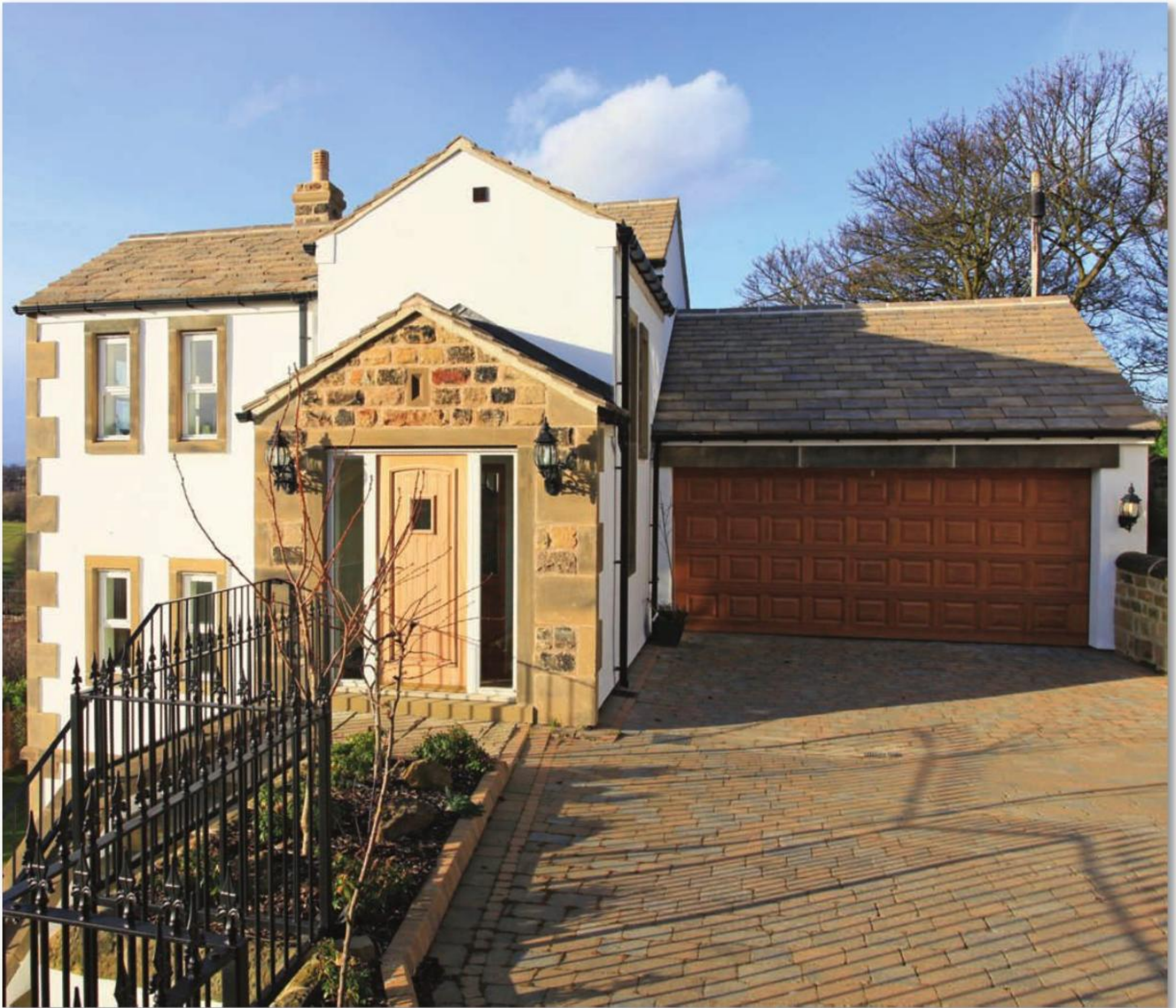
RETAINING WALLS SET INTO THE HILLSIDE ACCOMMODATE THE STEEP THREE-STOREY STRUCTURE AND KEEP THE ROOFLINE AS LOW AS POSSIBLE
