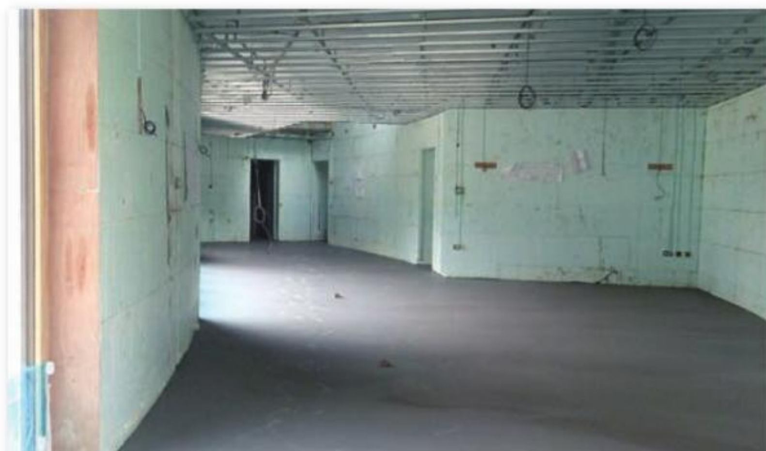
LOUNGE – DINING ROOM WITH THE NEW SCREED
