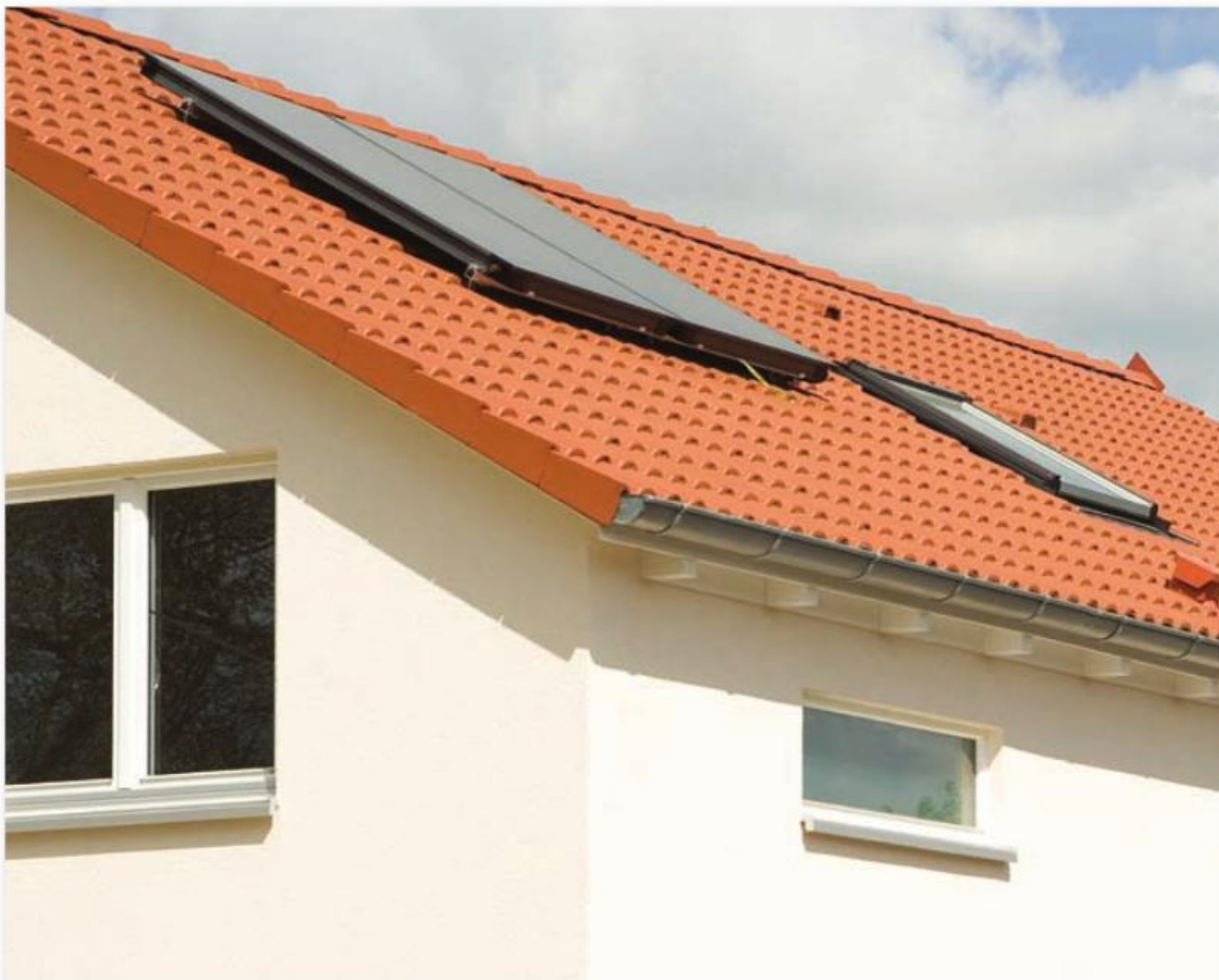
SOLAR WATER HEATING ON THE SOUTH-FACING ROOF HAS NOW BEEN JOINED BY A PHOTOVOLTAIC ARRAY
