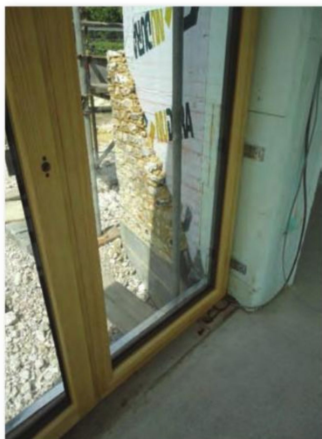
THE NEW KNAPPED FLINT FACADE VIEWED THROUGH THE WINDOW.
