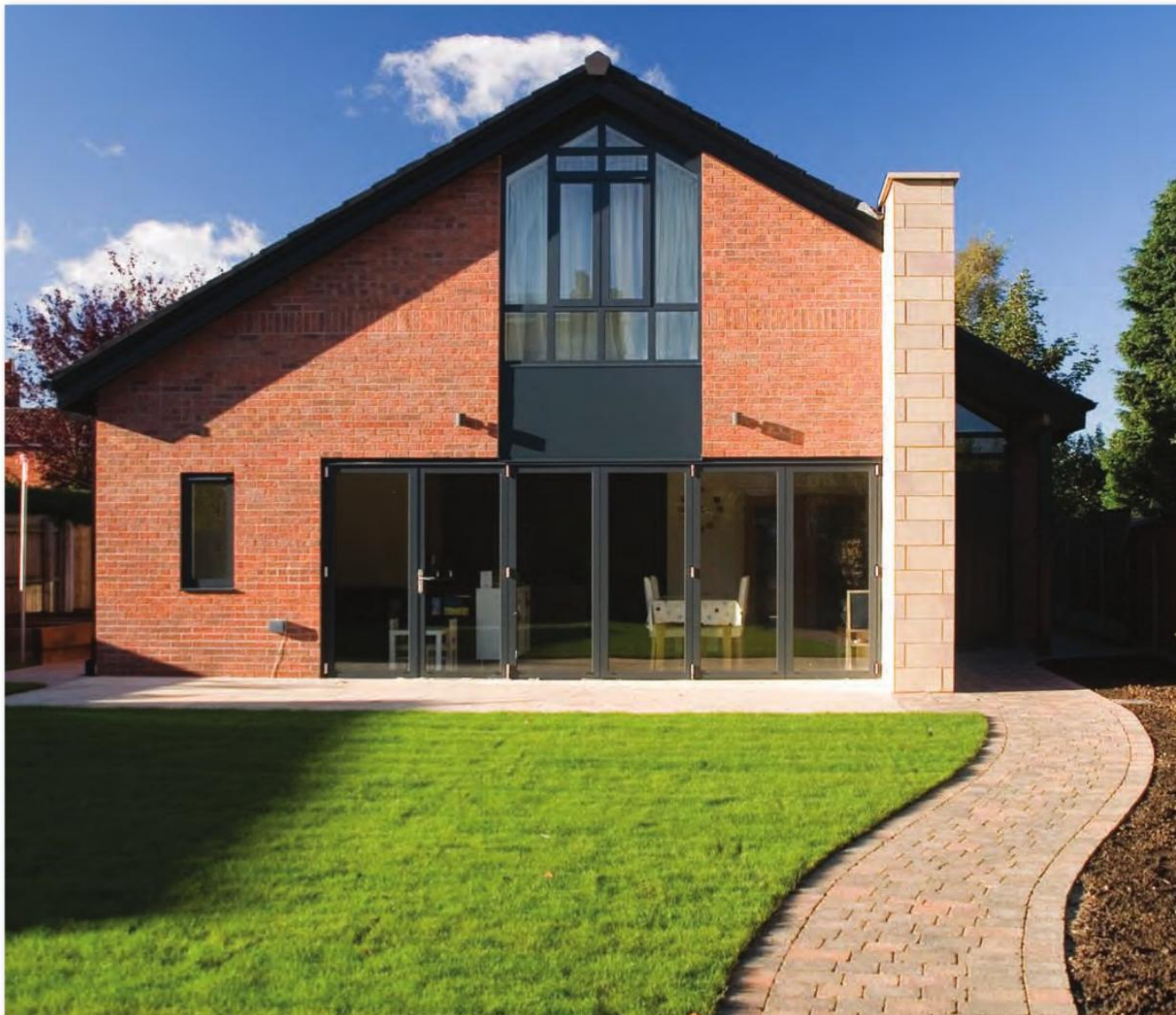
ABOVE: ARCHITECT'S HOME ACHIEVING CODE FOR SUSTAINABLE HOME LEVEL 3 RATING
