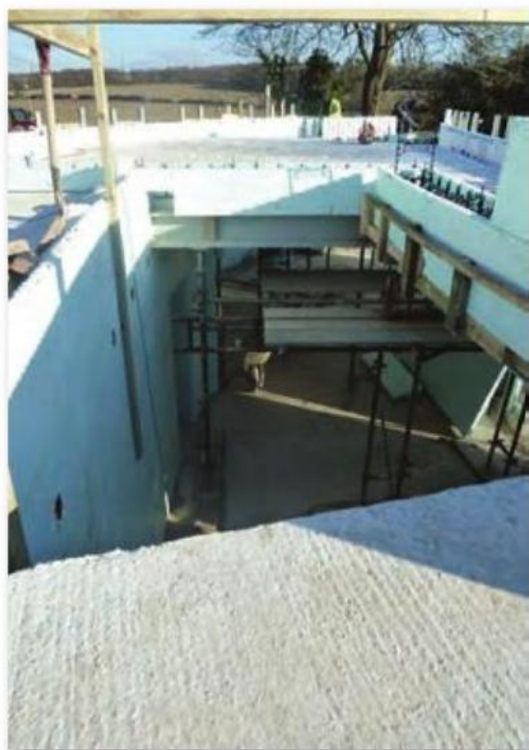
VIEW LOOKING DOWN STAIRCASE VOID INTO THE KITCHEN
