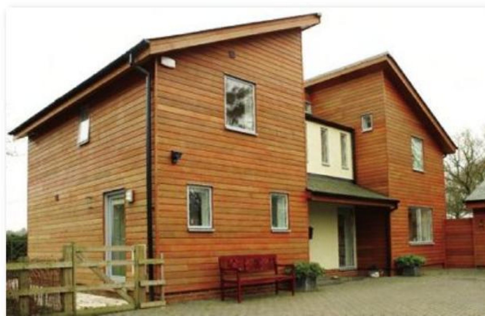
THE FRONT EXTERIOR OF THE FISHER'S CEDAR CLAD SELF BUILD PROPERTY INCLUDING A DRIVEWAY AND GARAGES BUILT BY JONATHAN. THE CLADDING IS WESTERN RED CEDAR FROM TRAVIS PERKINS
