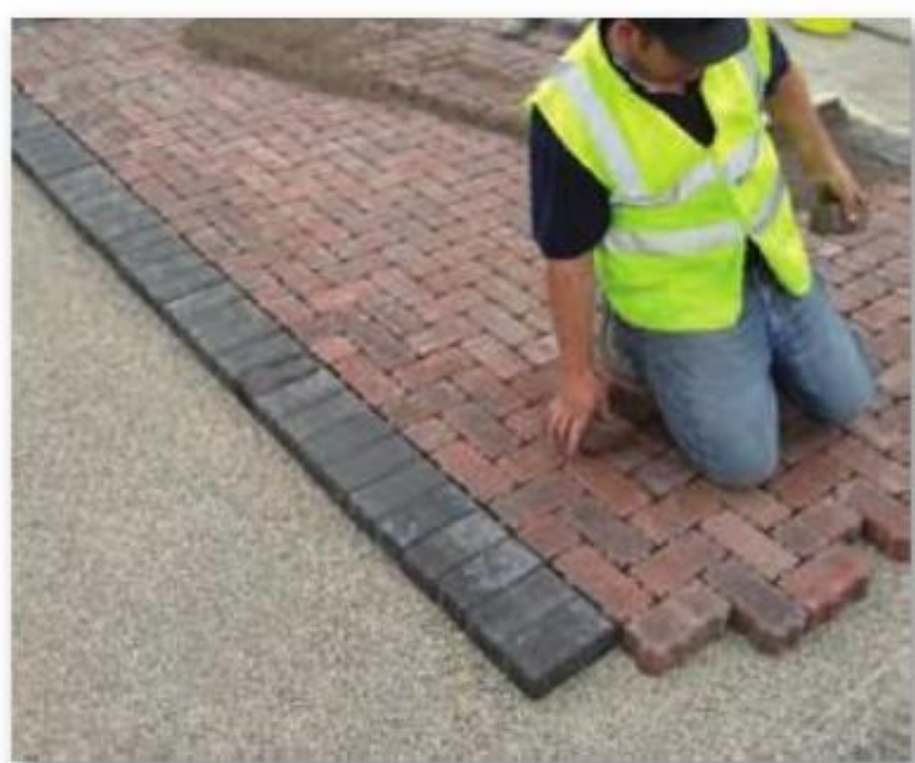
PERMEABLE BLOCK PAVING ALLOWS SURFACE WATER TO PASS THROUGH GAPS BETWEEN BLOCKS, WHILE DELIVERING A BEAUTIFUL FINISH
