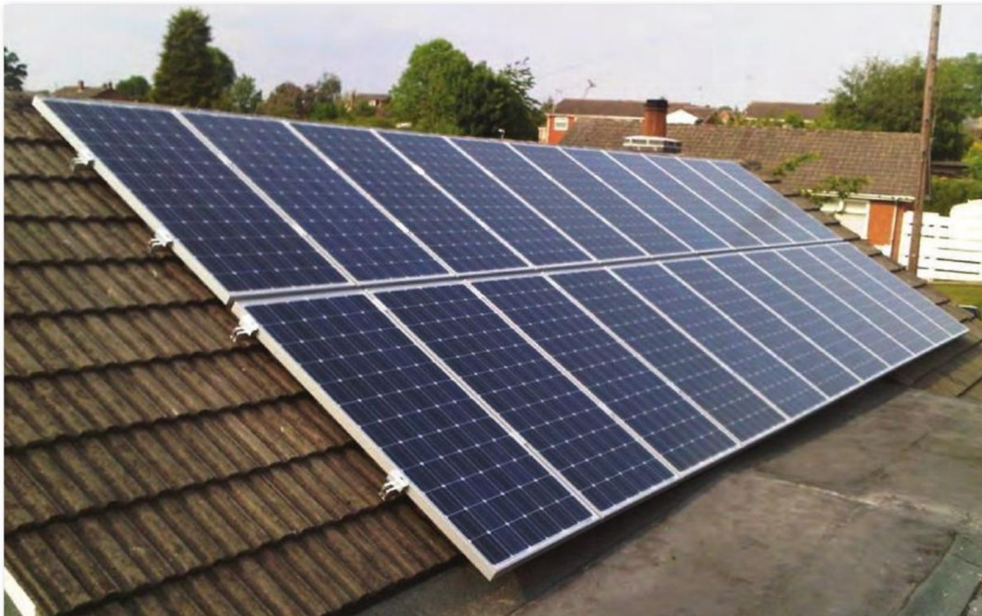
THE PANELS TO BE INSTALLED BETWEEN SOUTH EAST, SOUTH AND SOUTH WEST
