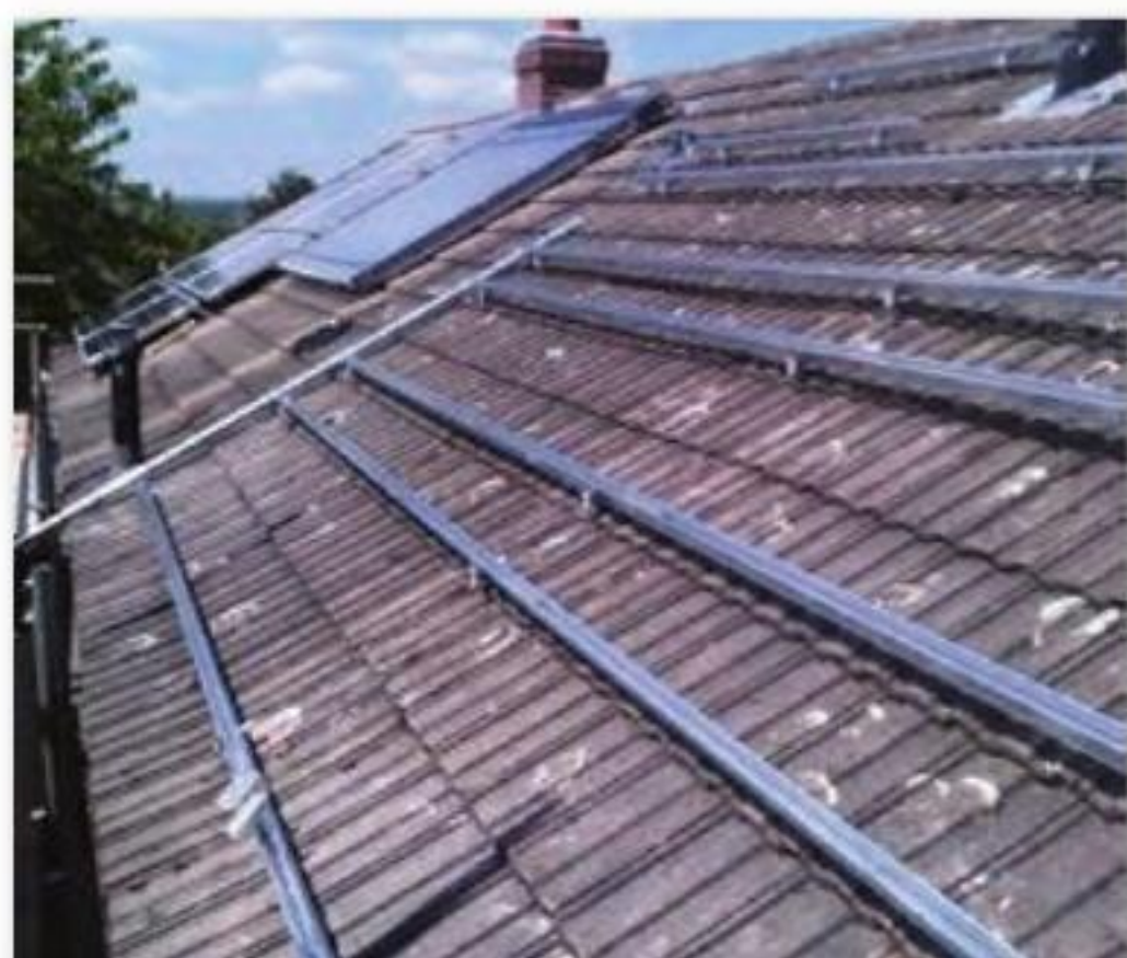
INSTALLATION OF PV PANELS
