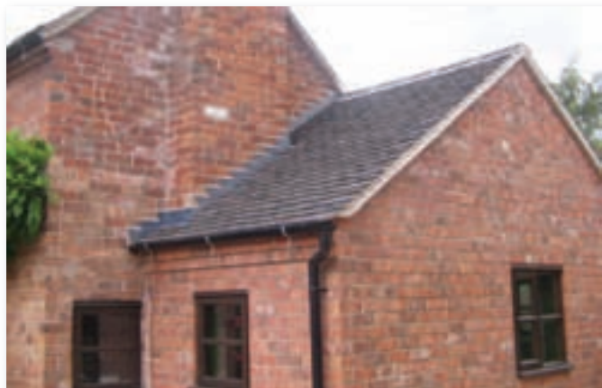
COTTAGE EXTENSION SHOWING IMITATION 'OLDE WORLD' BRICKS AGAINST ORIGINAL BRICKS
