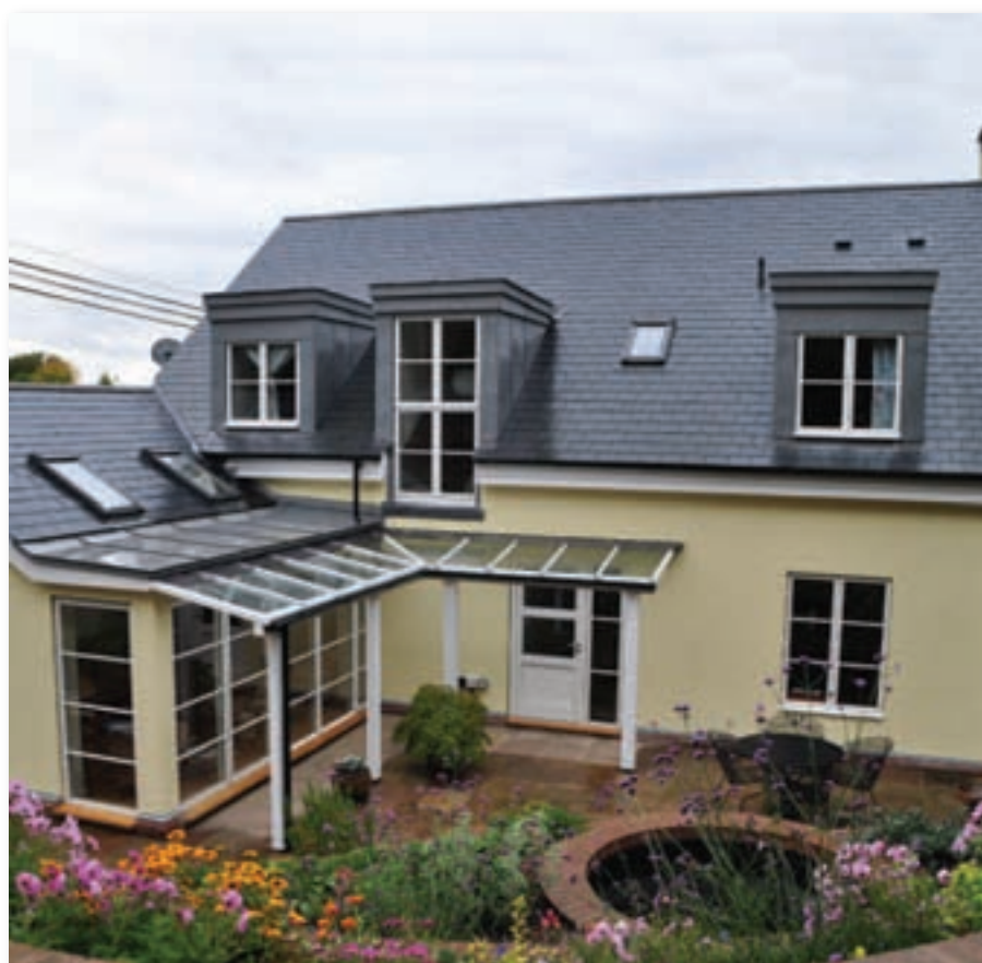
THE REAR ELEVATION OF THE PROPERTY, FROM THE TOP OF THE GARDEN, SHOWING THE CANOPIED AREA, WHICH IS AWAITING ITS GLASS ROOF
