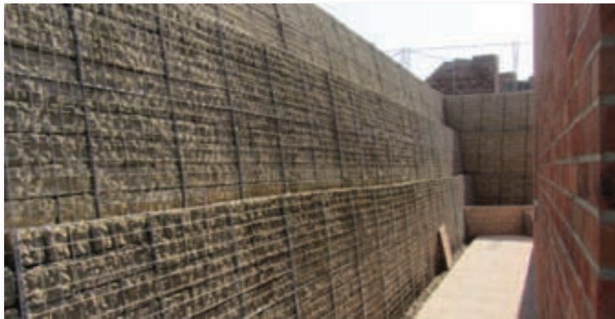
PREVIOUS: CONSTRUCTION OF GABIONS FROM LEFT: COMPLETED GABIONS ON GRAVITY RETAINING WALL; CLOSE UP VIEW
