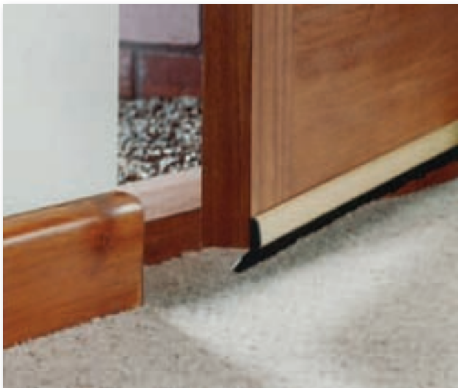
DRAUGHT PROOFING TO THE BOTTOM OF A DOOR
