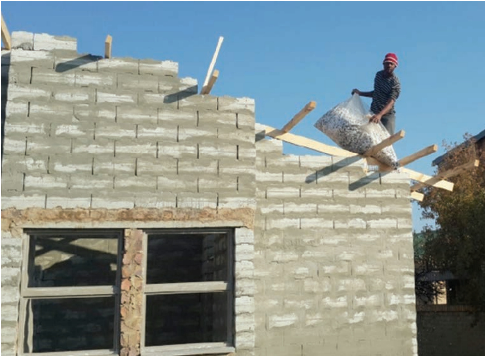
Figure 3 The polystyrene regrind is being thrown into the wall cavity for insulation.
