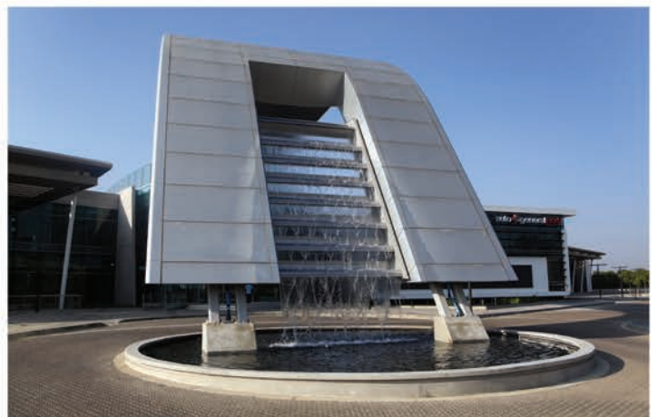
Photograph courtesy of Auto & General
