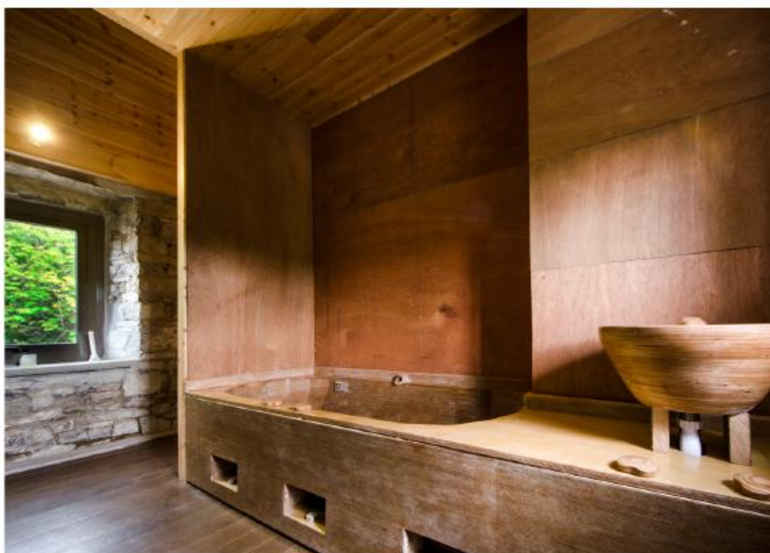
The bath and sink are made of laminated plywood.
