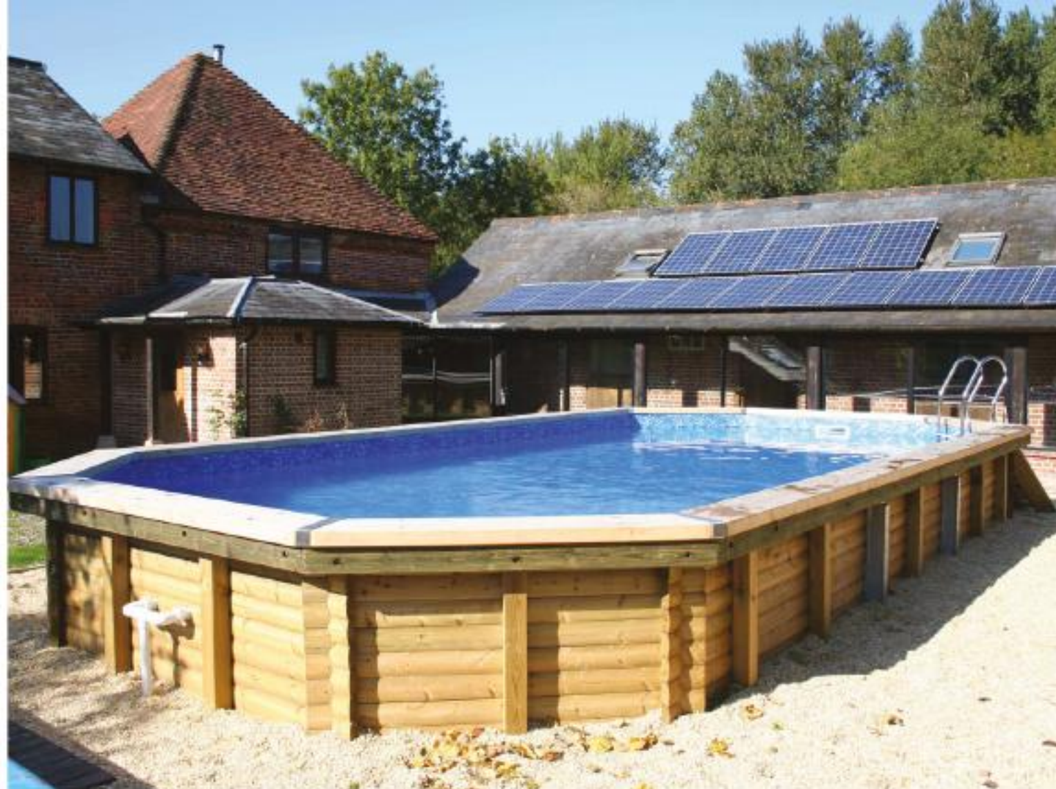
Above ground pool in area with high water table where an in-ground pool installation wasn't possible.
