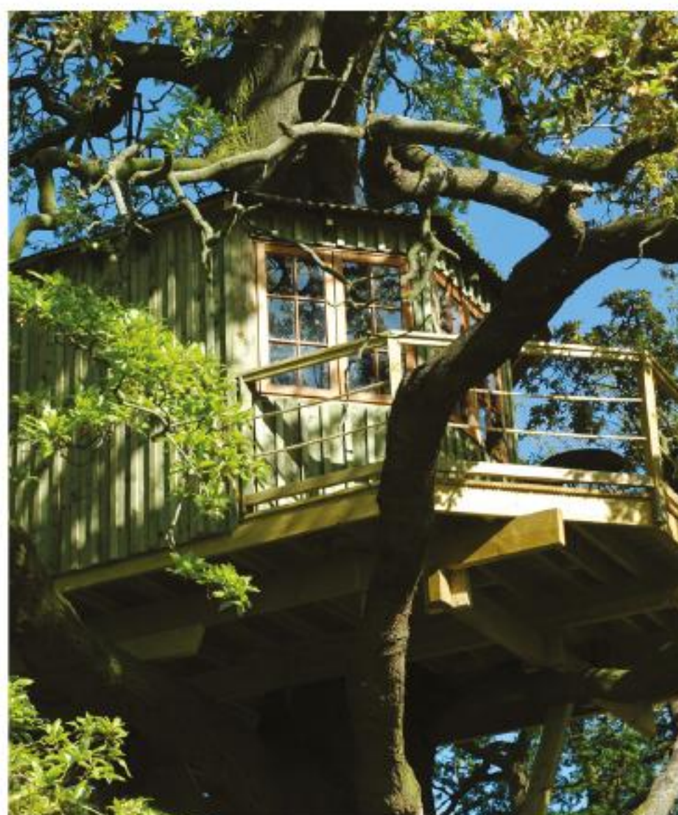
Previous page, left page and below: A one-tree treehouse construction on a mature oak tree, Co Louth
