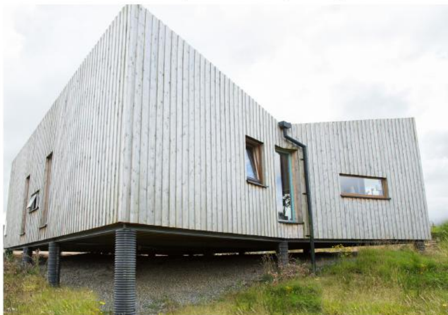
Steel reinforced concrete stilts
