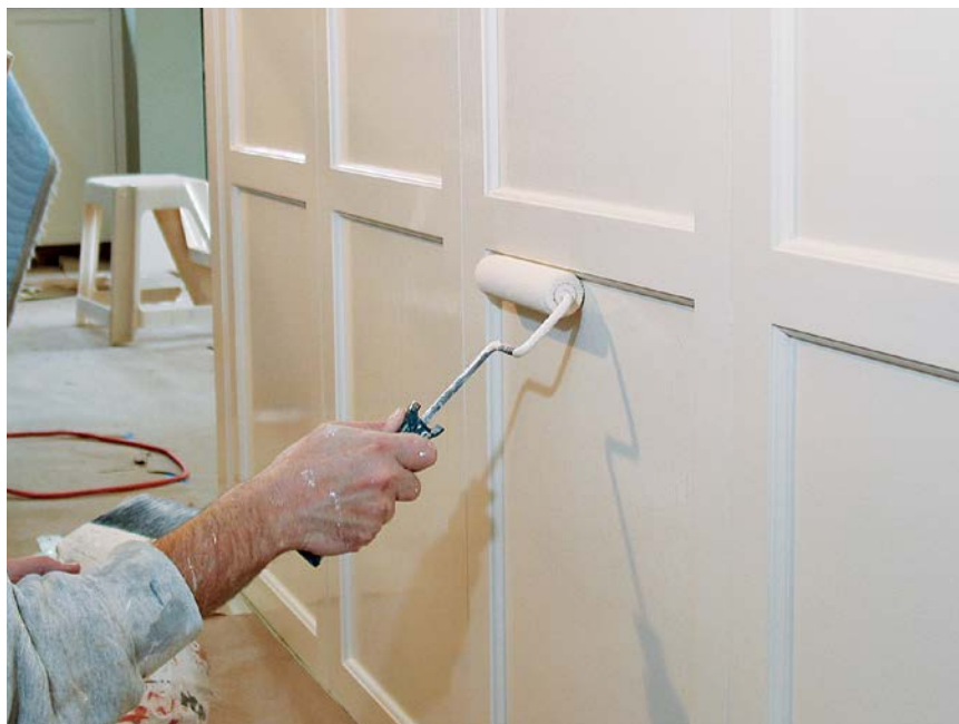
In this 1920s house, the homeowner wanted an older look for the cabinets. So after spraying three coats of oil-based enamel, the painters rehung the doors and rolled on a final coat . . .
