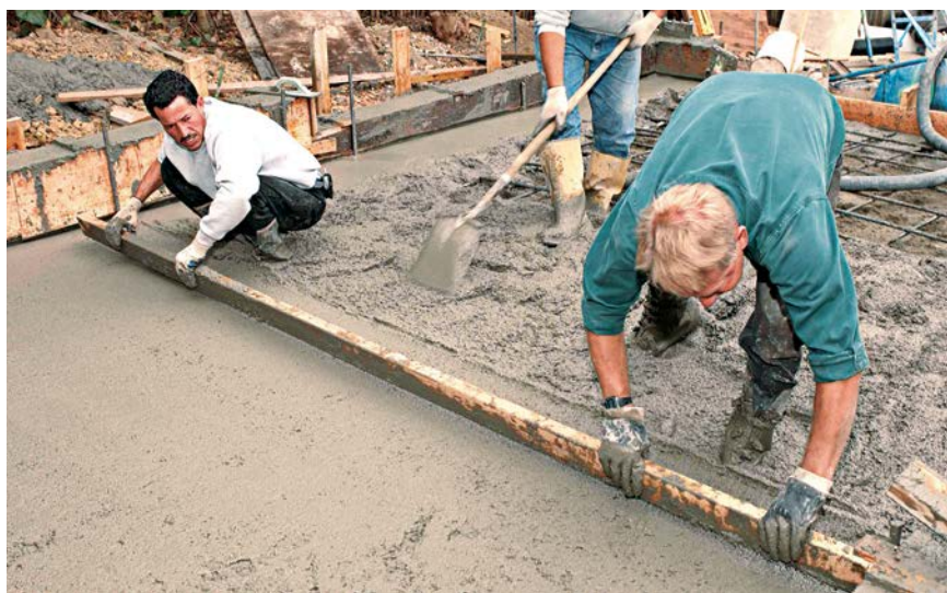
Screeding is a job for three people: two to level the concrete by moving the screed rail from side to side and a third with a shovel or rake to fill low spots and pull away excess.
