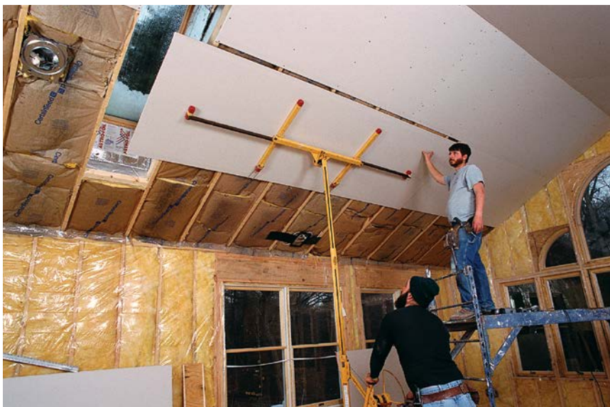
If the ceiling is higher than 9 ft., and especially if it's a cathedral ceiling, rent a drywall lift.
