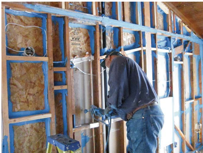
When wall surfaces are exposed, it's possible to spray an air-sealing caulk before insulating. Sprayable caulks were developed to improve the efficiency of fiberglass batts by stopping air movement within walls.
