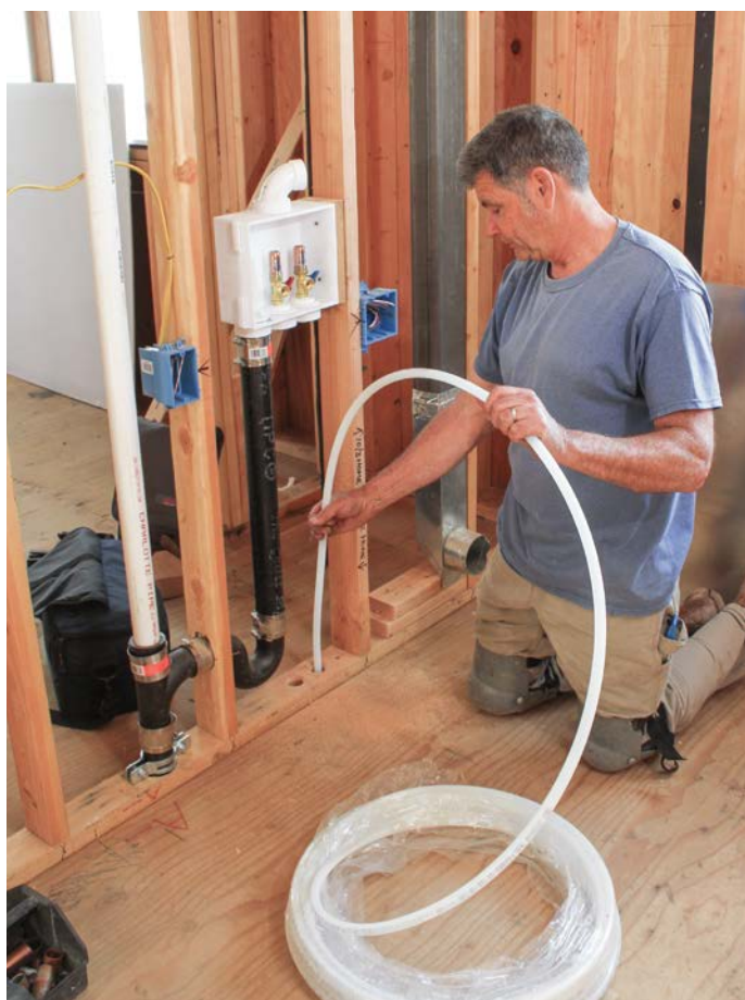
Flexible PEX tubing is fast overtaking rigid copper and PVC water-supply systems. PEX is faster, easier, and less expensive to install, particularly the soft PEX-A tubing shown, which readily uncoils so it's a snap to feed through holes and snake through walls.
