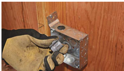
Plastic snap-in connectors snap easily into place and don't require tightening to secure cable.
