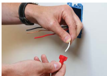
2. If the switch does not need a neutral wire, cap it and fold it into the box.
