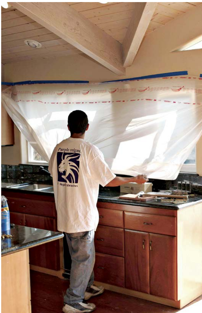
Before you start sanding floors, cover cabinets, air registers, and other fixed elements with plastic sheeting. To seal edges, use blue painter's tape to avoid lifting off paint or cabinet finishes, but remove the tape as soon as possible.
