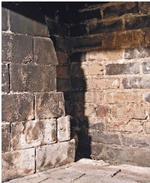
This is a partially dismantled fireplace firebox. To the left, the firebrick sidewall is solid enough to be left in place, although mortar joints need repointing. The back-wall firebricks have already been removed, revealing the back of the chimney. (An intervening wall of rubble bricks also was removed.)
