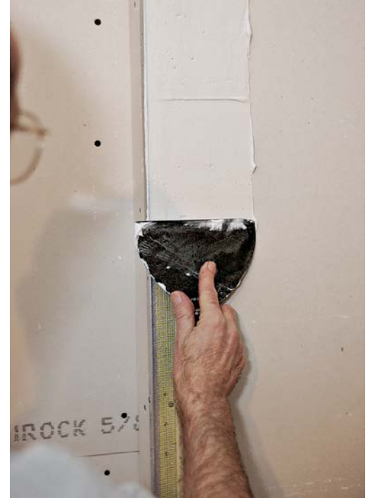
To prevent cracking along an outside corner, this installer covers the edges of the corner bead with mesh tape before applying a setting-type compound.
