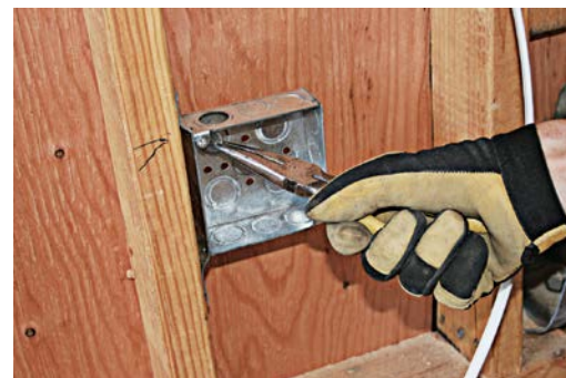
Once the knockout is loose, remove it using pliers.
