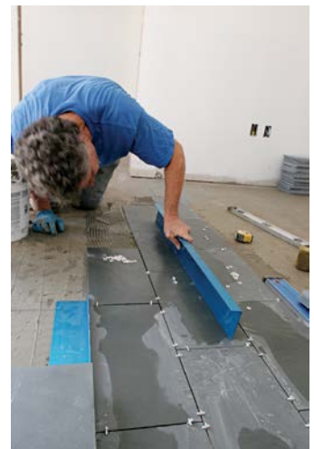
In addition to checking the alignment of tile joints to the two primary layout chalklines, use a straightedge periodically to make sure tile faces are level.
