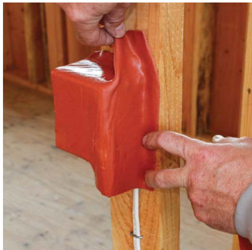
A Putty Pad shaped around an outlet box cuts sound leaks.
