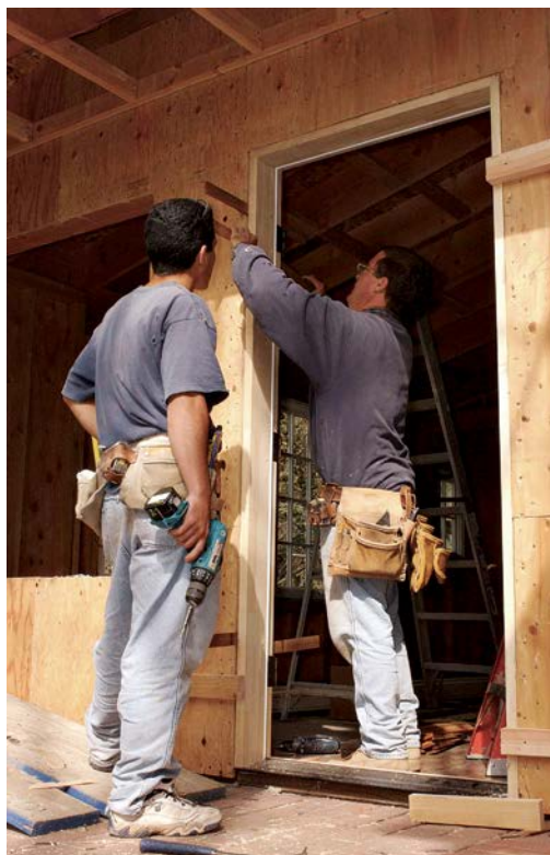
Before installing a prehung exterior inswing door, remove the door and test-fit the frame in the opening. The 2x4 cleats nailed to the sheathing act as depth gauges, so jamb edges will be flush to sheathing.
