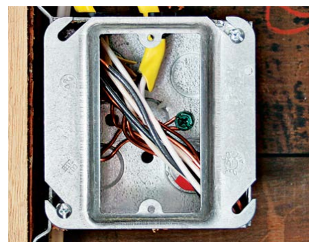
Throw a single- or double-gang mud (plaster) ring on a 4-in. box and it's hard to overfill.
