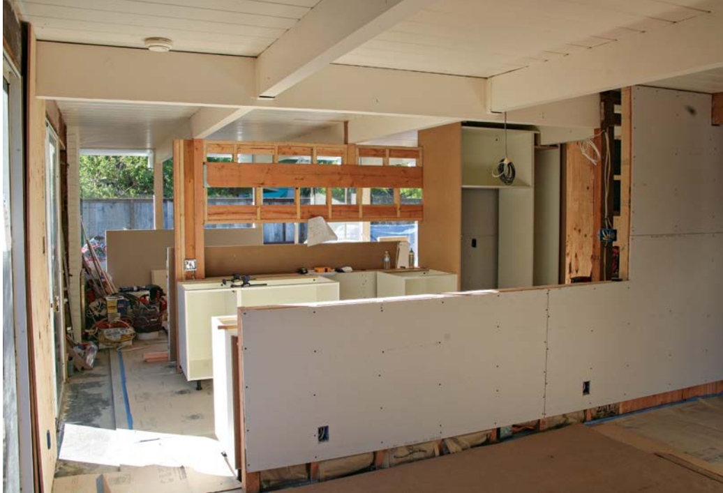
The kitchen, framed and Sheetrocked, as seen from the dining room.
