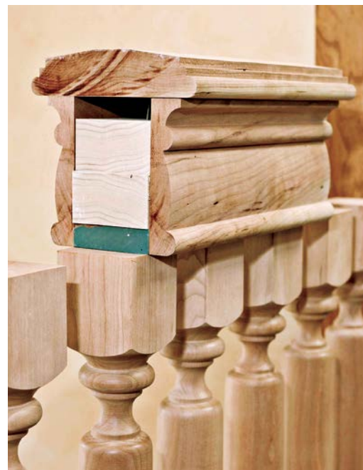
This three-piece railing assembly mockup has two skirt (side) pieces that cover the tops of the balusters and a cap. This unusual assembly will create a massive, magisterial look.
