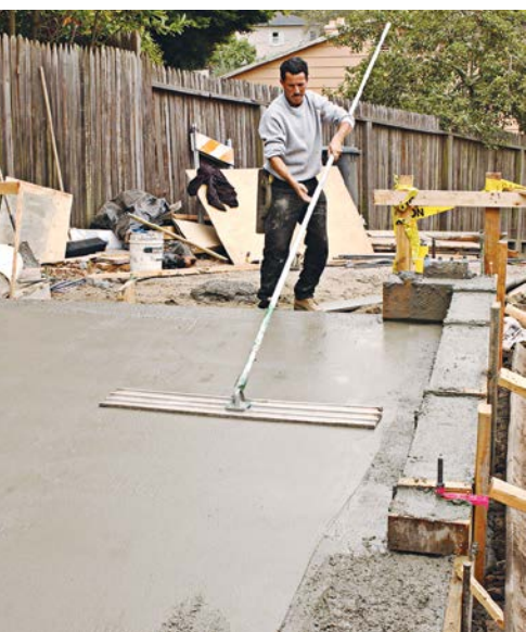
Bull-floating the concrete pushes down gravel near the surface and brings the concrete's cream to the surface.
