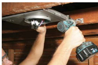
When the can height is where you want it, fasten its hanger bars to the joists.
