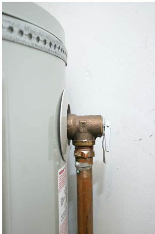
A TPR valve can prevent water-heater explosions caused by excess pressure. The discharge pipe running from the valve should end 4 in. above the floor.
