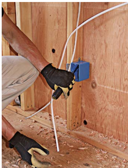
Use a screwdriver to remove a plastic-box knockout.
