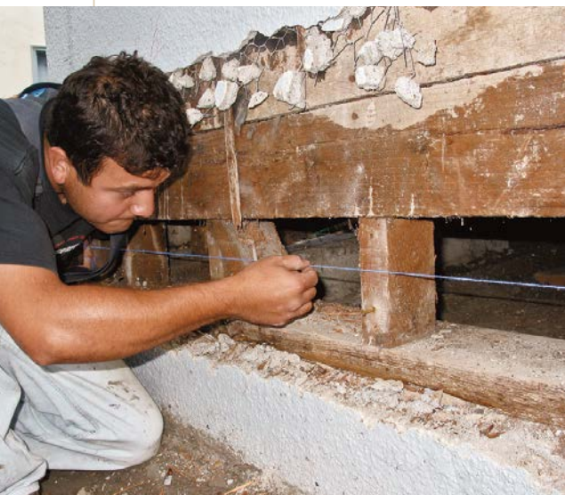
This old mudsill rotted out because the foundation was too close to the ground. After using a laser level to transfer the height of the new foundation, this builder snapped a chalkline across the pony-wall studs to indicate the height of the new sill.
