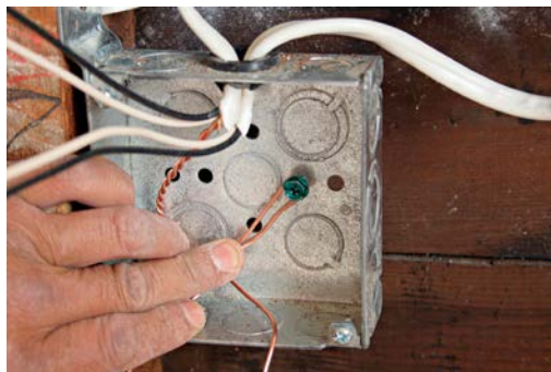
The long wire of the spliced grounds is looped beneath the grounding screw in a metal box.
