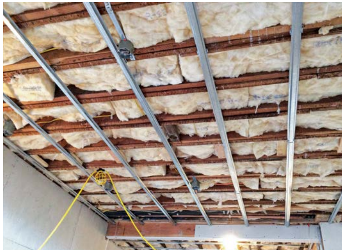
Hat channel and Putty Pads are in place as part of soundproofing this ceiling. The GenieClips are also in place, but not visible.
