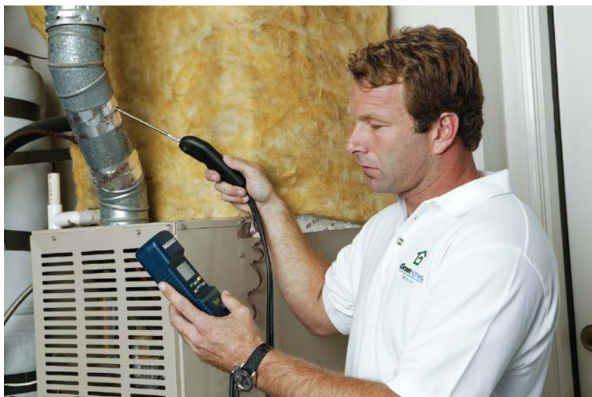
Digital combustion analyzers see how efficiently a furnace, boiler, or gas water heater is consuming fuel. An audit may also test the draft in flue pipes.
