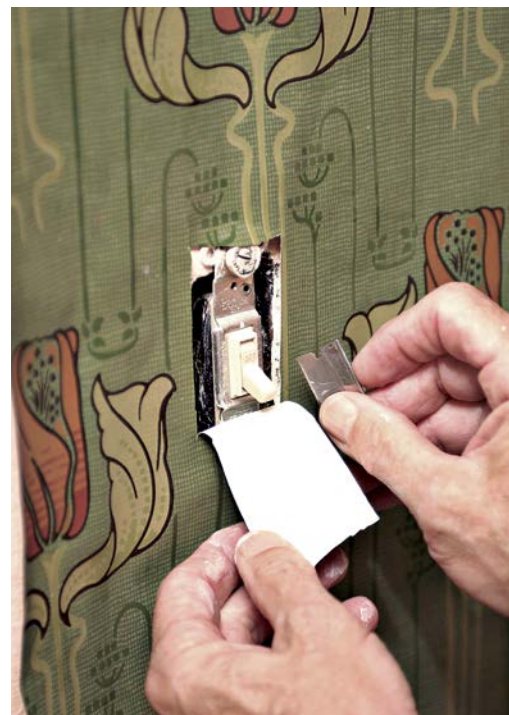
Cutting option 2: Loosely hang the paper, and cut around the outside of the outlet box. When the cutout is complete, brush the paper flat.
