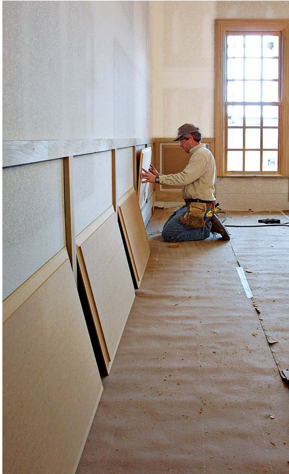
After screwing the preassembled frame to the studs, insert shaped MDF panels, nailing them directly to the wall with 2-in. brads. Leave a 1-in. gap around each panel, which you'll cover with stock molding.
