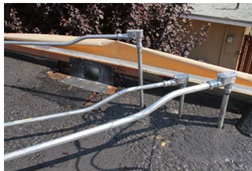
A good deal of prep work must precede the foam spraying. Here, electrical conduits running above the roof had to be raised so they would be accessible after 4 in. of foam was added.
