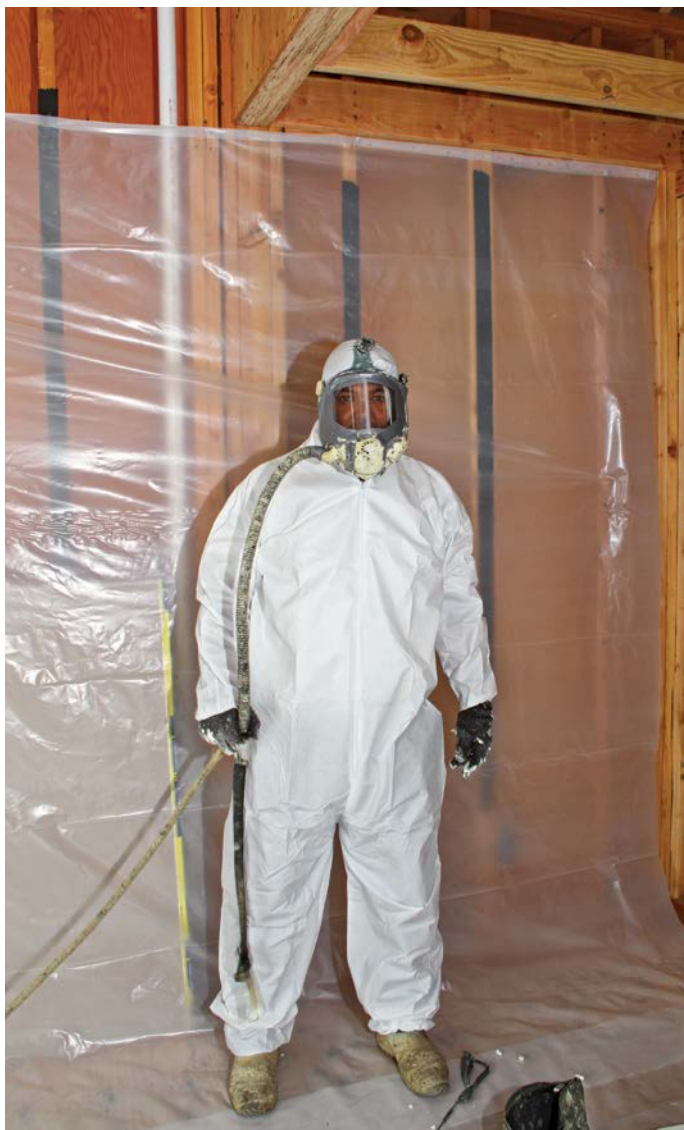
Pro gear: a Tyvek suit, gloves, and an air-fed respirator mask. Fresh air is pumped into an air-fed system, creating positive pressure in the mask so that chemical fumes cannot enter it.
