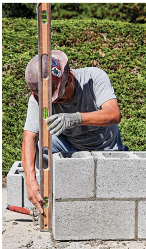
Plumb block faces with a spirit level, and use a line level (not shown) to ascertain course height.
