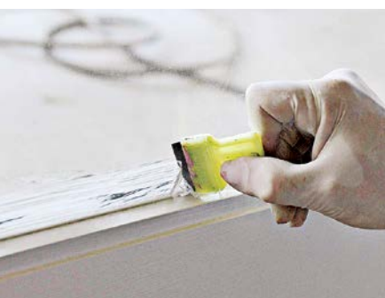
Rather than masking windowpanes or attempting to cut in clean paint lines, paint slightly ( \frac{1}{16} in.) onto the glass. After the paint dries, use a razor to cut a clean line.
