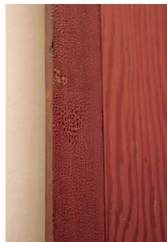
Orange peel, often seen near kitchens, is caused by airborne cooking oils.
