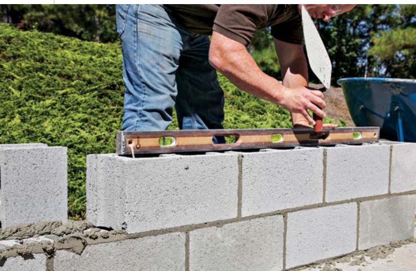
Using the handle of your trowel to tap blocks down, check for level along the length and across the width of blocks.
