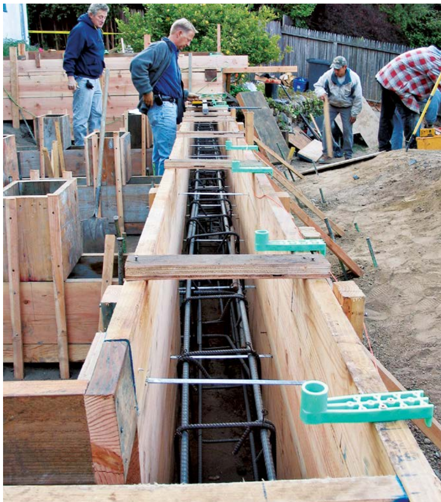
Before the pour, the rebar spine of this foundation wall is still visible. The green bolt holders will position anchor bolts 3 in. from the outside face of the foundation; as the 2x6 mudsill lines up with the outside of the foundation, the anchor bolts will be centered in the mudsill.
