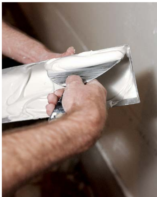
A mud pan holds enough joint compound to cover hundreds of screw holes or several long panel joints.
