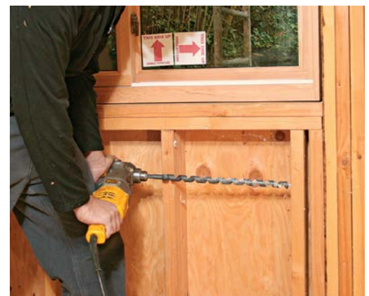
An 18-in. auger bit—also called a ship's auger—bores easily through several studs or wall plates.
