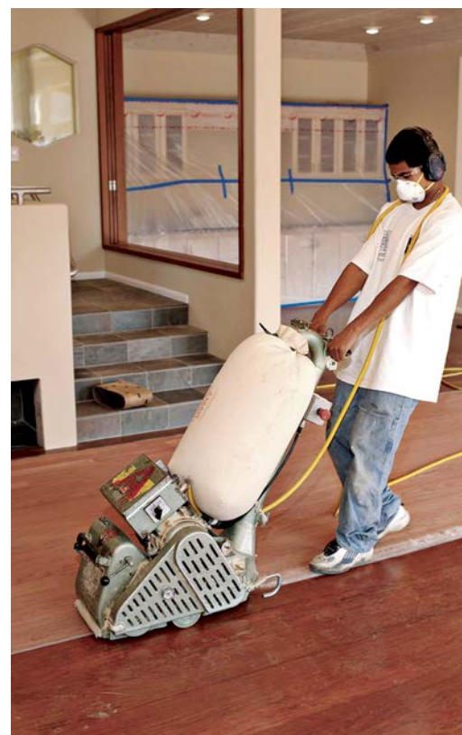
To prevent sanding over the cord, keep the excess looped over your shoulders. Drum sanders sand whether you're going forward or backing up, so as you back up, continually pull the cord away from the path of the sander.
