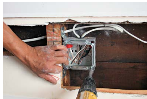
Fold the wires carefully into the box, and install a mud ring. This box is ready for a rough-in inspection.
