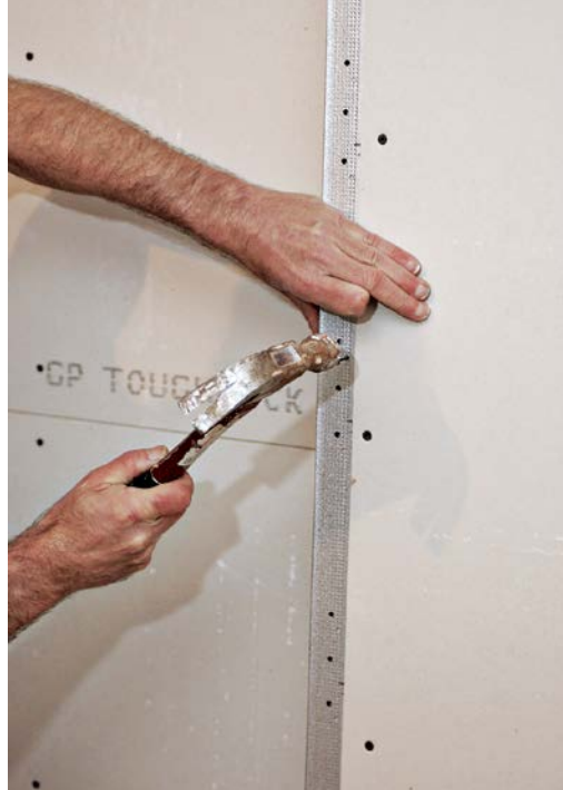
Corner bead protects fragile drywall edges and ensures a clean finished edge.
