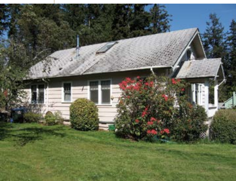
The west face of the 1928 farmhouse, before the renovation. The porch on the south face, which faces the street, had been the front door of the house when it was new.
