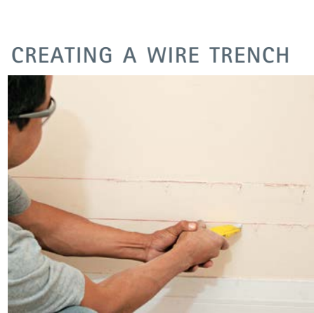
2. To ensure a clean cutline and facilitate patching when you're done, use a utility knife to score along chalklines.
