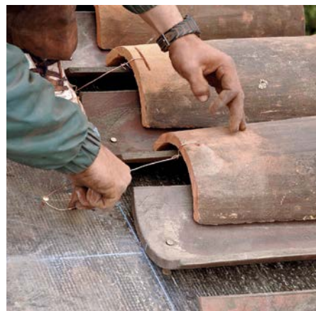
Individual mission-barrel tiles are irregular, so it's smart to snap horizontal chalklines to align tile courses and vertical lines to line up trough tiles, which are nailed directly to the roof deck. Cap tiles, which lie atop trough tiles, are secured to the roof deck with copper wire. To prevent galvanic corrosion, use nails and wires of the same material.
