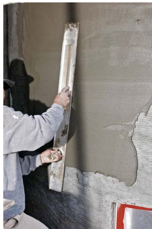
Applying the brown (second) coat takes a lot of skill. The mason starts with an irregular scratch coat and builds it up until the surface is flat and within \frac{1}{8} in. of its final thickness.
