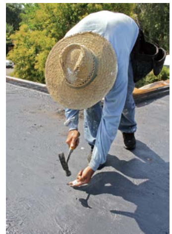
Polyurethane foam can be sprayed right over old roofing—a big selling point—but the old roof must be clean and well attached. Here, a worker installs tabbed roofing nails every 2 ft. to 3 ft. to secure the old roofing.
