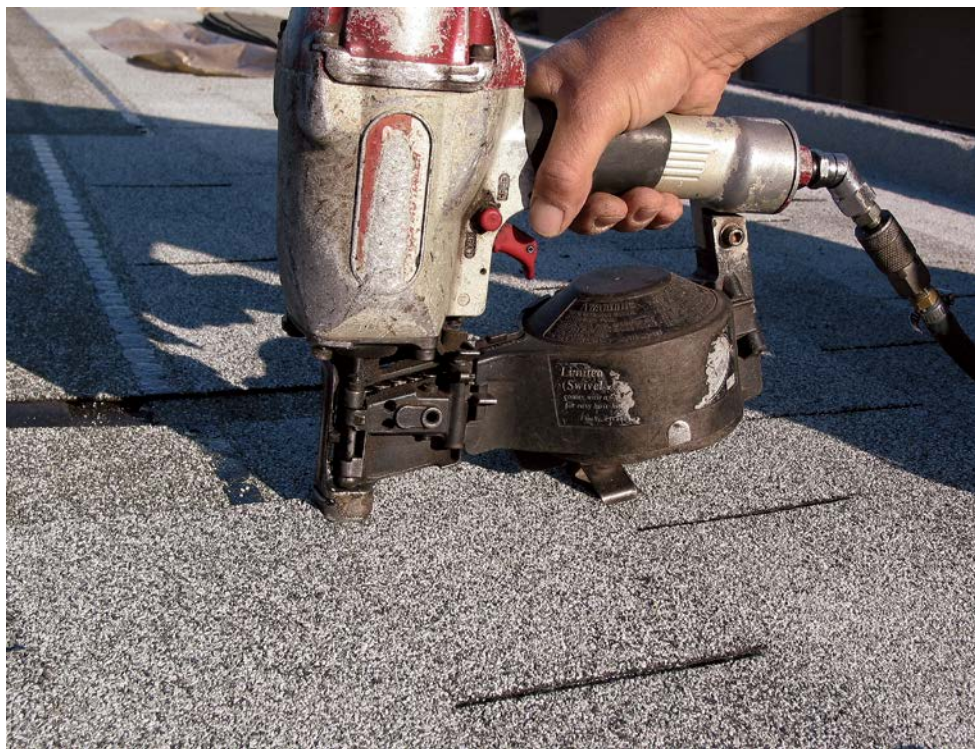
A gauge stop on the base of a pneumatic nailer can be used to set the correct shingle exposure. When the gauge stop is snug to the butt of a shingle, the next shingle above—placed against the nose of the tool—will be positioned correctly.
