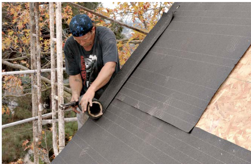
After installing drip-edge along the eaves, double the first course of shingles or, as shown, install a starter strip. The lower edge of the starter strip overhangs the drip-edge by \frac{1}{4} in. to \frac{3}{4} in.—or even 1 in. if bowing eaves or rake boards require it.
