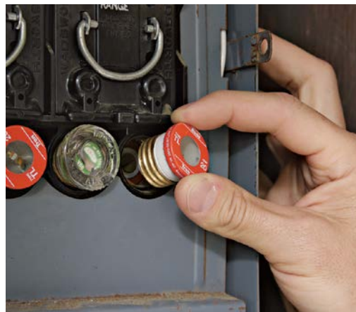
If you’re working on a fuse panel, unscrew and remove the fuse that protects the circuit you’re working on.
