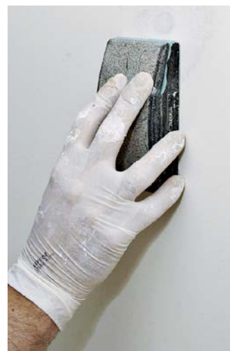
Use a sanding block or fine sandpaper to lightly sand all fills and patches before priming.
