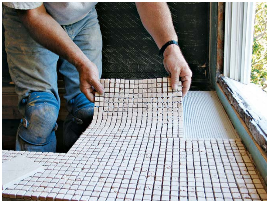
These tumbled-marble sheets are attached to a paper backing, which is embedded into the adhesive.
