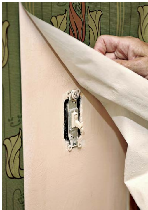
Cutting option 1: Loosely hang the paper, locate the outlet, and cut a small X over the center of the outlet, extending the X until the paper lies flat.
