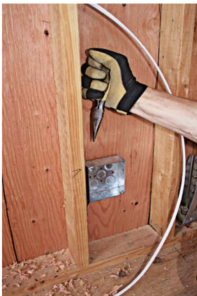
Knockouts on metal boxes require a bit more force, so jab them with a stout pair of needle-nose pliers.
