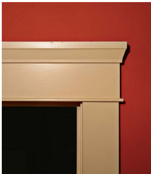
Square-cut casing needn't be plain. Here, square door casing is spiced up with a \frac{1}{4} -in.-thick beaded strip between the head and side casing and a beveled cap molding.
