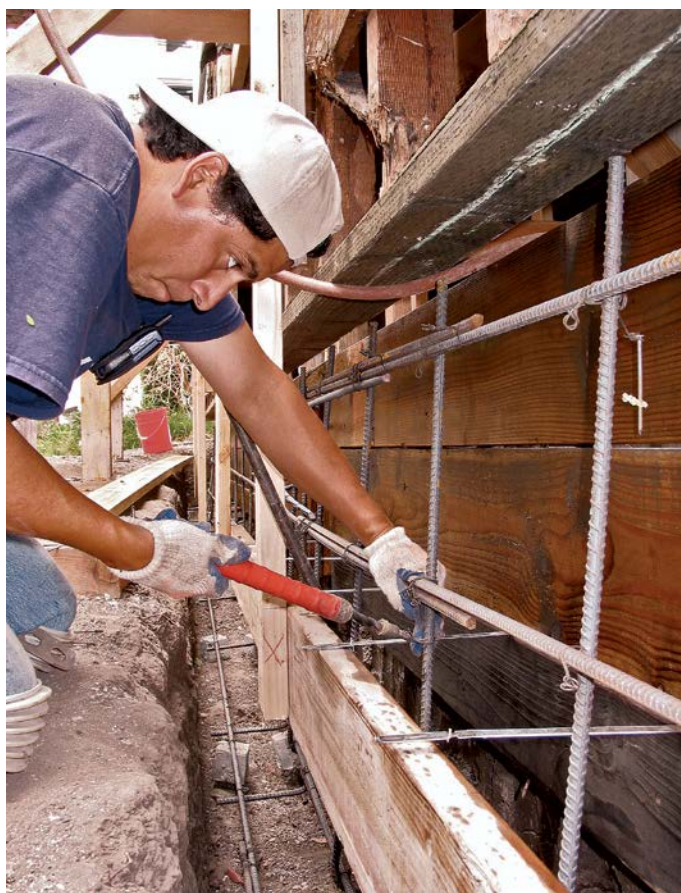
Use prelooped wire ties to splice lengths of rebar, overlapping rebar sections at least 12 in. Note the cleanly cut sides of this trench, which will serve as forms for the poured foundation footings. An electric demolition hammer with a shovel bit was used to cut this dense soil.
