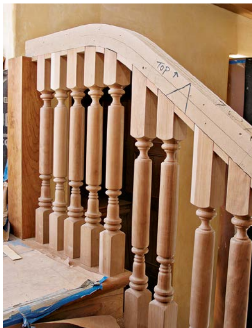
The rough cap atop this baluster section of a custom-built staircase will be covered by a three-piece railing assembly. The short fillet strips between the baluster tops can be removed should balusters need replacing later.
