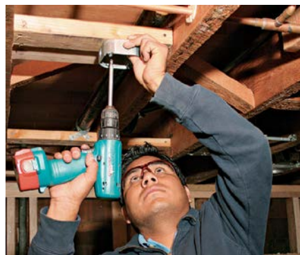
Alternately, you can nail 2x4 blocking between joists.
