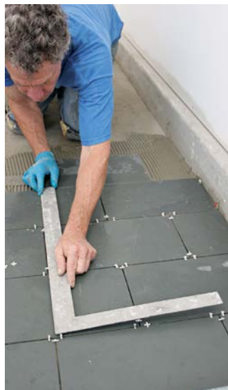
Periodically, use a framing square to check to make sure end joints line up. The white spacers between tiles ensure the correct spacing for the grout, which will be applied when the tiling is complete.
