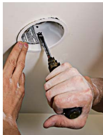
13. Use a screwdriver to push up the spring-loaded clips that pivot and press against the back face of the drywall to hold the fixture snugly in place.
