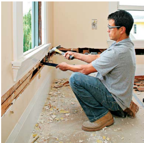
5. Use a hammer and a flat bar to pry the lath free from the studs. Work slowly to minimize damage.
