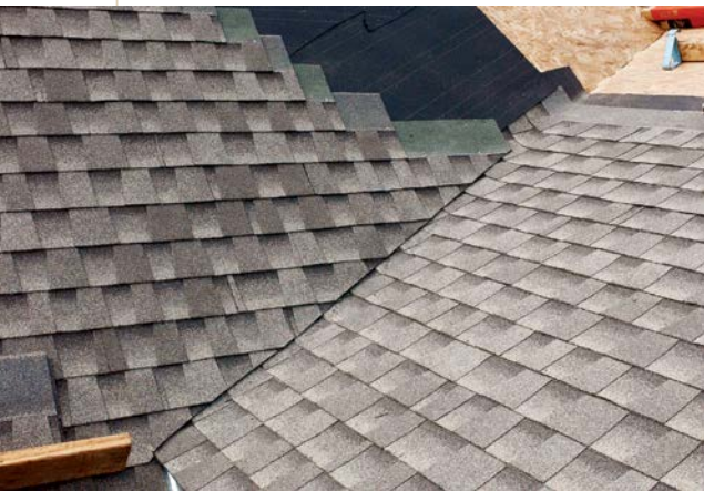
Closed-cut valleys are faster to install than woven ones because you don't need to weave shingles from two converging roof planes at the same time.
