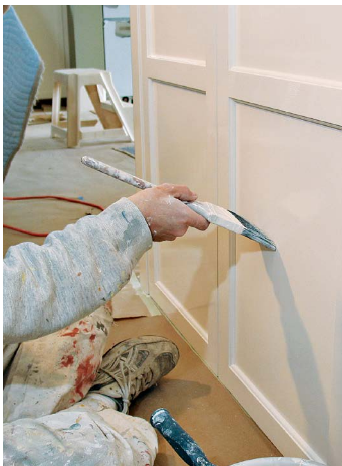
. . . which they then lightly tipped off with a dry brush, intentionally leaving very faint brushmarks.
