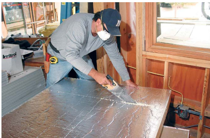
Rigid-foam insulation panels such as polyiso cut easily with a crosscut saw. To reduce the movement of air around panel edges, seal them with a compatible canned spray foam or caulk.
