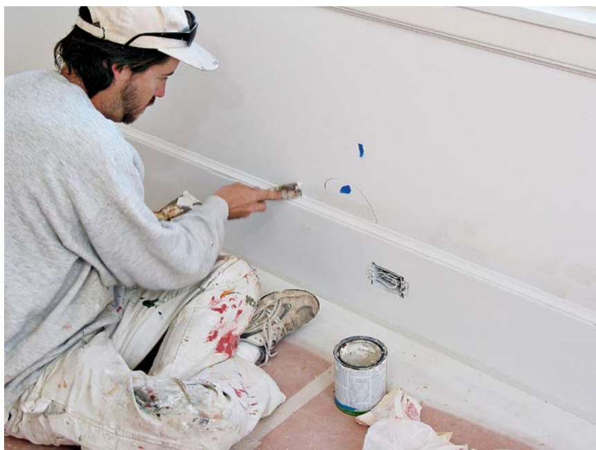
Highlight all blemishes for filling later by circling them with a pencil or attaching scraps of painter's tape near them, as shown.
