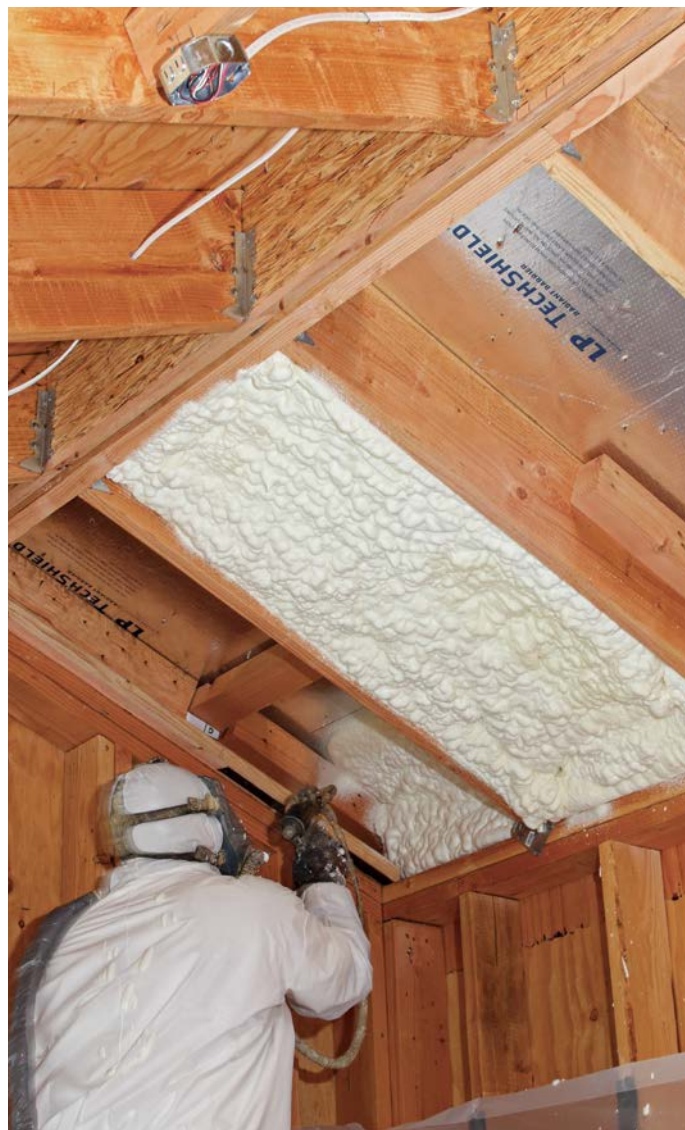
Here, rafter bays are being filled with BaySeal OCX—OC stands for “open cell” and the X denotes the fire retardant it contains. (Fire-retardant foam typically gives residents about 10 minutes to escape a burning house after the foam first outgasses a distinctive smell.)
