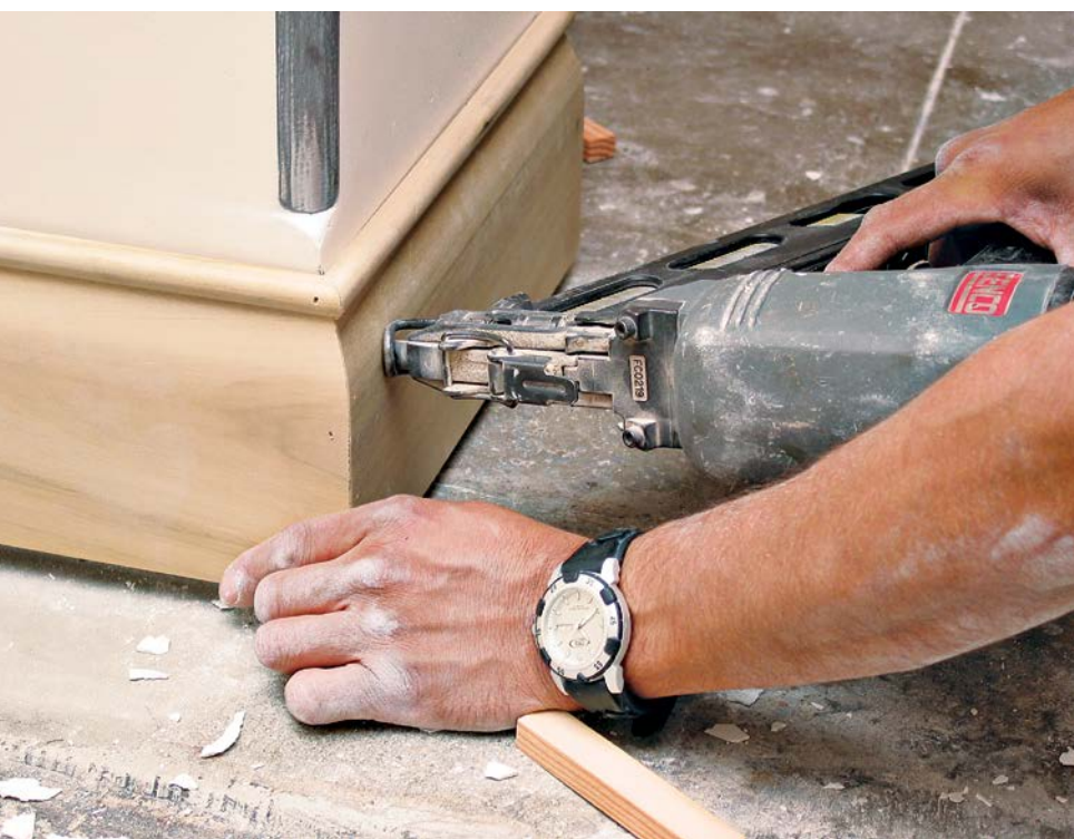
Trim covers gaps between building materials and dresses up a room. Here, baseboards are shimmed \frac{1}{2} in. above a concrete basement subfloor so engineered wood flooring or carpet can slide under it. Pneumatic nailers are much faster than hand nailing and far less likely to split or dent trim.
