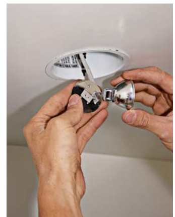
14. Insert the bulb with a gentle pressure until all pins seat. This is a low-voltage halogen bulb. Wear gloves or hold the bulb by the rim to avoid getting contaminants on the bulb.
