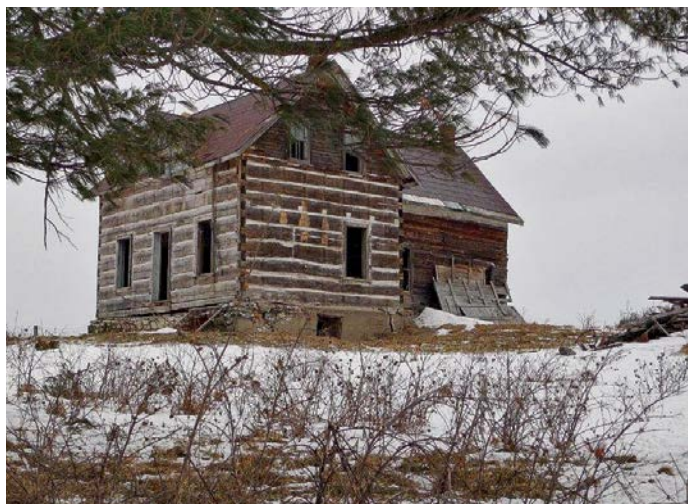
Constructed by Scandinavian immigrants around 1830, this dovetailed log house north of Ottawa was one of the few survivors of Canada's frontier era.
