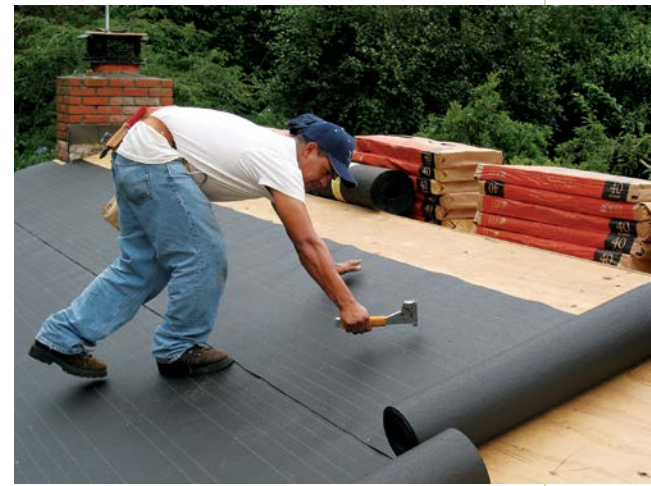
A hammer tacker allows you to staple building paper quickly so the paper won't slide down the roof as you roll it out. Later, secure the paper with tabbed roofing nails.
