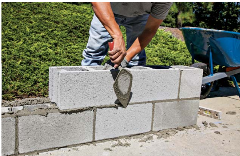
Trim excess mortar as you go, returning it to the mortar pan for reuse.
