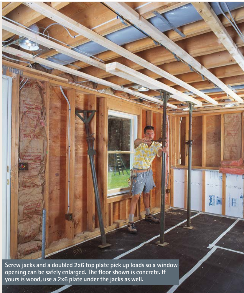
In the foreground is a 2x4 shoring with a horizontal brace.
