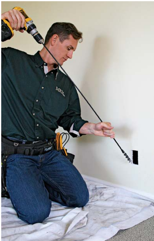
To fish cable to a new outlet, insert a flex bit into the new opening and drill down through the floor or bottom plate.
