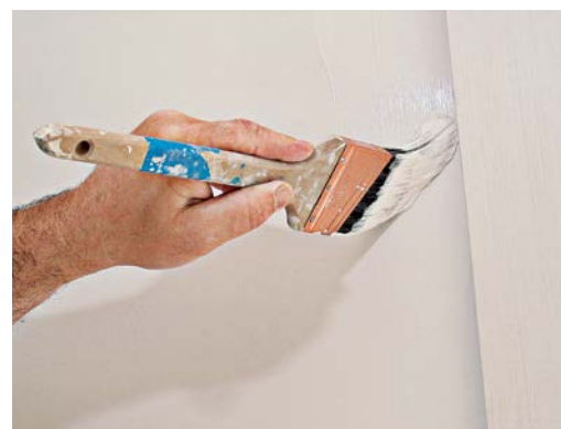
Quality bristles fan out as you apply paint. Here, the tapered bristles of a 2½-in. angled sash brush cut a straight edge where walls meet trim.
