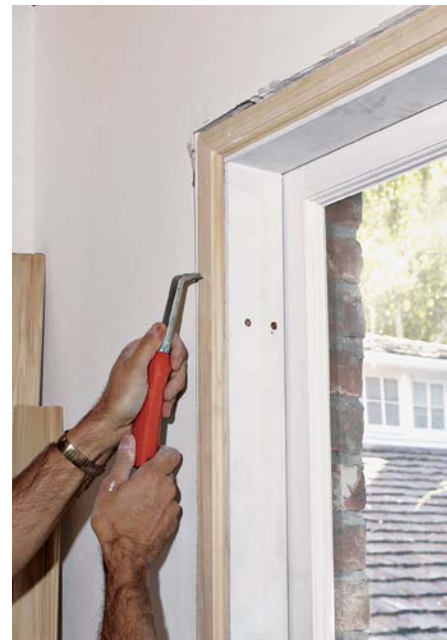
Use a scraper with replaceable carbide blades to shave drywall high spots and hardened joint compound. Use a utility knife to cut back shims still protruding around frames.
