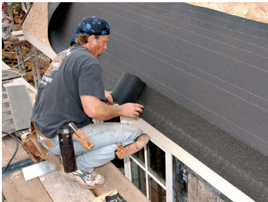
After installing drip-edge along the eaves, double the first course of shingles or, as shown, install a starter strip. The lower edge of the starter strip overhangs the drip-edge by \frac{1}{4} in. to \frac{3}{4} in.—or even 1 in. if bowing eaves or rake boards require it.
