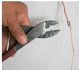
A crimp tool may be used instead of a wire nut to splice ground wires.
