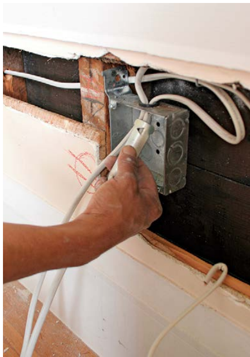
A cable ripper slits sheathing without damaging individual wire insulation. Use diagonal cutters to cut free sheathing.
