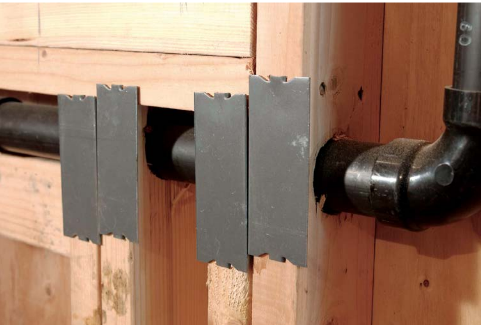
Made of 16-gauge steel, nail plates protect plumbing pipes and electrical wires from being punctured by nails.
