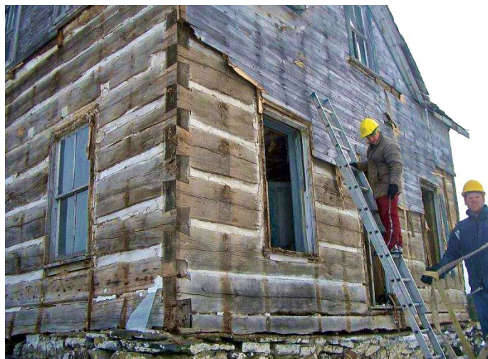
Workers remove siding before disassembling the log structure. Installed about 20 years after the house was built, the siding protected the logs from the harsh climate.
