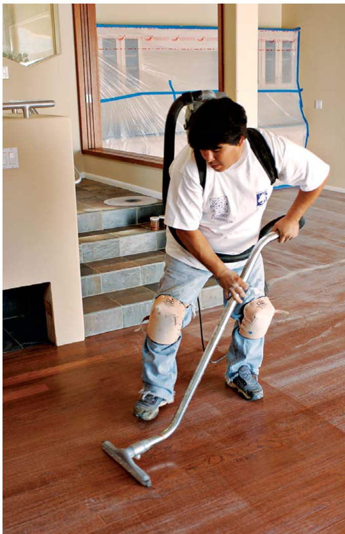
Backpack vacuums are less likely to gouge flooring or bash woodwork, but their capacity is generally less than that of floor models. Empty vacuums when they're one-third full because the fuller they get, the less efficient they become.
