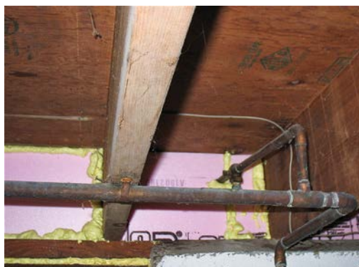
Rim joists lose a lot of heat in cold climates. Here, a Connecticut homeowner cut and fitted XPS foam panels into joist bays and sealed edges with expanding foam. Seal any penetrations in basement walls.
