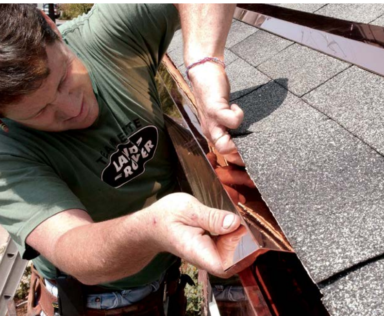
Drip-edge flashing allows water to drip free from roof edges. Here, copper drip-edge is being retrofitted under an existing roof before being fastened with 3d copper flashing nails. An uninstalled piece is shown lying atop the shingles.
