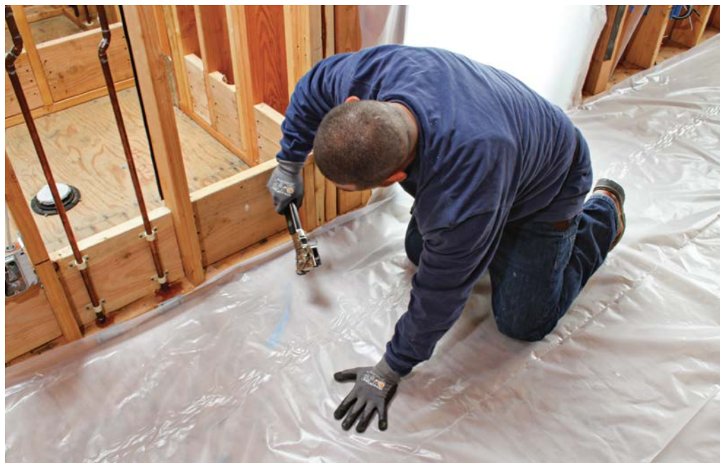
To prevent foam from sticking where it wasn't wanted, the crew stapled sheet plastic over windows, doors, plywood subfloors, finish surfaces, and stud walls to a height of 8 ft.
