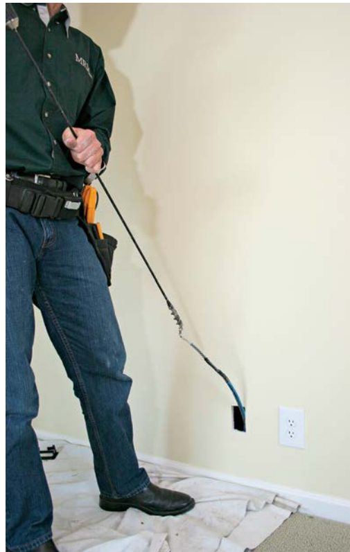
Pull back after a helper below the floor attaches the cable.
