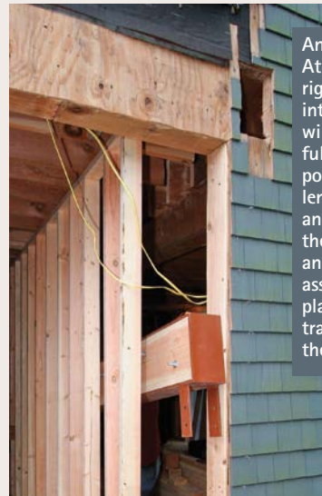
The subfloor in place, with an I-beam waiting to be hoisted. Note that a slot has been cut into the 2x12 ceiling-joist array above, into which the W12x26 I-beam will fit. At this transitional point, the girder and post seen in the photo above right are now carrying roughly half the load—the joists at left—and shoring, at right, supports the cut-through joists. Once the I-beam is in place, the severed joist ends will hang from the 2x12s bolted to both sides of the I-beam. Peeking up from under the I-beam is cribbing on which the shoring sole plate rests.
