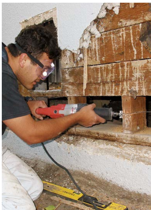
Once the needle beams are in place to pick up the loads that were previously carried by the pony wall, you can cut the pony-wall studs and remove the sill.
