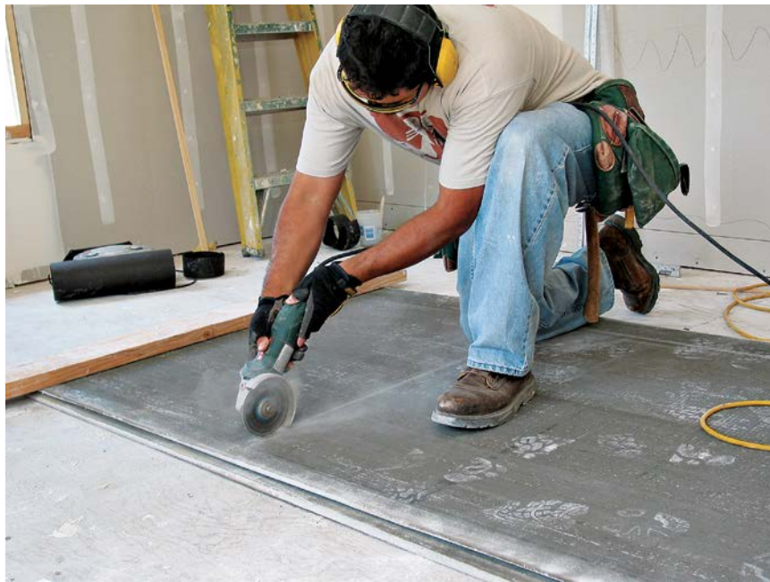
A handheld grinder with a diamond blade makes a faster, more reliable cut in backer board than a utility knife, but it also produces more dust.
