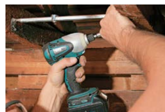
For box placement midway between joists, use an adjustable bar hanger.
