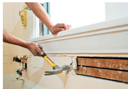
4. If walls are drywall, simply pull out the isolated strips. If plaster, use a hammer to break out the plaster and expose the lath.
