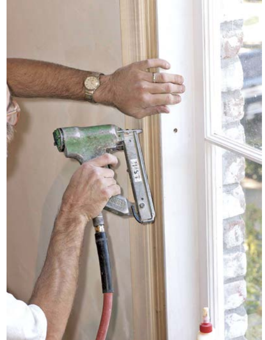
When it comes to finish nails and nailers, smaller is often better. This pin nailer weighs less than 5 lb. and shoots 1-in. to 1½-in. nails.
