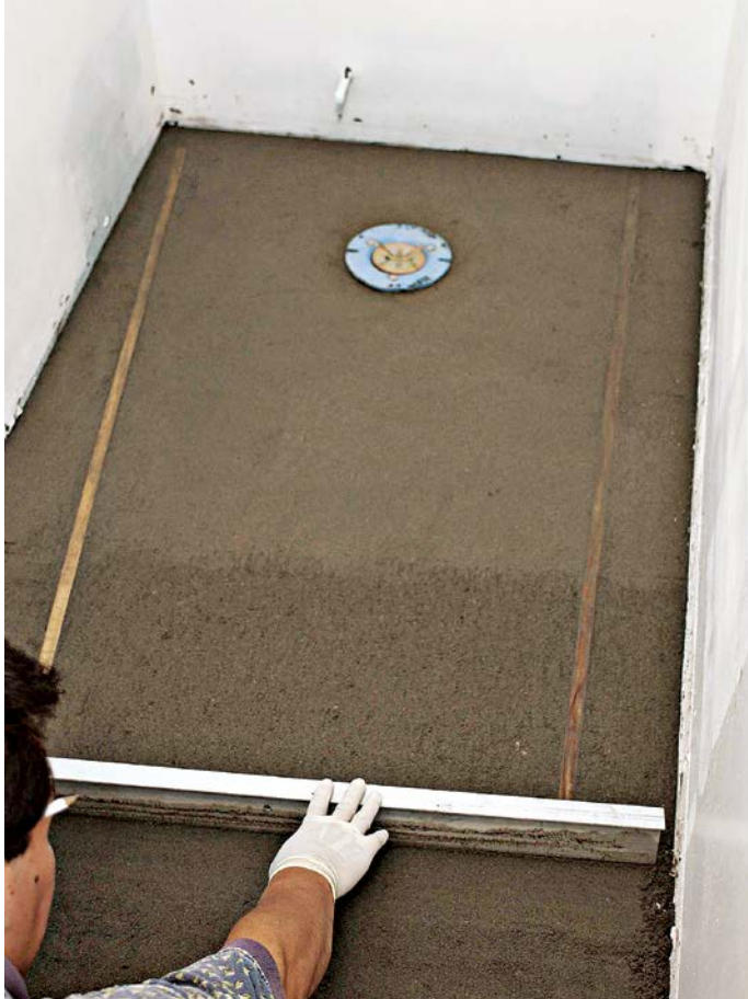
Create a level mortar bed by drawing a metal screed board across two float strips pressed into mortar columns. After the mortar has been screeded, the wood float strips are removed and their voids filled with mortar.
