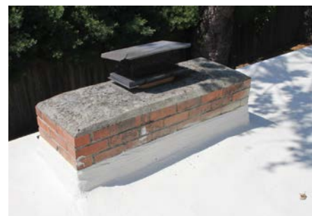
Spray foam adheres aggressively, so it’s important to mask everything you don’t want foamed. Here, polyurethane foam is being applied to the chimney. In the background is the masked-off parapet.
