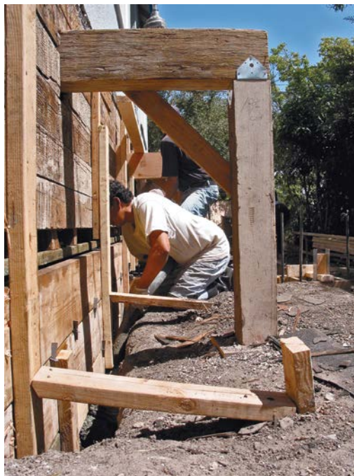
Ready for concrete—the form walls are up and braced. Metal wedges inserted into the ends of the form ties will keep the formboards from spreading. The next step is to pour the footings before pouring the foundation walls.
