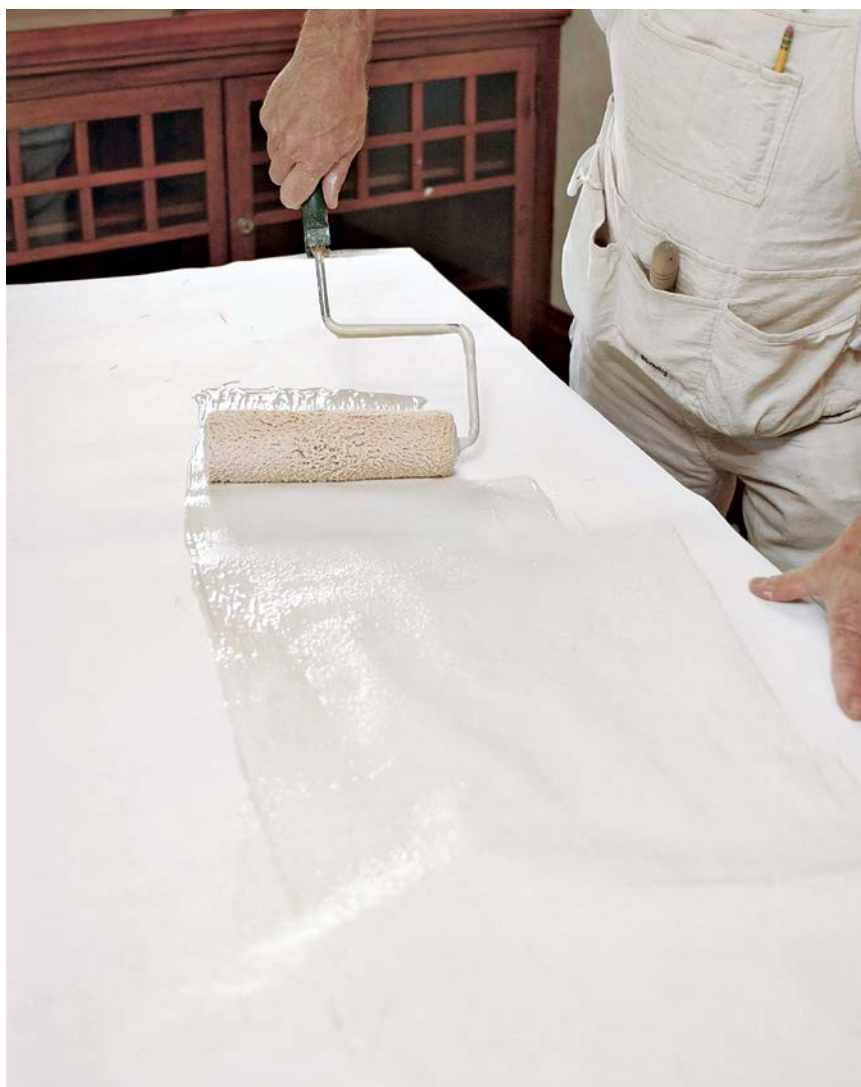
As you apply paste, roll it out from the center toward the edges. Hold down the wallcovering with one hand to keep it from sliding as you roll.
