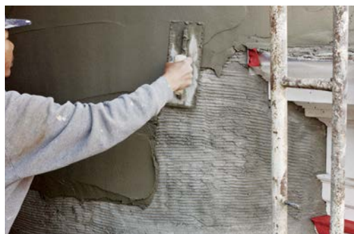
Applying the brown (second) coat takes a lot of skill. The mason starts with an irregular scratch coat and builds it up until the surface is flat and within \frac{1}{8} in. of its final thickness.
