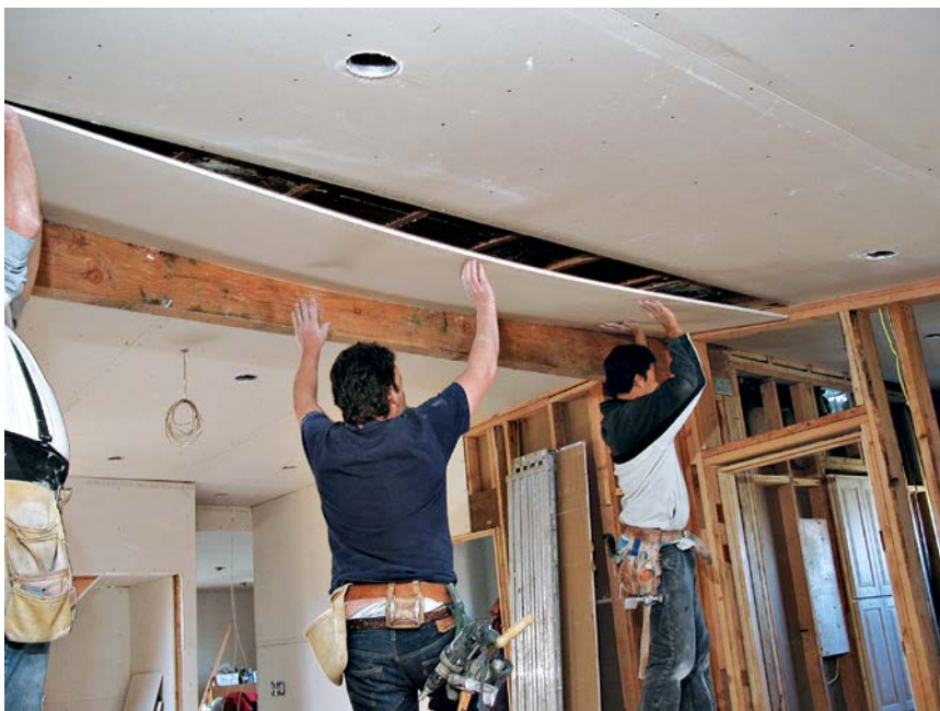
With a helper and a set of drywall benches, you can safely raise long panels to the ceiling. Lift one end at a time. Whenever possible, run the panels perpendicular to the joists.
