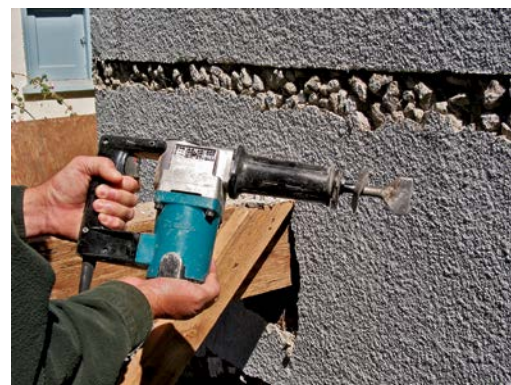
Used correctly, an electric chipping hammer fractures stucco without destroying the underlying wire mesh and waterproofing membrane.
