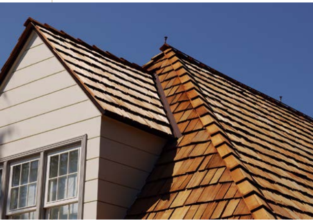
This classic wood shingle roof has an open valley. Shingle caps cover the roof hip.
