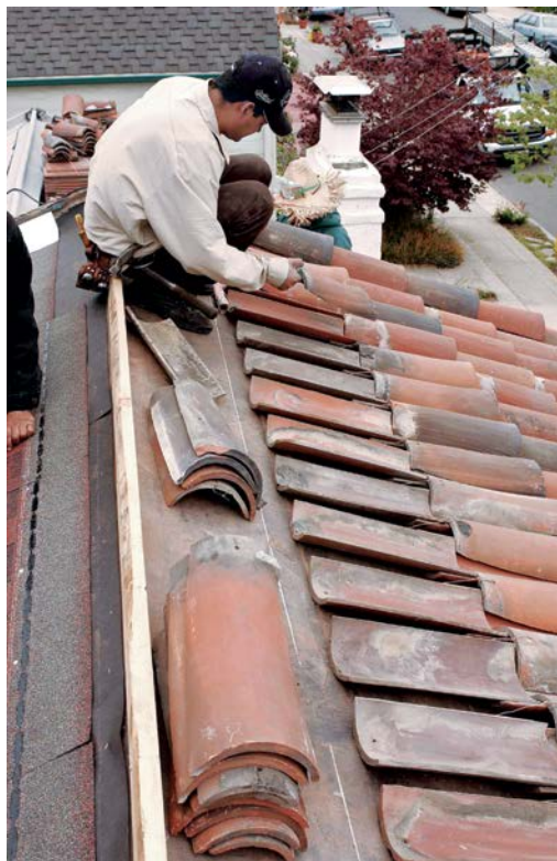
If properly installed over a durable membrane—such as the fiberglass-reinforced underlayment shown here—a tile roof can last 80 years.
