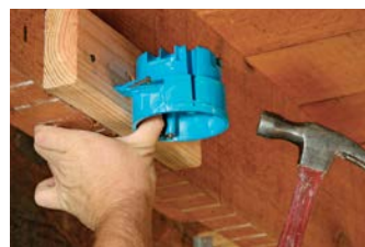
Use blocking to get the box in just the right spot.
