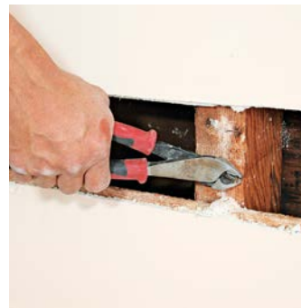
6. Pull out any nails still stuck in the studs; this will make later repairs easier.
