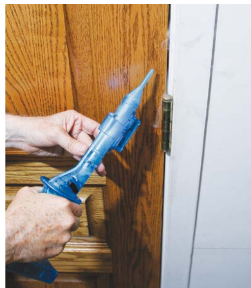
A smoke pencil helps make air leaks visible.
