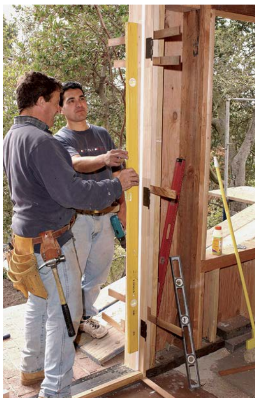
Shim and secure the hinge jamb first, checking for plumb often. Here, installers place shims slightly above and below the hinges so the hinge screws sticking through the jamb won't snag on the shims.
