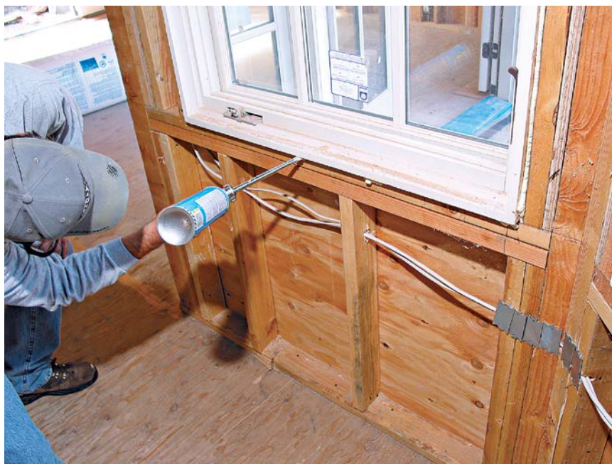
To fill gaps around window and door frames, use a mild-expanding polyurethane foam; more expansive foams can bow frames and cause a window or door to bind in the frame.
