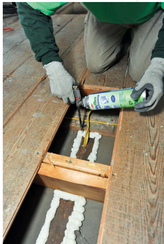
Air-sealing is a crucial first step before insulating. Here, polyurethane foam is used in the attic floor to seal gaps along the top plate of a partition. Penetrations for plumbing pipes and electrical cables may be small but they can add up to big heat loss.
