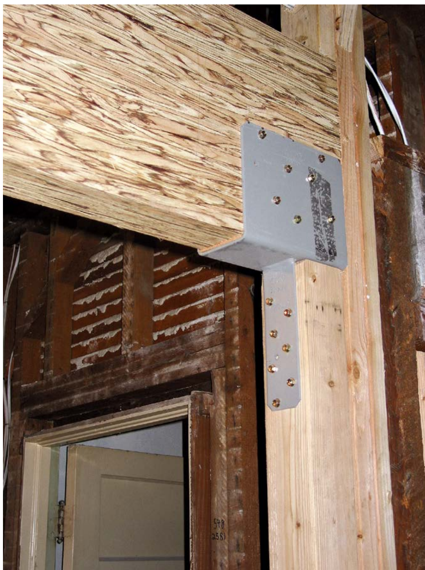
This engineered beam is a 4-in. by 14-in. Parallam girder secured with a Simpson CCQ column cap.
