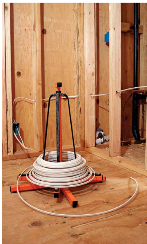
A wire reel prevents kinks in cable as you pull it.
