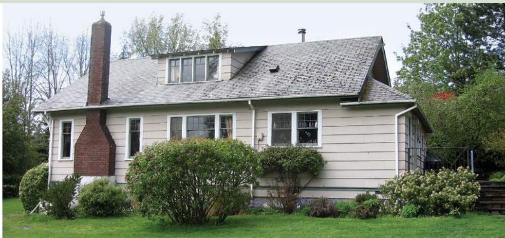
The east face of the farmhouse, before the renovation. This face would receive the most radical makeover, including a bump-out for the dining room. The enclosed north porch, at right, would rise to two stories.
