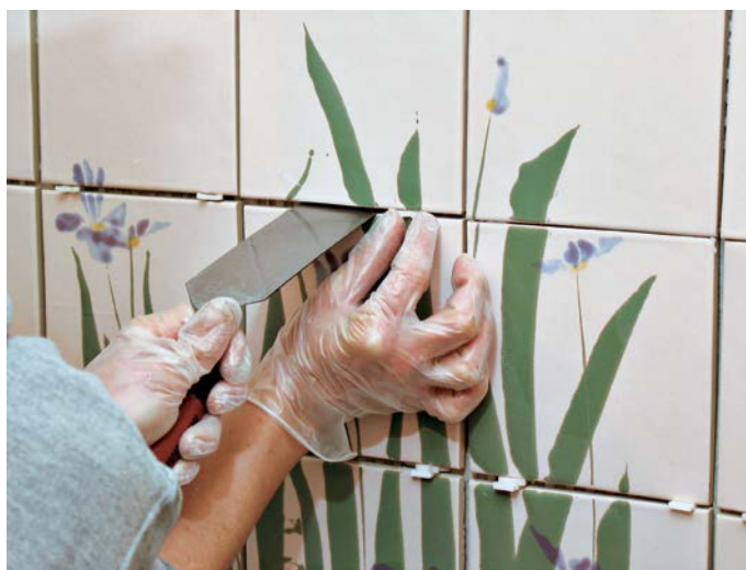
Because handmade tiles are irregular, they often need to be moved slightly after they've been set in adhesive. Use plastic shims to raise tiles so they're level with others in the course.
