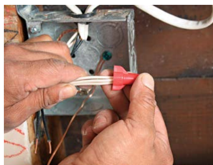
Strip about \frac{1}{2} in. of insulation from wire ends, and splice like-wires together.
