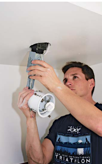
11. Feed the cable and the now-wired fixture into the hole.
