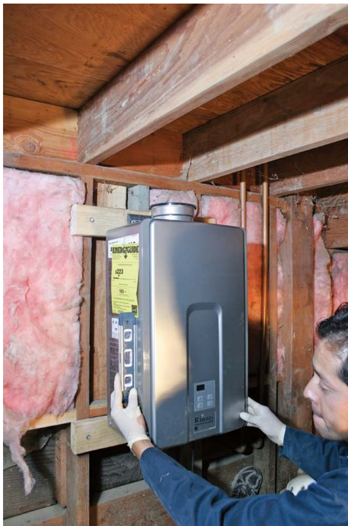
Plumb and mount the water heater. Just visible to the right of the unit are existing copper water pipes—a convenient place to tie the tankless unit into house lines.
