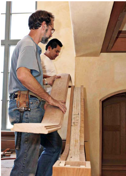
With skirt pieces glued and clamped to both sides of the rough cap, the finish railing cap is test-fitted.
