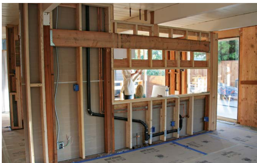
Kitchen wall framing, viewed from the living room. Running wiring and plumbing through one wall reduced the number of holes through the roof membrane.
