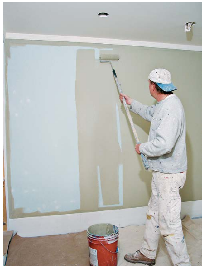
After unloading most of the paint on the roller in a zigzag pattern, spread it out evenly, top to bottom.
