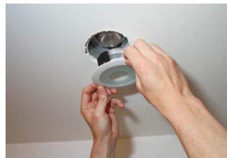
After turning off the power to the fixture and testing to be sure, remove the trim plate and screw out the incandescent bulb. The recessed can stays put.
