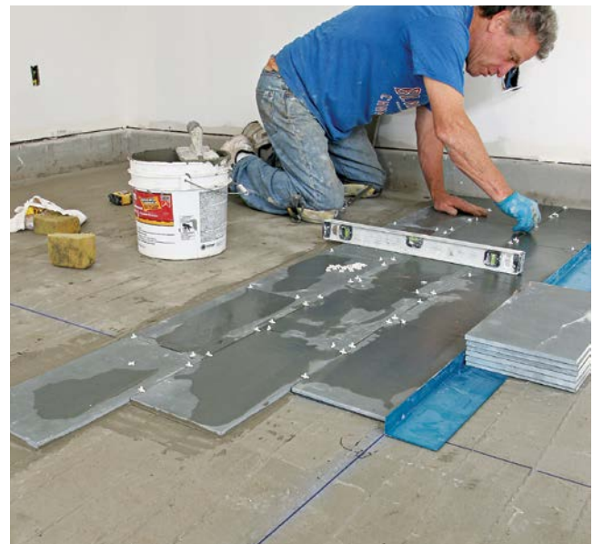
Installing an offset tile array is a bit trickier because every other row of tiles will cover one of the control lines. Here, the first tile in the first row sits within the intersecting chalklines, but the first tile in the second row is offset by 8 in., covering the chalkline.
