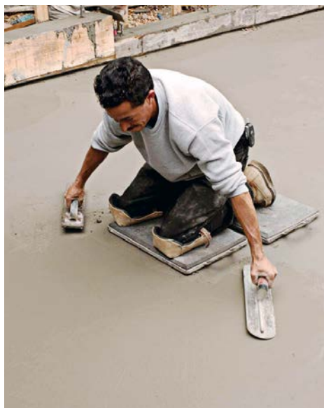
Finishing the slab. Start with magnesium or wood floats, and finish with a steel trowel for a smooth, hard finish. Knee boards distribute your weight as you work.
