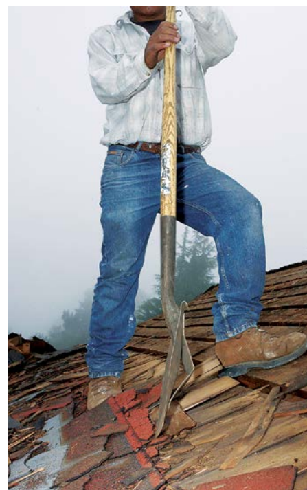
A stripping shovel is a flat-nose shovel whose blade is serrated to peel off shingles and grab nail shanks. The fulcrum on the back increases leverage as you pry up old nails and roofing.
