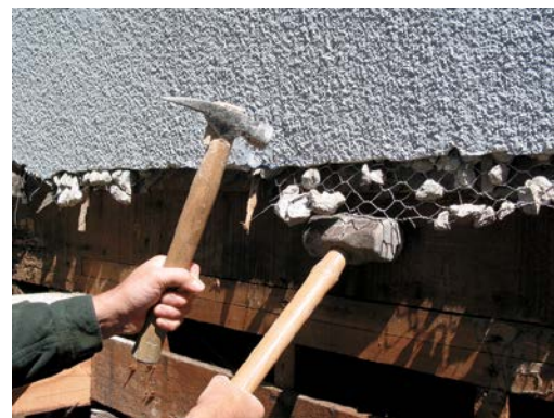
To remove stubborn chunks of old stucco from the wire mesh, pry up the mesh enough to slide the head of a hand sledge underneath so it can serve as an anvil. Hammered stucco will then pulverize. Wear eye protection and a paper respirator mask.
