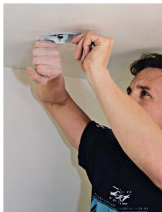
12. The lip of the can should sit flush to the ceiling; use your fist as needed to seat it.
