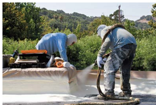
Spray foam adheres aggressively, so it’s important to mask everything you don’t want foamed. Here, polyurethane foam is being applied to the chimney. In the background is the masked-off parapet.
