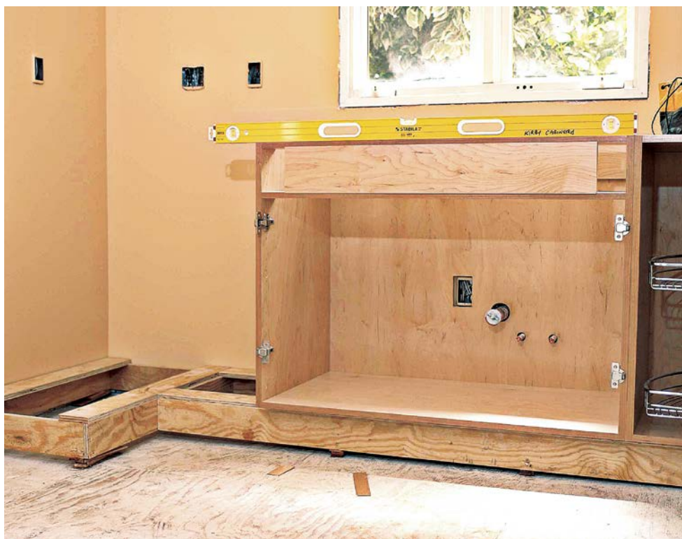
Once you've leveled the toekicks along a wall, start setting the base cabinets on top, and check them for level as well. If the cabinets are in an L- or U-shaped layout, work outward from a corner.
