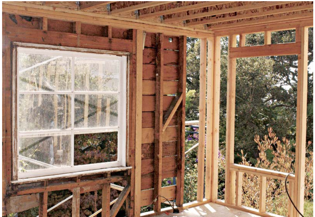
A skillful integration of old and new framing: After stripping interior surfaces and removing a wall to enlarge the room, carpenters installed a new 4x4 window king post and a third top plate to raise the old wall's framing. Note: Old and new window headers line up.
