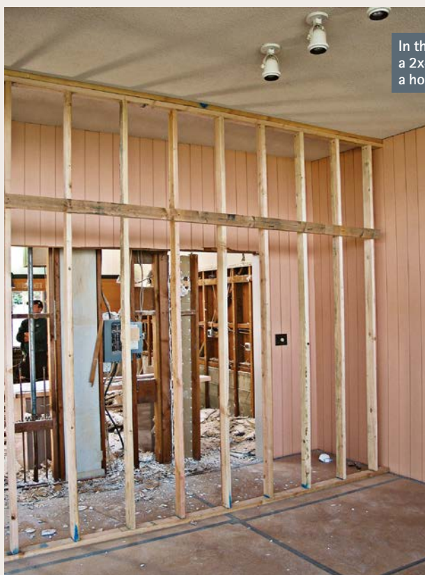
Screw jacks and a doubled 2x6 top plate pick up loads so a window opening can be safely enlarged. The floor shown is concrete. If yours is wood, use a 2x6 plate under the jacks as well.
