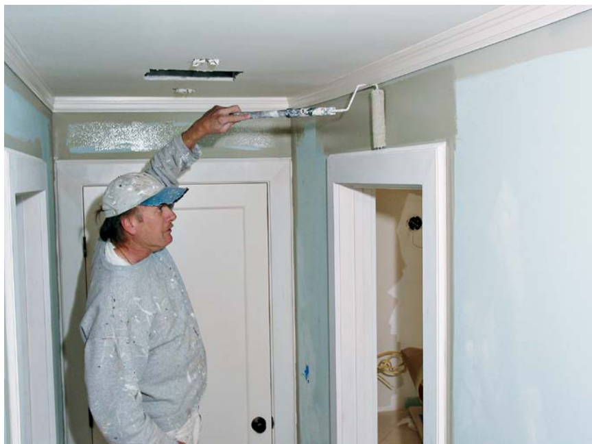
Use a hot-dog roller to fill those tight spaces over doors, around windows, inside cabinets, and the like.
