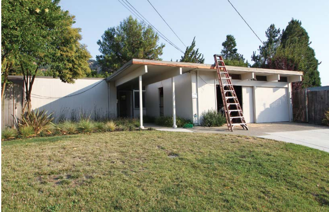
The flat roof of this 1957 Eichler-designed house was a good candidate for a polyurethane spray-foam roof.
