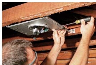
Then slide the can to fine-tune its position. Tighten the screws to lock it in place.
