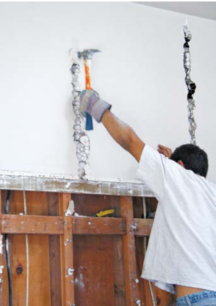
When demolishing, be as deliberate as possible. Here, a worker carefully breaks through old plaster so he can remove plaster and lath in manageable chunks.
