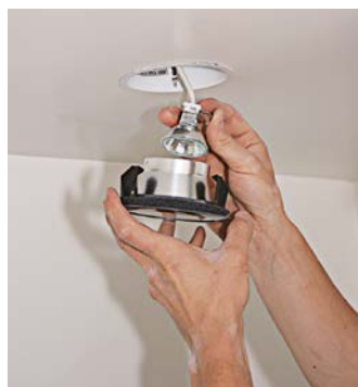
15. Install the trim assembly. The black ring in this assembly is a moistureproof gasket.
