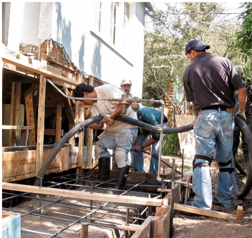
This 2-in. (interior diameter) concrete-pump hose is easier to handle than a 3-in. hose. But its smaller diameter requires smaller \frac{3}{8} -in. aggregate in the mix. Although a 2-in. hose is much lighter than a 3 in., tons of concrete pass through it—so you'll need helpers to support the hose and move it to the pouring points.
