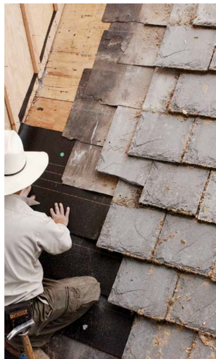
When replacing sections of slate or slatelike materials, alternate slate courses with strips of 30-lb. building paper. Century-old sheathing boards can become pretty hard, so if copper nails bend or deform, use stainless-steel roofing nails instead.
