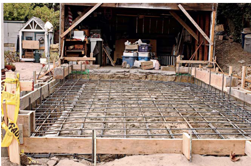
The garage floor is pretty typical of slab-on-grade foundations. Because it has only a single layer of rebar, it can bear the weight of walls only along its perimeter walls.
