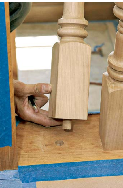
The doweled end of this square-cut baluster fits precisely into a hole predrilled into a stair tread.
