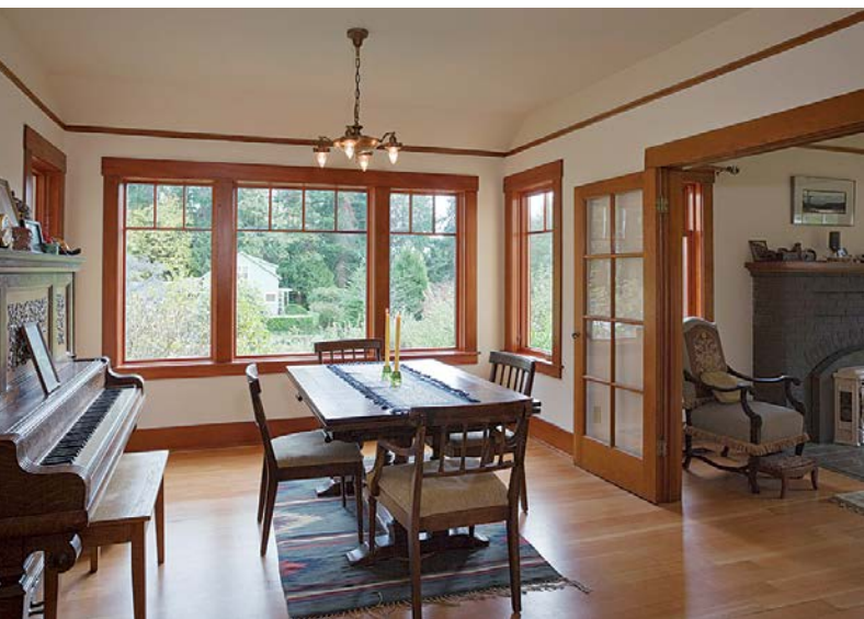
A cantilevered bump-out roughly 3½ ft. by 12 ft. created a dining room that comfortably seats more than a dozen guests. The fir flooring of the bump-out was rescued from the attic demo.
