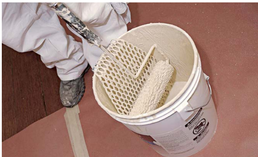
Expanded metal ramps allow you to load paint quickly and roll excess into the bucket. Note the building paper protecting the floor from paint spatters.
