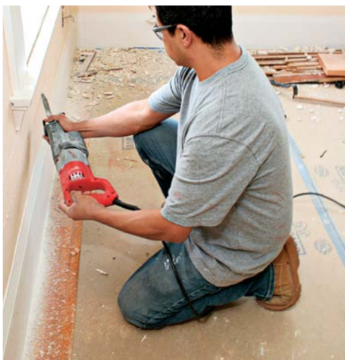
3. Cut along the chalklines, holding the reciprocating saw at a low angle so you don't cut into lath or framing.
