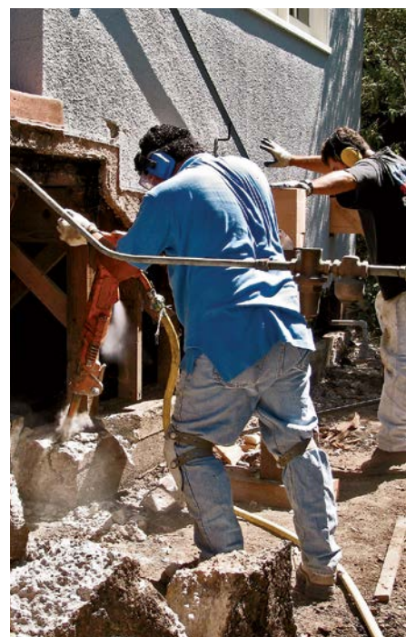
A 60-lb. jackhammer is powerful enough to bust concrete yet light enough to lift onto the foundation. Jackhammering is bone-rattling work, so have workers take turns at it.
