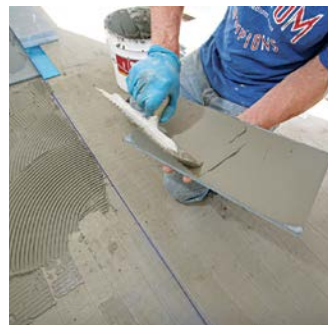
When tile thicknesses are slightly irregular, butter the backs of tiles with thinset adhesive in addition to troweling adhesive on the floor. That is, you'll butter the backs of all tiles, but apply varying thickness of thinset.
