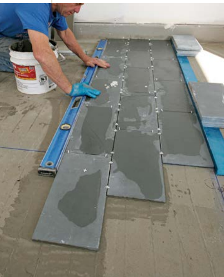
The tiler sets the first row of tiles all the way to the wall, places a straightedge along the edge of the row (at left), and weights down the straightedge so the first row won't move as he adds successive rows.
