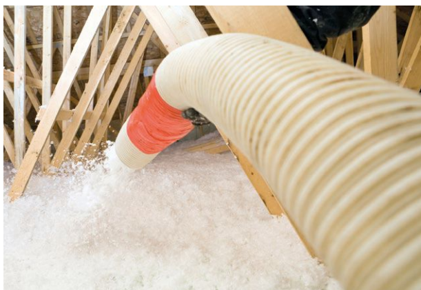
If access to your ceiling cavity is difficult, use a blow-in application
