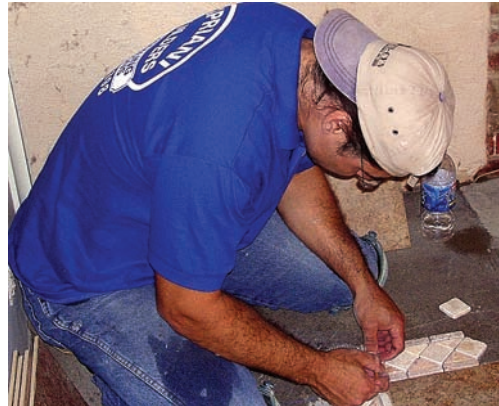
Edging tile is trimmed to fit on a wet saw.
