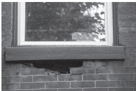
Proper window installation should include wall repair.
