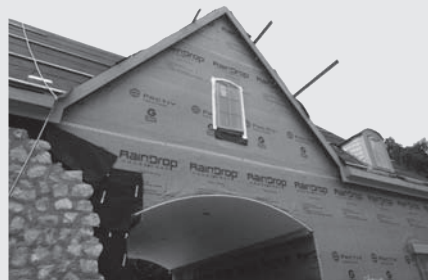
GreenGuard® RainDrop® housewrap, the industry's first woven housewrap with water drainage channels that move bulk water down to the base of the exterior wall (Photo courtesy of Pactiv Inc.).
