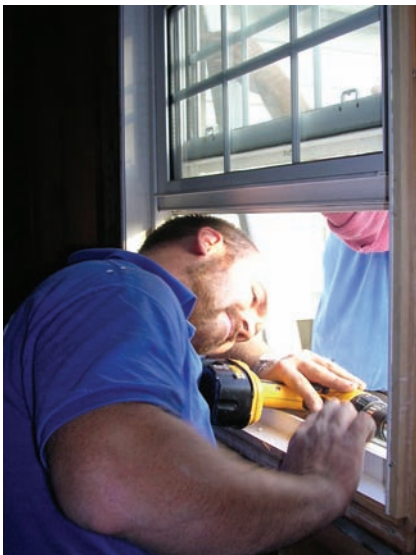
A window is installed in a frame with one worker working on the inside and another, outside.
