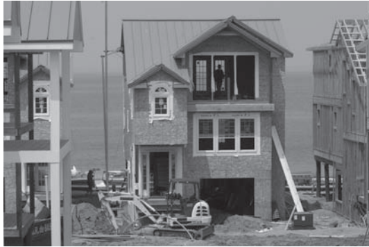
Simonton StormBreaker windows are installed on new construction on the oceanfront. The windows can withstand hurricane force winds and flying projectiles (Photo courtesy of Simonton).
