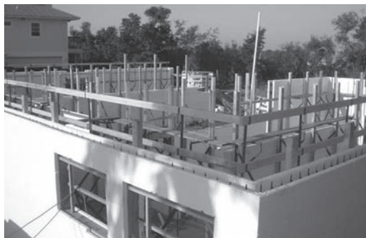
ICFs are used to create a house; included will be a safe room that will provide storage and shelter from the storm.
