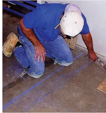
Using a notched trowel to spread the adhesive on which the tile will be laid.
