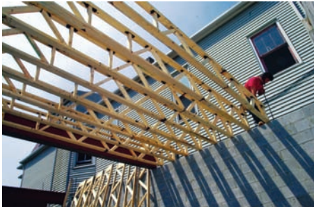
Framing the roof of an addition.
