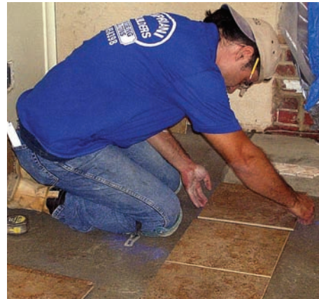
Making sure that the tile is aligned to the chalk line that designates the center of the room.
