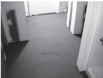
A wet bed is the traditional subfloor for ceramic tile floors.
