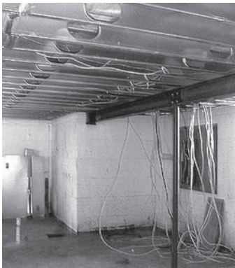
Light-gauge steel beams reinforcing a basement ceiling during a renovation have holes for wiring and plumbing prepunched before installation.
