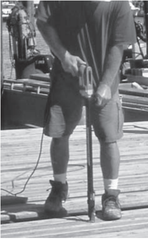
A drill attachment is used to put screws in decking to hold it to the frame.
