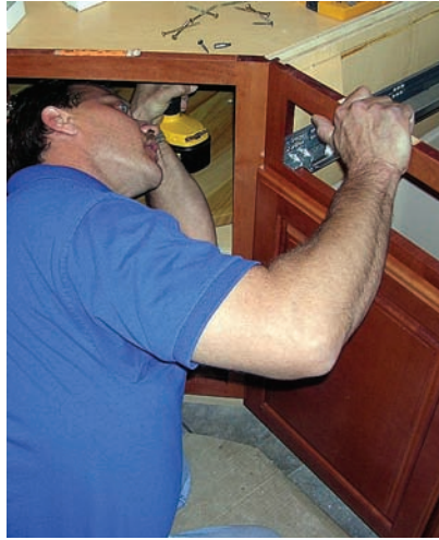
Installing the face frame on a base cabinet.
