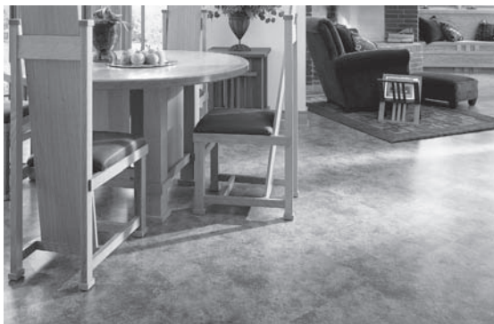
Laminate flooring can be made to look like tile. This flooring is glued rather than nailed to the subfloor.
