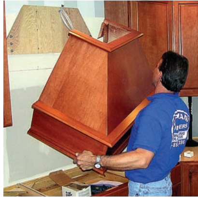
Lifting the cherry wood hood in place on the base.
