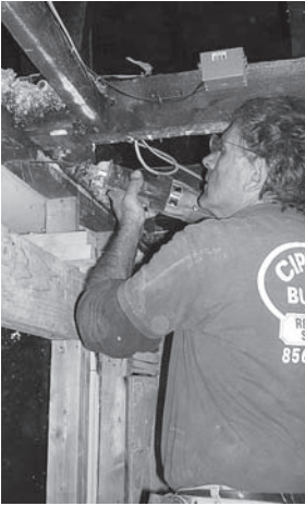
Old framing is cut away to make room for the new.
