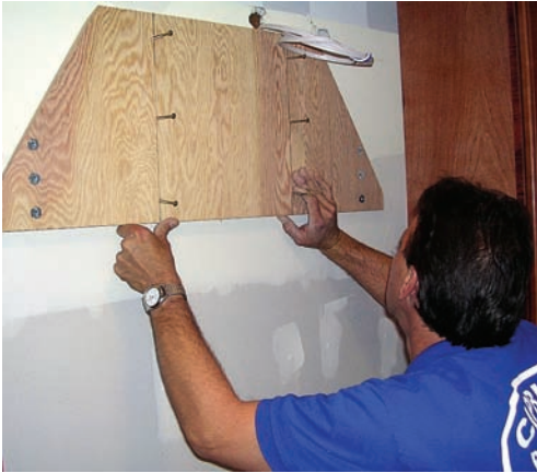
Aligning the plywood base on which the hood will be centered and installed.
