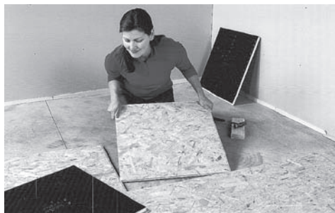
Two-by-two foot panels—wood on the top and corrugated plastic on the bottom are installed as a basement subfloor over concrete. The plastic keeps the cold and damp below the floor (Photo courtesy of SubFlor Advance).
