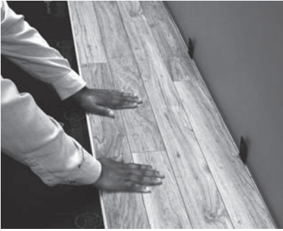
Laminate flooring simply snaps into place (Photo courtesy of Armstrong Flooring).
