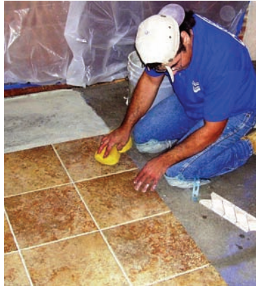
Making sure the grout lines are even.
