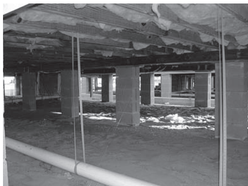
To prevent damage from flooding from storm surges, houses are built on pilings.
