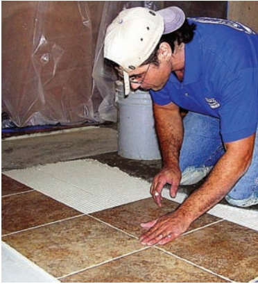
Adhesive is cleaned from the surface of the tile with a sponge before the adhesive dries.
