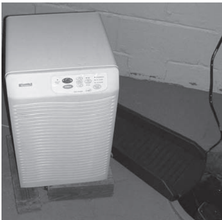
A basement dehumidifier set at 40 percent.
