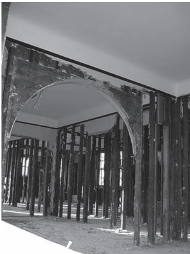
(Left) Mold created by flooding was eradicated by stripping the house to the studs.
