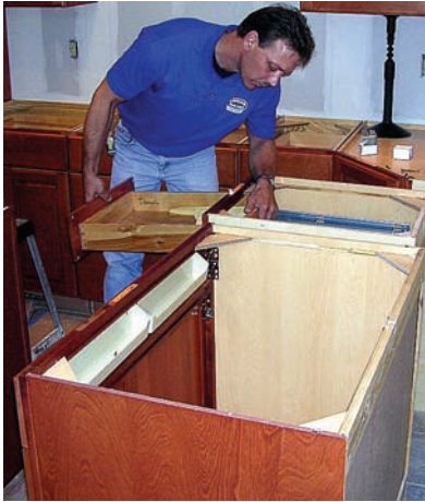
Checking drawer alignment in a kitchen base cabinet before installation.
