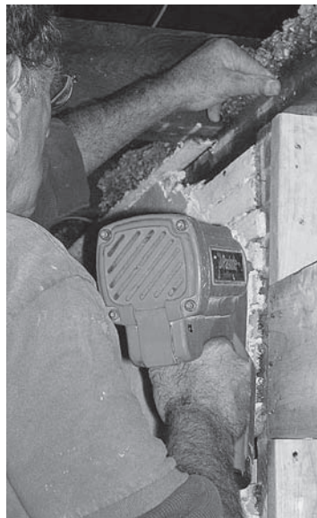
Framing out the master bedroom door.
