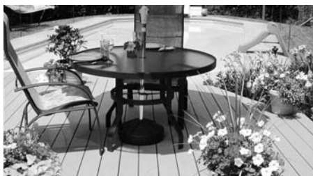
Composite decking is used on this play area near a swimming pool. Composite decking is virtually maintenance free.
