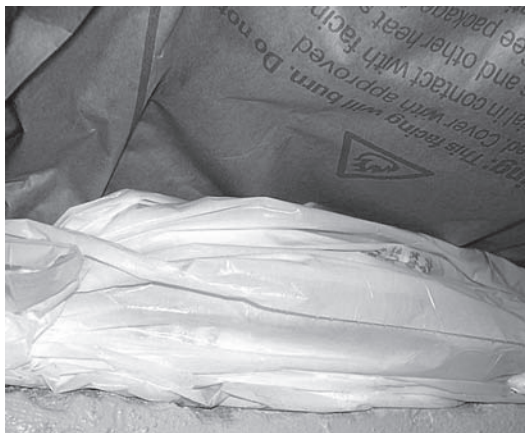
Air leaks can be sealed with a piece of unfaced insulation in a plastic kitchen bag. Any gaps around the seal can be filled with foam insulation.
