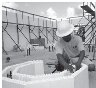
Insulated concrete forms have been shown to withstand hurricane force winds and stand up to storm surges (Photo courtesy of Greenblock).
