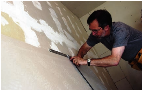
Measuring a cut on a sheet of drywall for installation.
