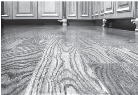
Hardwood flooring has found its way into the kitchen, thanks to baked-on finishes and quick curing polyurethanes that can withstand dampness and still let wood expand and contract.
