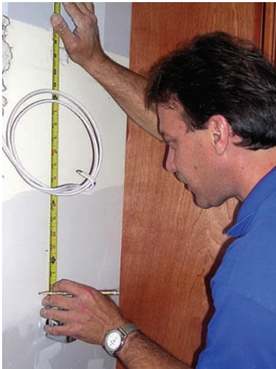
Taking measurements on the wall for vent-hood installation.
