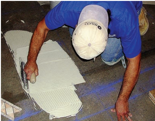
Fitting a tile into the adhesive.
