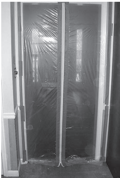
Cleanup of pollutants requires rooms to be sealed off.
