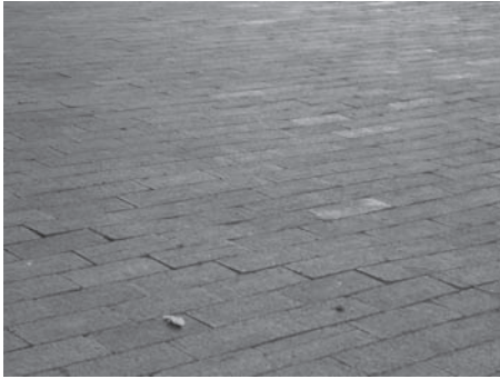
Brick pavers were used for this patio. Patterns are limited and there usually is a lot of cutting involved.
