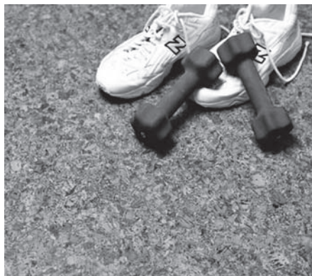
Cork flooring is easy on the feet, and appropriate for exercise rooms.
