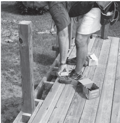
Decking is fitted between the posts before the railing is added.
