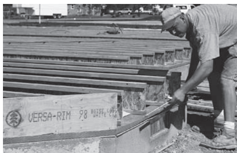
Floor joists made of engineered wood are used for an addition over a crawlspace (Photo courtesy of Boise Cascade).
