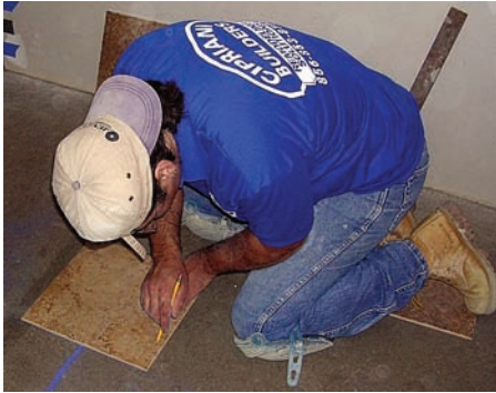
Snapping another chalk line from the center line on which the tiles will be aligned.
