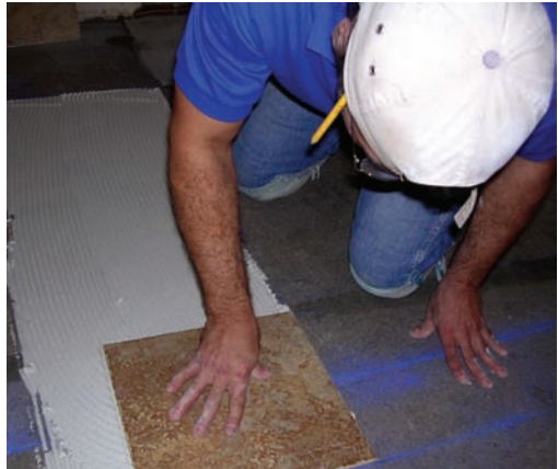
Making sure a row of tile is correctly aligned. One mistake and the tile would be off.
