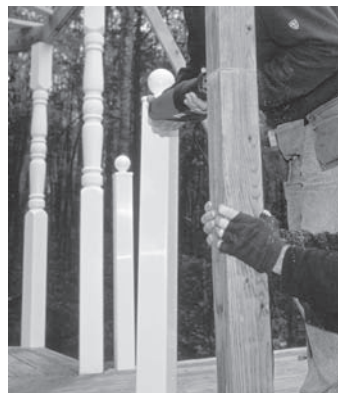
A reciprocating saw is used to cut the deck post to size before the vinyl railing is added.
