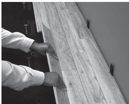
Tongue and groove laminate flooring is easy to install (Photo courtesy of Armstrong Flooring).
