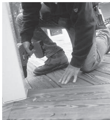
Pressure-treated decking is used in combination with vinyl railing for this deck.
