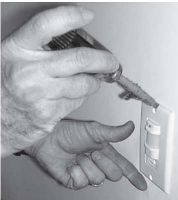
A light switch is controlled by motion.
