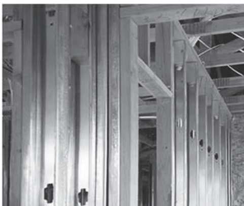
Wood framing is reinforced by light-gauge steel studs.
