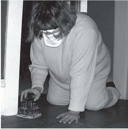
Sanding yellow pine is easy, and oiling where you've sanded can bring out the old floor.
