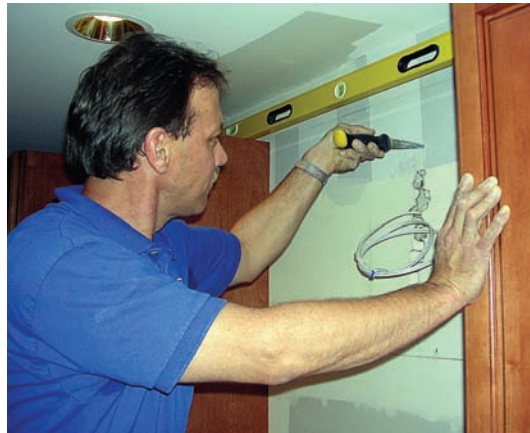
Using a drywall saw to make cuts for vent-hood installation.
