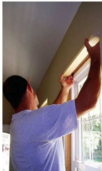
Trim is installed after a window installation.
