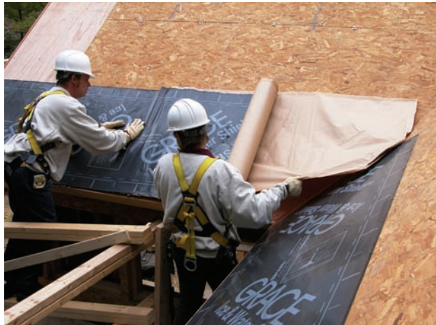
To prevent leaks from ice damming on a roof, a rubber membrane manufactured by W. R. Grace is installed.
