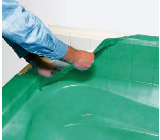
The excess acrylic is peeled away from the tile surrounding the tub after installation.
