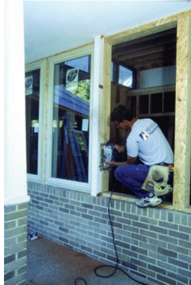
A window frame is trimmed before a window is installed (Simonton Windows).
