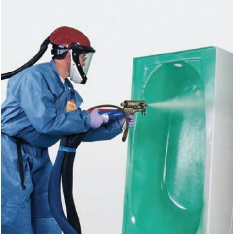
Acrylic spray is used to revitalize an old bathtub.
