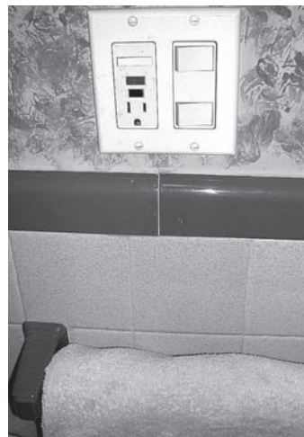
GFCI outlets should be installed in normally damp spaces such as kitchens, bathrooms, basements and out of doors. Switches for lights and heater fans in the ceiling are accessible from a wheelchair.
