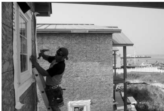
Windows are framed so that moisture intrusion is prevented during heavy rainstorms driven by wind (Photo courtesy of Simonton).
