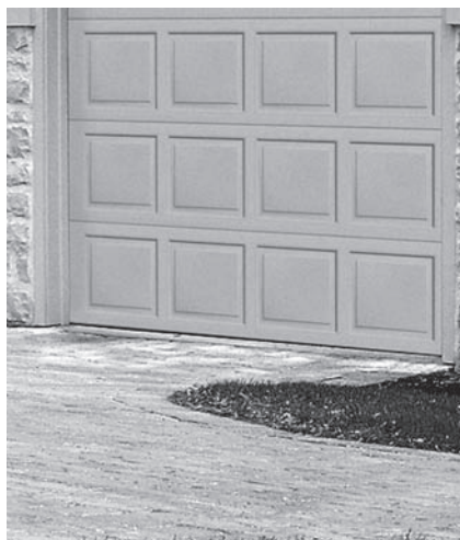
A hurricane-resistant garage-door retrofit.
