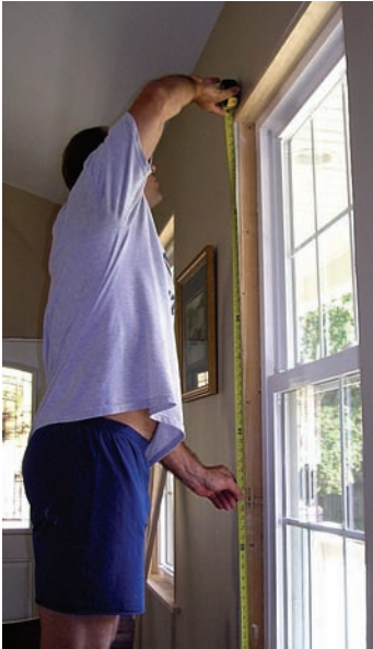
The window opening is measured carefully before the trim is installed.
