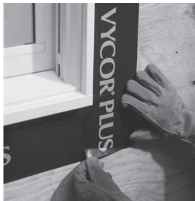
Windows are sealed to prevent moisture intrusion.
