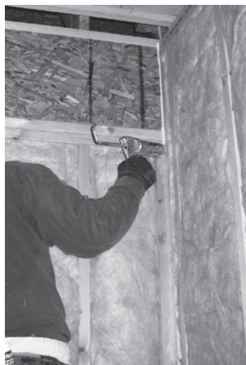
Fiberglass insulation cut to fit into framed openings is made completely tight with caulk.
