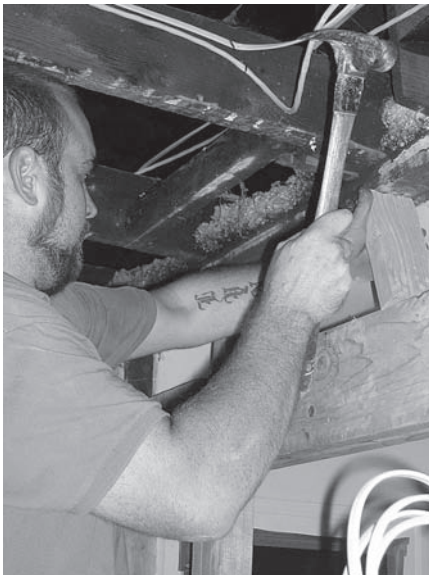
Renovation begins on a master suite in a 1930s-era house.
