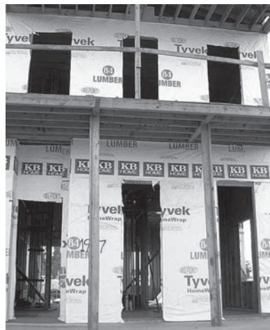
Tyvek is a house wrap building membrane, used to limit air leakage, and still allow breathability.
