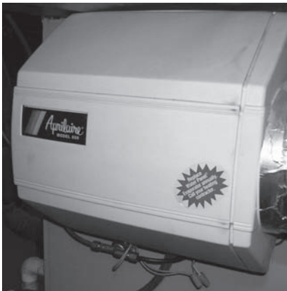
A whole-house humidifier adds moisture through the heating system.
