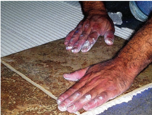
Edging tile is measured for the tile floor.
