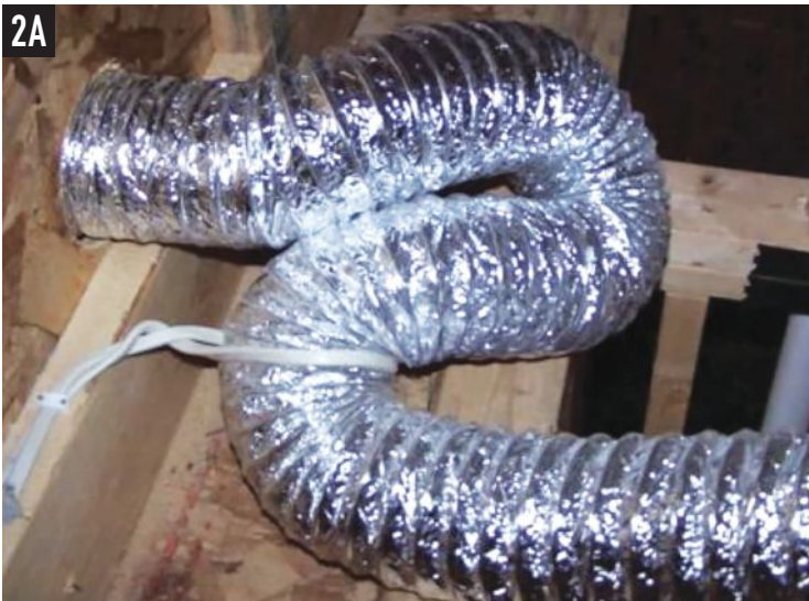
1 All ducts, whether rigid or flexible, should be sealed with UL-181-rated duct mastic. Duct tape has many uses, but sealing ducts isn't one of them.
