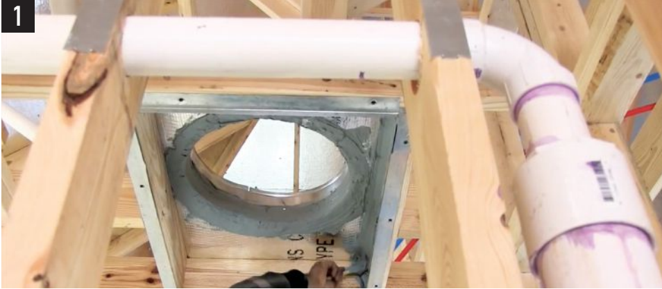
1 All ducts, whether rigid or flexible, should be sealed with UL-181-rated duct mastic. Duct tape has many uses, but sealing ducts isn't one of them.
