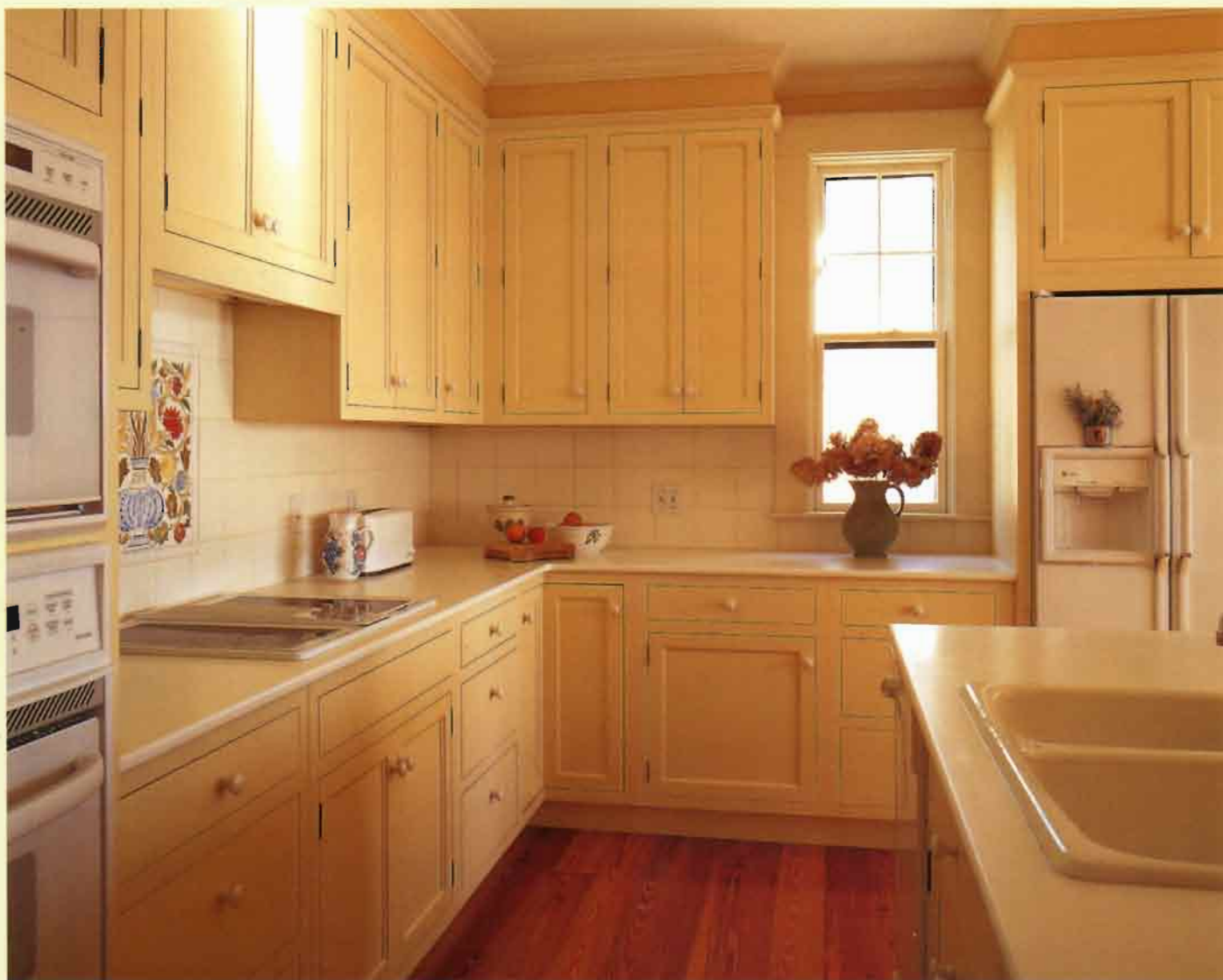
▲ A WHITE SOLID-SURFACE COUNTERTOP WITH EASED EDGES brightens an urban kitchen that has only one window. Flat white 4-in.-square tile makes a water- and heatproof backsplash. The space between the cabinets is filled with flat trim topped with crown molding and painted a darker gold to match the softwood floor.
