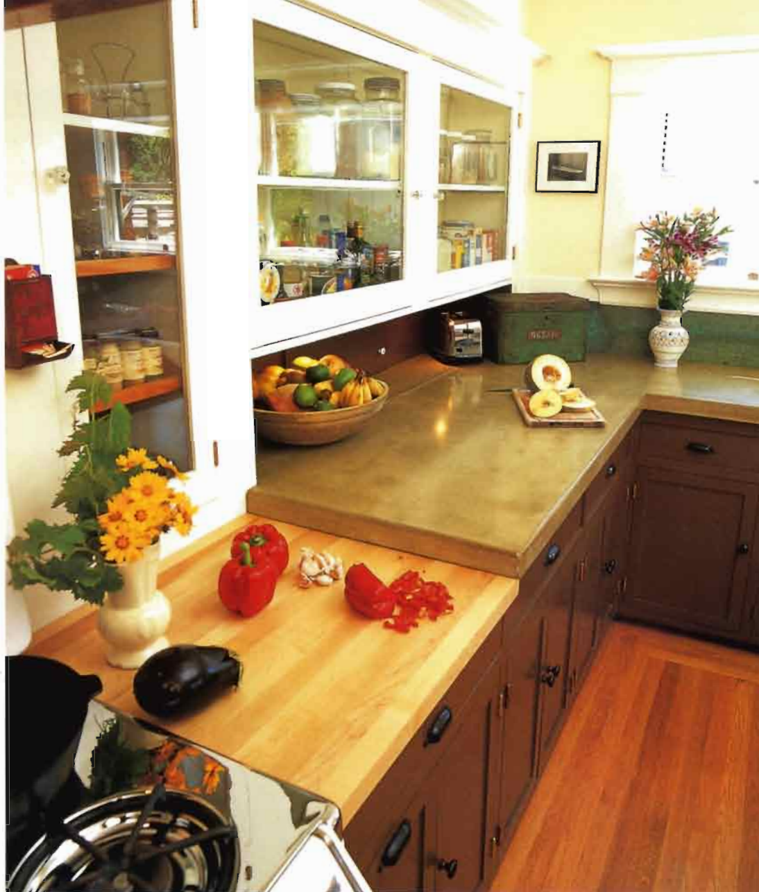
THIS THICK, GREEN-TINTED CONCRETE COUNTERTOP WAS PRECAST on site and lifted into place on cabinets original to this 1920s bungalow. Concrete gives way to a lowered butcherblock counter next to the restored 1940s range.
