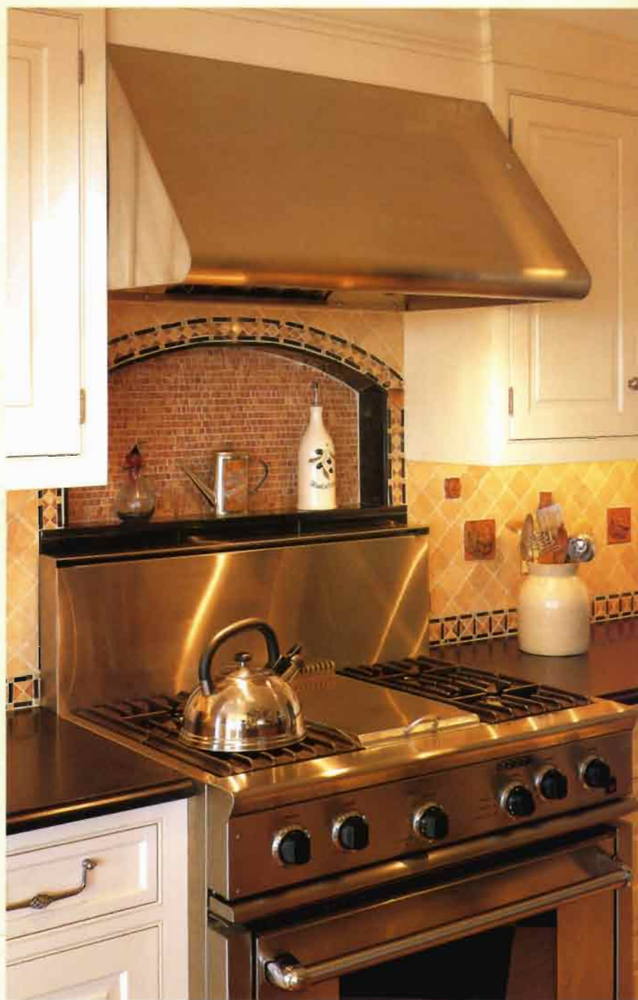
▲ THIS BACKSPLASH IS TUMBLED MARBLE WITH INSET ceramic tiles, each with a charming bas-relief face. Contrasting mosaic stone tile fills and frames the arched recess over the downdraft vent/backsplash. The countertop is honed "Absolute Black" granite with a Dupont profile.
