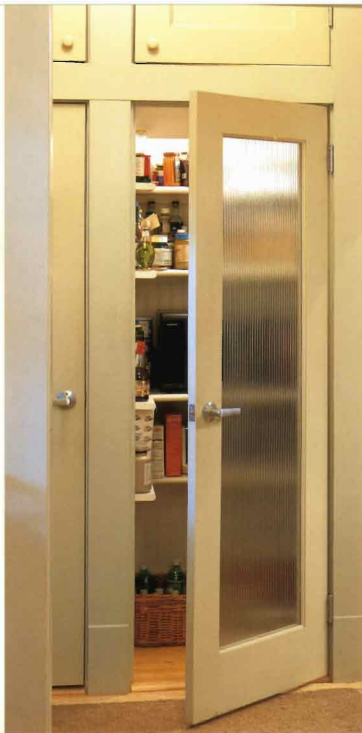
▲ THE FIXED, BULLNOSED SHELVES IN THIS WALK-IN PANTRY are supported by cleats on beadboard paneling, and they've been spaced to accommodate items of varying heights. It's easier to scan the pantry quickly when shelves are narrow. A ribbed-glass door blurs contents (good for those messy days).
