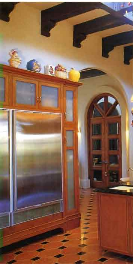
▲ A FULL-SIZE REFRIGERATOR AND A SEPARATE FREEZER are built into a 10-ft.-tall cabinet with frosted-glass doors and birch veneer case and doors. The assembly is scaled to fit a large kitchen built for big parties.
