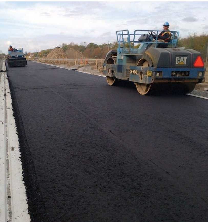
Digram Developments focuses on site servicing, including asphalt work, sidewalks and curbs.
