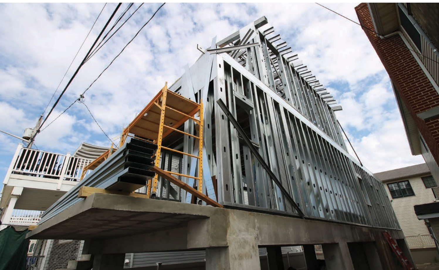
Metal studs with drywall in effect create a second home inside the concrete house.
