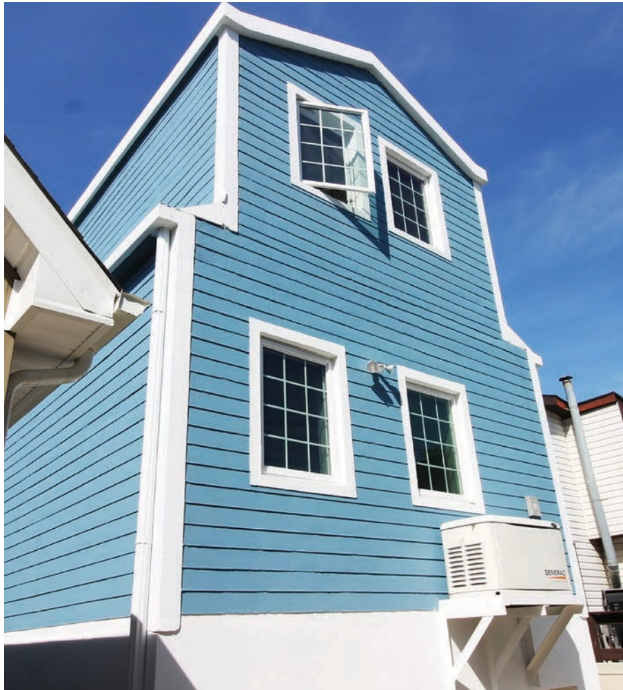
Leeward Living subcontracts the electrical, plumbing and HVAC work on its concrete homes.
