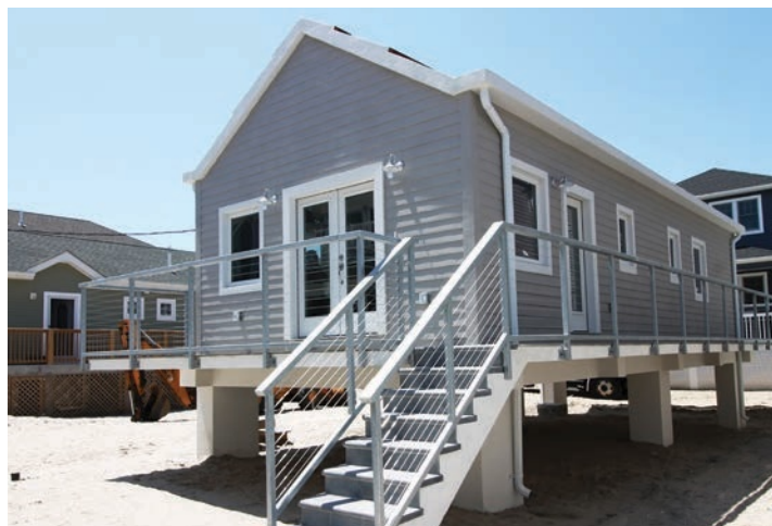
Leeward Living elevates houses on platform decks designed per FEMA guidelines.
