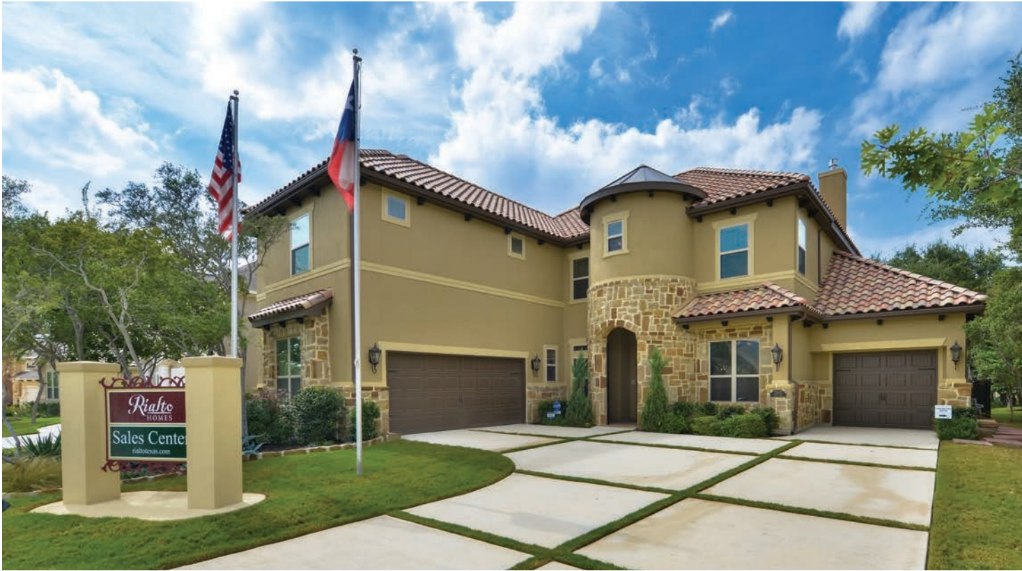
Rialto Homes builds for homeowners looking to “move up” in the quality of their homes.
