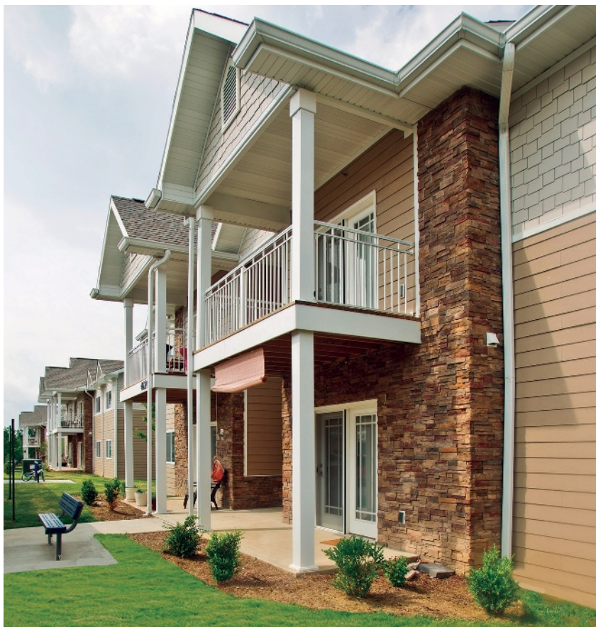
The Chandler Bay Apartments in Missouri achieved LEED certification by using energy-efficient techniques.
