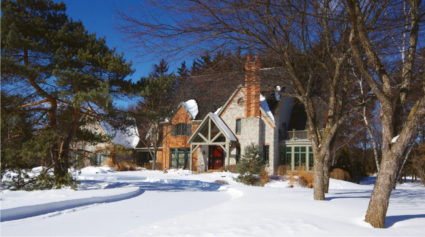
Many of Hemphill Builders' homes feature a split-face natural graystone, which is difficult to find in its Midwest market.
