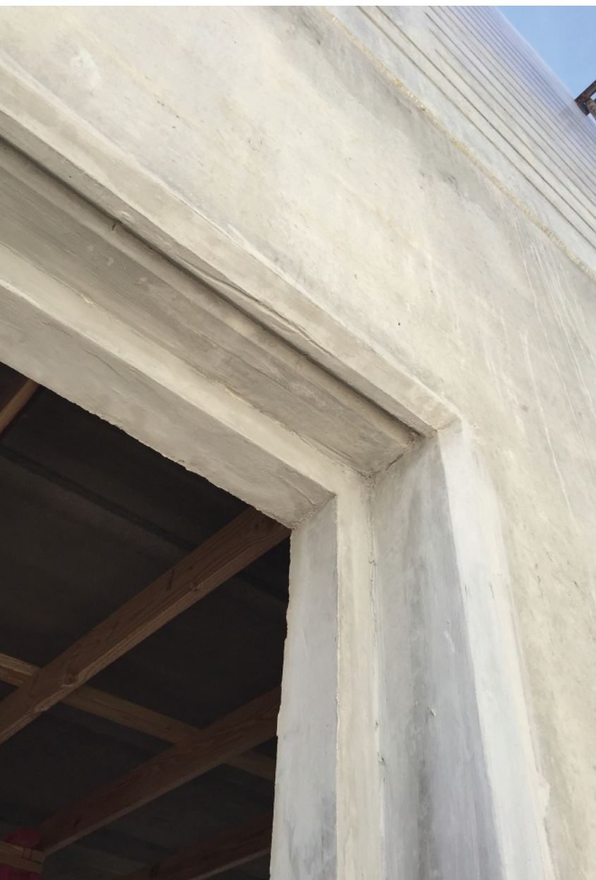
CFH can use technology in concrete casting to mimic wood siding to the point where a difference can only be found through close examination. In addition, its building system provides sustainability.
