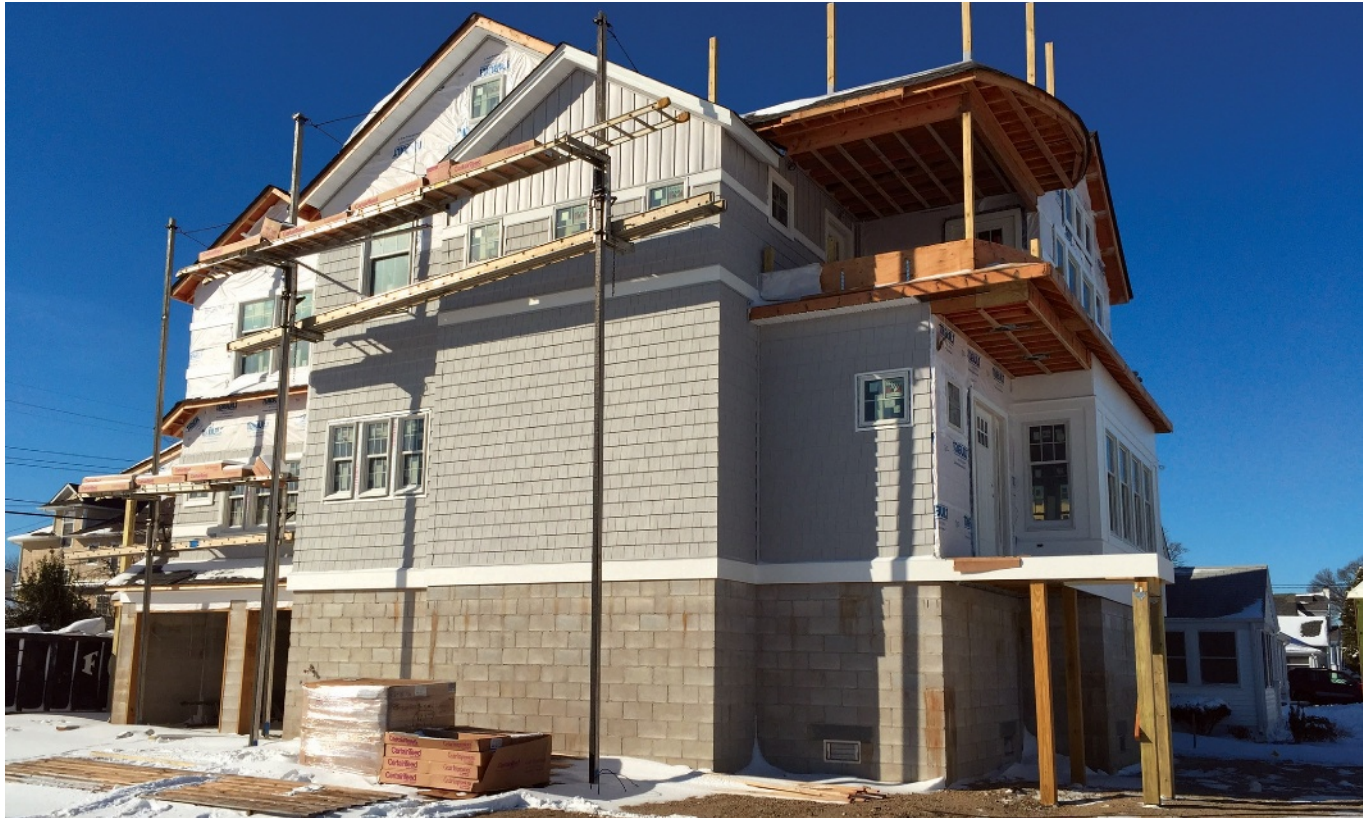
Menard Construction's expertise in restoring and recreating unique homes is helping it rebuild Jersey Shore neighborhoods that were hit by Hurricane Sandy.
