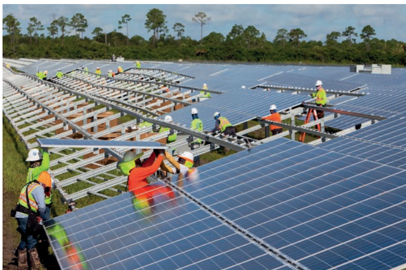
Black & Veatch crews work to expand Florida Power & Light's solar photovoltaic capacity at the Babcock Ranch, the first solar powered city in the US
