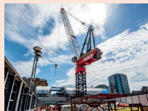
Marr's M1680D HLL is installed at Central Station to complete heavy lift and general construction requirements
