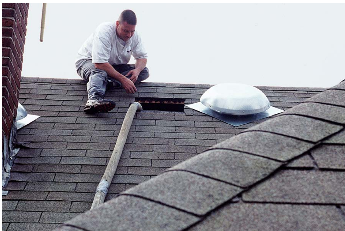
If there's no access into the attic, you can cut an opening for a roof vent. Climb in and insulate, then install the vent to cover the hole.
