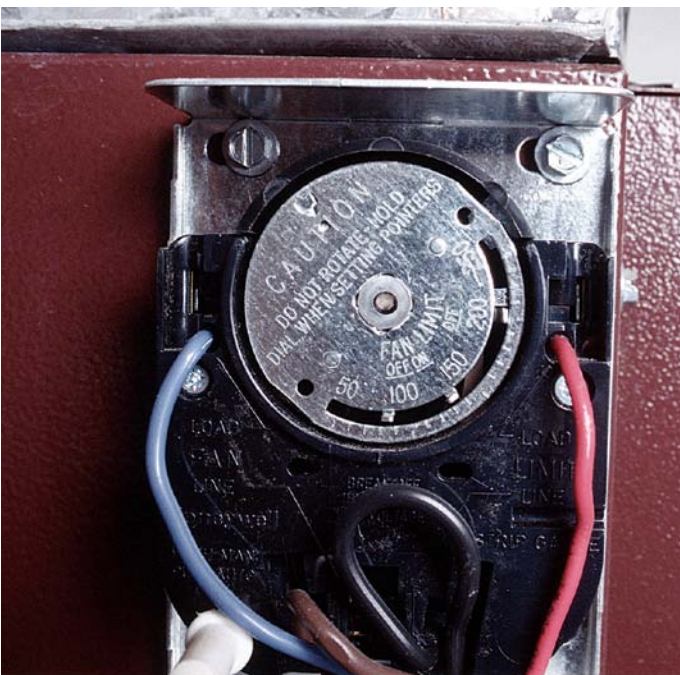
The blower control turns on the fan when it senses heat from the burner. The fan's on and off temperatures (the tabs at the bottom of the dial) must be set properly for maximum efficiency. This one also has a built-in adjustable peak limit (the tab on the right side of the dial).
