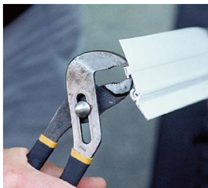
After trimming a door sweep to size, crimp the ends to hold the rubber strip in place.
