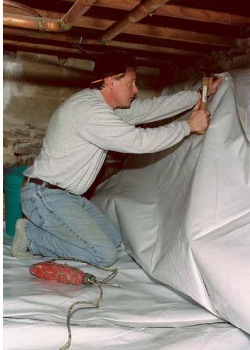
Plastic button anchors (see inset: Outwater Plastics; www.outwater.com ) can be pressed into ¼-in. holes drilled with a hammer drill. One button every 3 ft. can support even a heavy liner.
