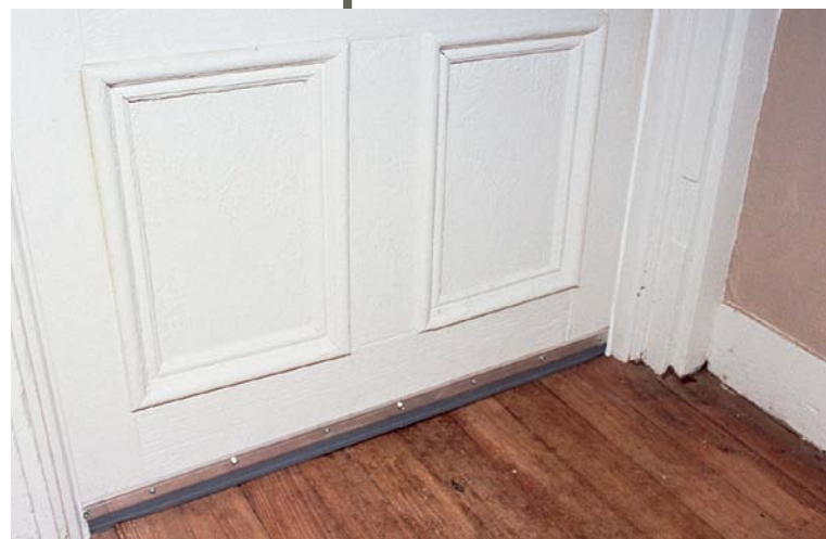
This door sweep lifts out of the way when you open the door, riding clear of carpets and uneven floors.
