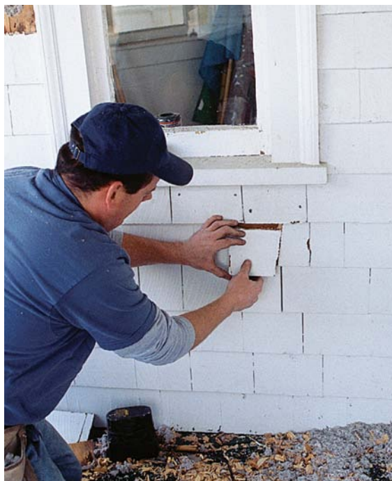
Once the hole is plugged, set the shingle or siding in place and attach with siding nails.
