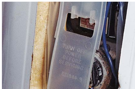
This tank is insulated with urethane foam. A tank with insulation rated R-10 or higher won't benefit much from an insulation wrap.
