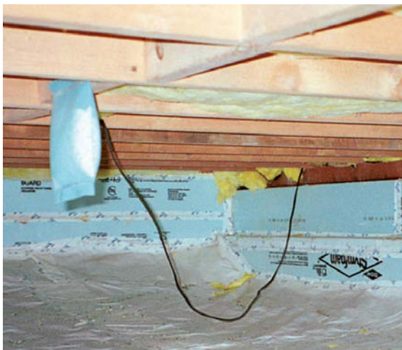
The insulation on these crawlspace walls was carefully sealed to the vapor barrier on the floor, creating a warm, dry space.
