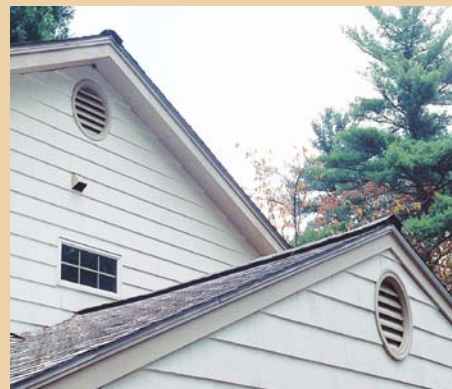
Passive roof vents are designed to transport moisture out of attics.
