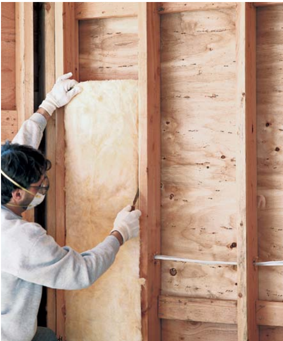
Use a putty knife or a 6-in. taping knife to tuck the back corners of batts into place to help prevent the corners from rounding. When fiberglass batts are properly installed, you’ll get much closer to the R-value you paid for.
