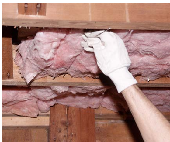
Push rods are used to hold unfaced fiberglass insulation batts in place in the floor joists. It's important not to compress the fiberglass too much with the push rods.
