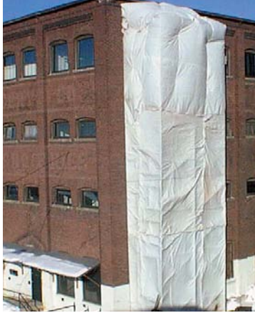
This photo of a building under construction displays the air pressure pushing the tarp out at the top and in at the bottom. This clearly shows the pressures that move air through a building in winter.
