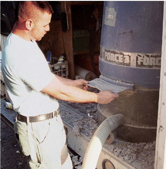
On this machine, you increase the air-to-cellulose mix for dense-packing by closing a gate in the hopper, which reduces the material feed. Other machines have air-inlet ports that open to increase the air pressure; either type will adjust the air-to-material ratio.
