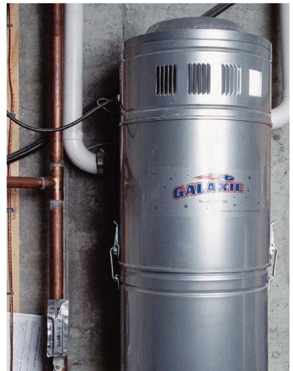
A central vacuum system, if it vents to the outside, can also act as an exhaust appliance in the home.
