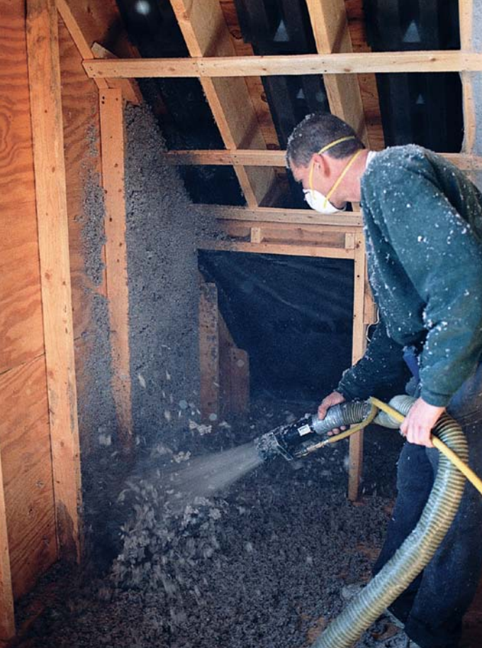
Damp-sprayed cellulose installs quickly and completely fills wall cavities.
