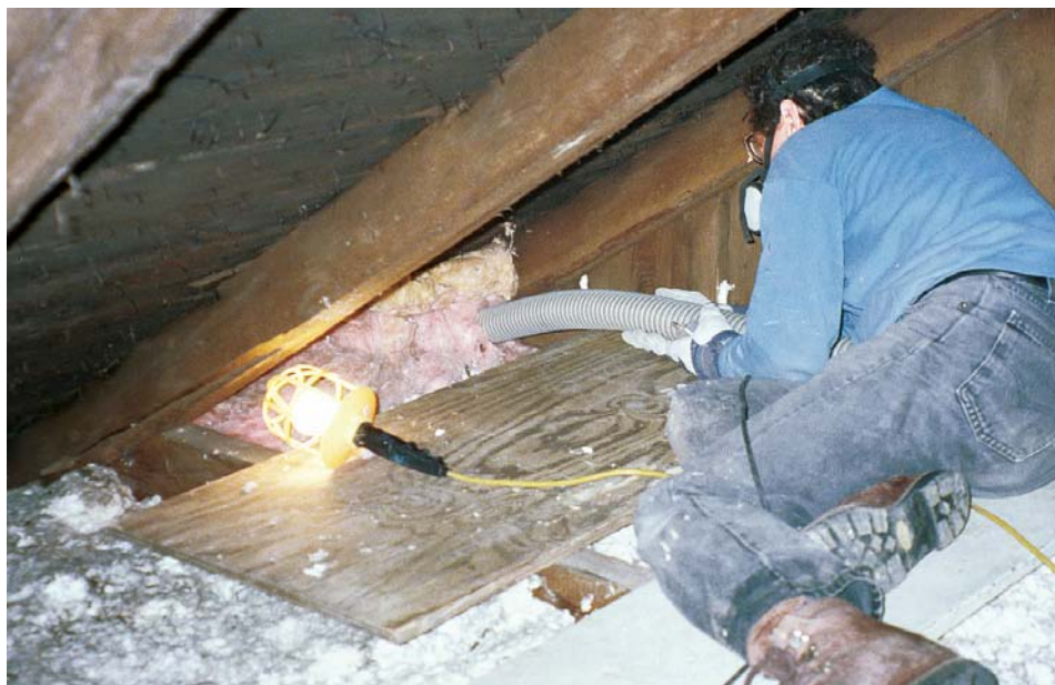
When insulating a closed cavity, such as this rafter bay, hold a piece of fiberglass batt across the opening. Wear a respirator and safety glasses in case the cellulose blows back at your face.
