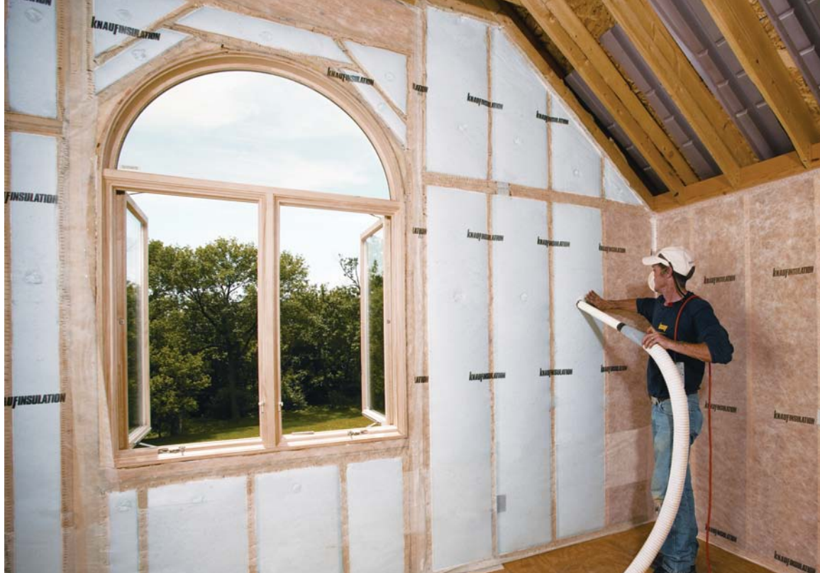
High-performance fiberglass can be blown into open walls behind netting, as shown, or used for effective dense packing in closed cavities.
