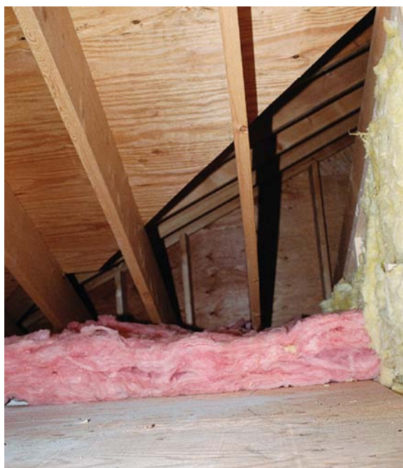
Sometimes, small dormer attics may be hidden behind the roof sheathing; in this case, fortunately, the attic is visible and easily accessed.
