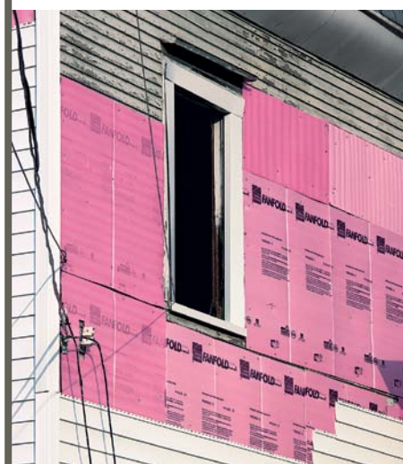
The backerboard that's installed underneath vinyl siding is mostly for the convenience of the installer.
