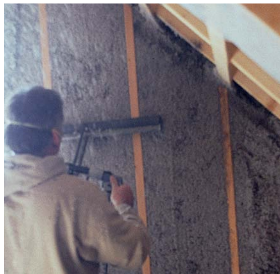
After spraying the damp material, a worker scrubs off any excess with a special rotary brush, leaving the wall perfectly flat.
