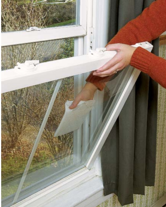
A tilt-out sash is one useful feature found in many replacement windows.
