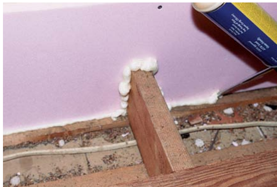
Sealing the floor bays with foam board is the air-sealing equivalent of closing up two to four large, open windows.
