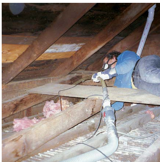
Some walls in older houses open into attic areas. Before you start drilling, check for this situation—you'll save yourself a lot of drilling if you can insulate the wall cavities from above.
