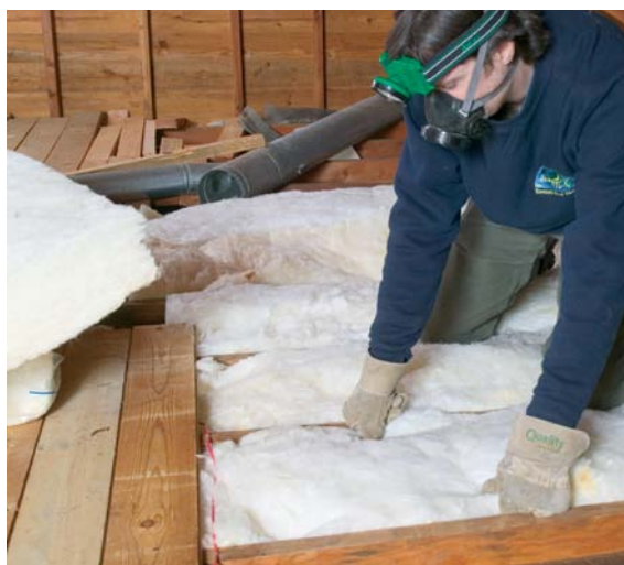
Tuck the first layer of batt insulation into each ceiling cavity as neatly as possible. These unfaced batts are being installed right over the existing 1½-in. faced insulation.
