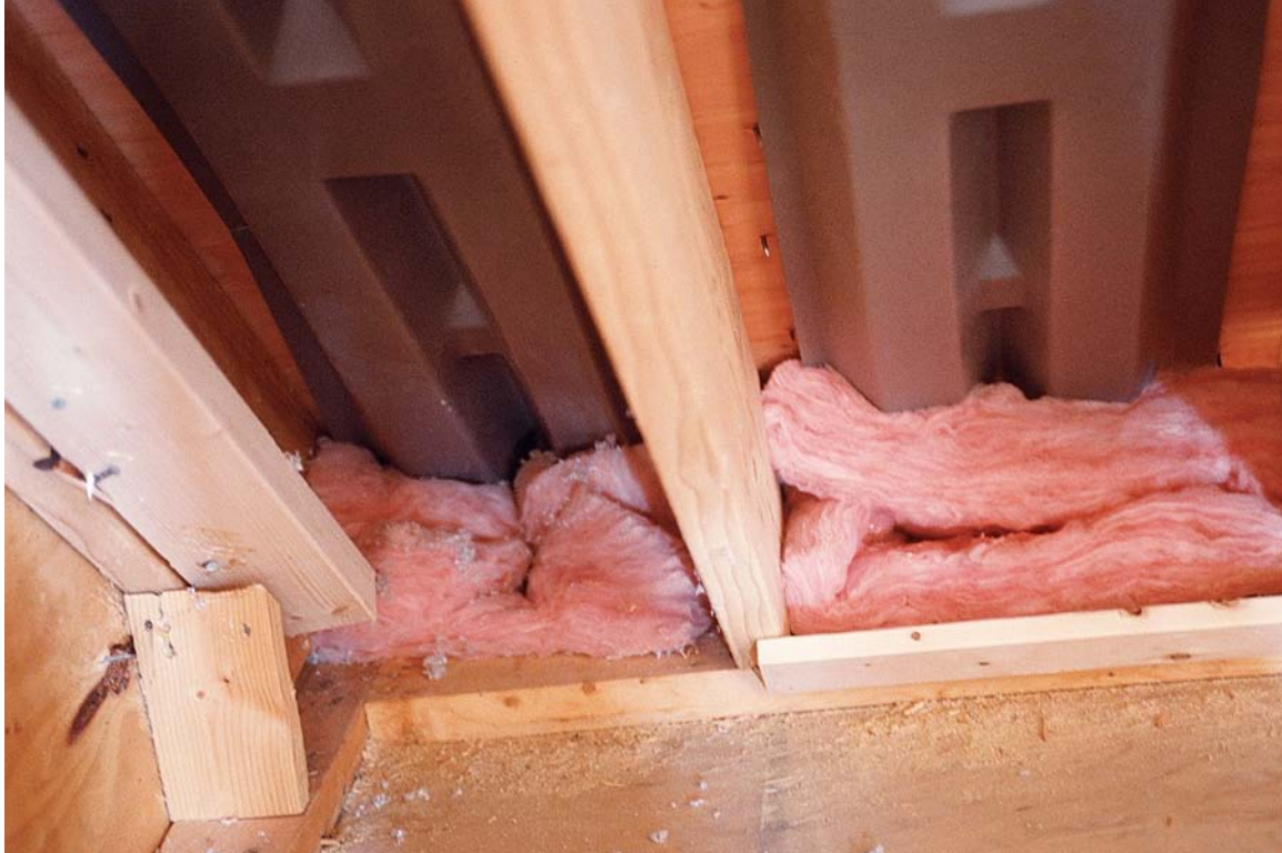
Standard foam vent chutes can be held in place with fiberglass batts and pushed in tightly to cut down on wind washing.
