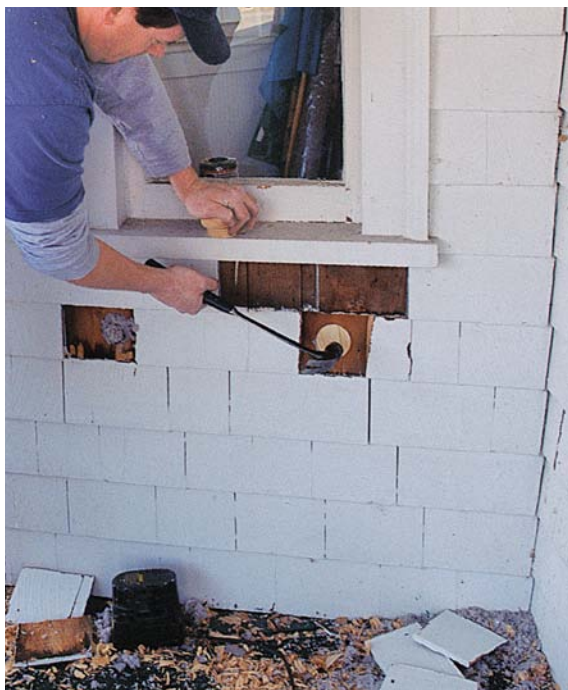
Be sure to plug any holes cut in the sheathing, even if the siding will cover them later. Precut tapered plugs are generally available from a cellulose supplier.
