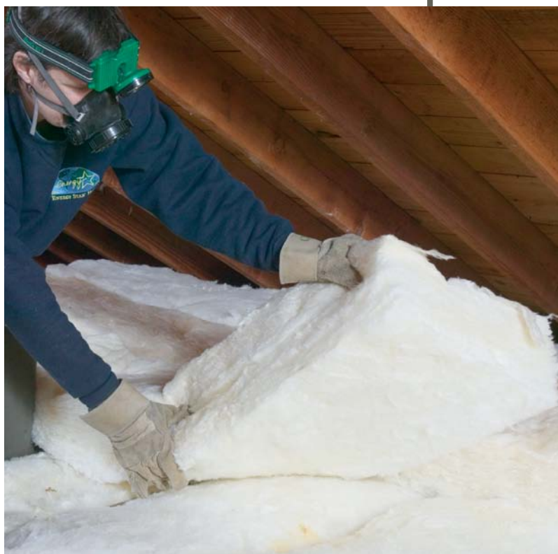
Tuck the first layer of batt insulation into each ceiling cavity as neatly as possible. These unfaced batts are being installed right over the existing 1½-in. faced insulation.
