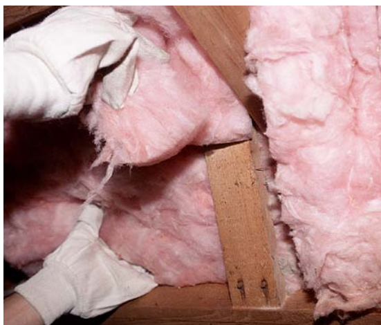
Fiberglass batts must be carefully cut and woven around any bridging, blocking, or other obstructions in the floor framing.
