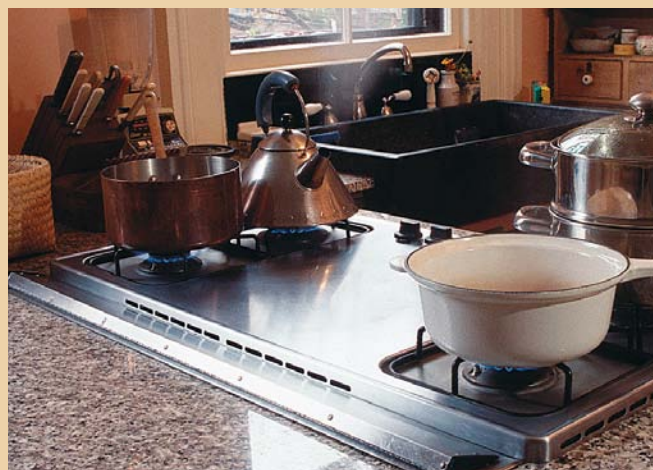
Kitchens are another source of moisture; range hoods should always be vented directly to the outside.
