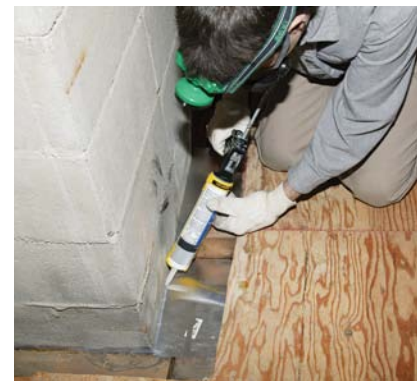
Any draft-stopper installed within 2 in. of the chimney must be made of a material that won't burn.
