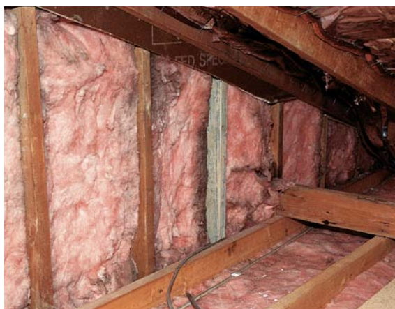
This attic area behind a kneewall has insulation in the floor, wall, and rafters, so it's unclear whether the area is inside the conditioned space. In this example, the thermal boundary is ambiguous.
