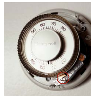
The anticipator is a sort of timer that prevents the furnace from firing too long as the house heats up. Setting the pointer correctly can improve the furnace's efficiency and your comfort.
