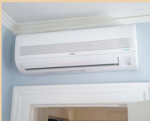
The inside half of a ductless mini-split typically mounts high on a wall. Other configurations are available, such as a small hidden air handler.
