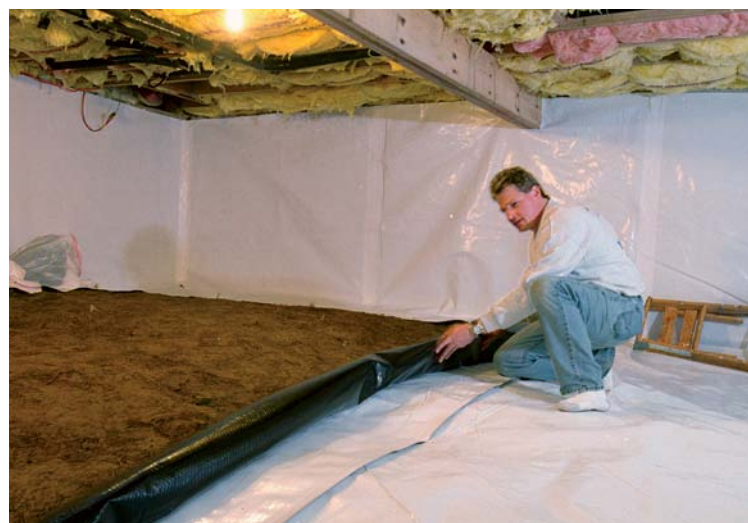
After the vapor retarder is hung on the walls, spread the overlapping piece on the floor. Be sure to seal it carefully at all edges and penetrations.
