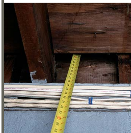
In some cases, walls are framed so that the bays open into the basement. Stuff the bottoms of these wall bays with fiberglass before blowing insulation.
