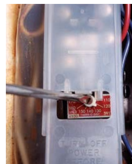
The thermostat on an electric water heater can usually be changed with a small screwdriver. Setting the temperature requires some trial and error, because the thermostat markings are often inaccurate.
