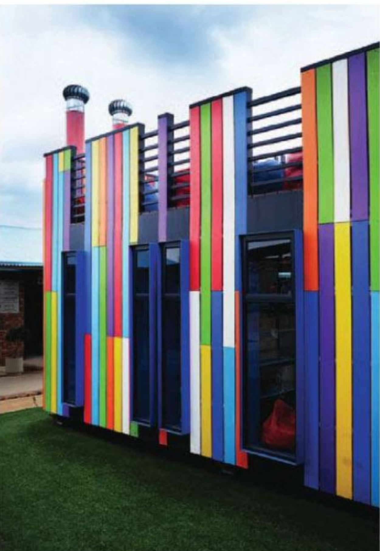
A desolate patch of land has been replaced with synthetic grass on which the children can play. BELOW AOJ's design was inspired by colour, shape, light and the children at MC Weiler Primary School. OPPOSITE The SEED Library opened its doors in 2012 after over two years of planning, designing and construction.
