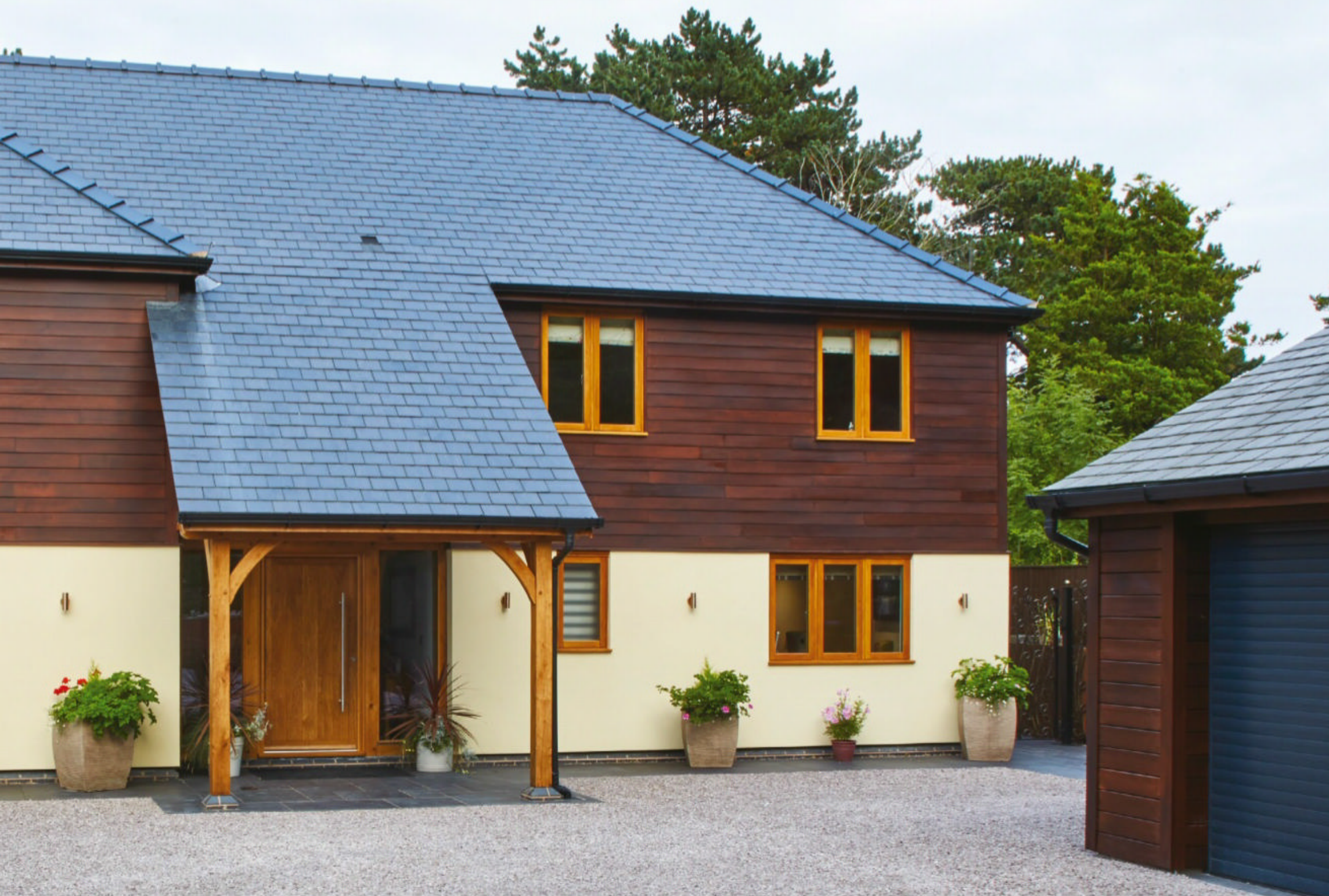
THE GARDEN ROOM In addition to the main house, the plot now features a garden room with a jacuzzi and a small snug. The garden room was designed to emulate the main house with its oak frame, timber cladding and Spanish slate roof.
