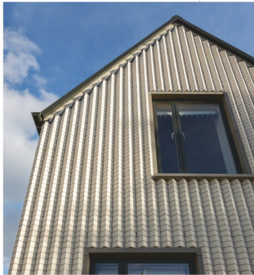
ABOVE: Bricks (supplied by Bea Clay Solutions) have been laid at 90° creating a striking aesthetic that gives this house its own contemporary identity.
