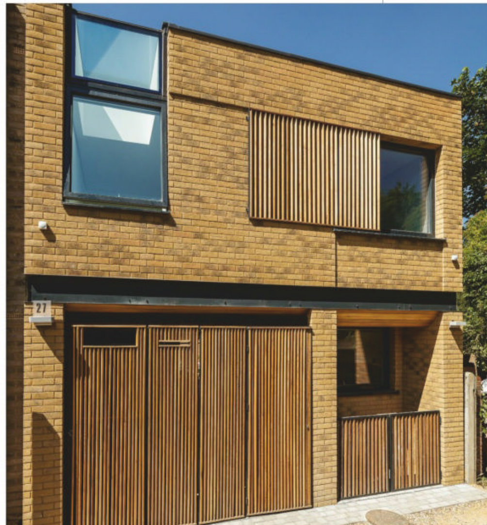
BELOW: This Passivhaus-certified self-build was constructed from structural insulated panels (SIPs) and is clad in brick slips to meet planning requirements. The brick and steel façade has been softened with red cedar louvres.
