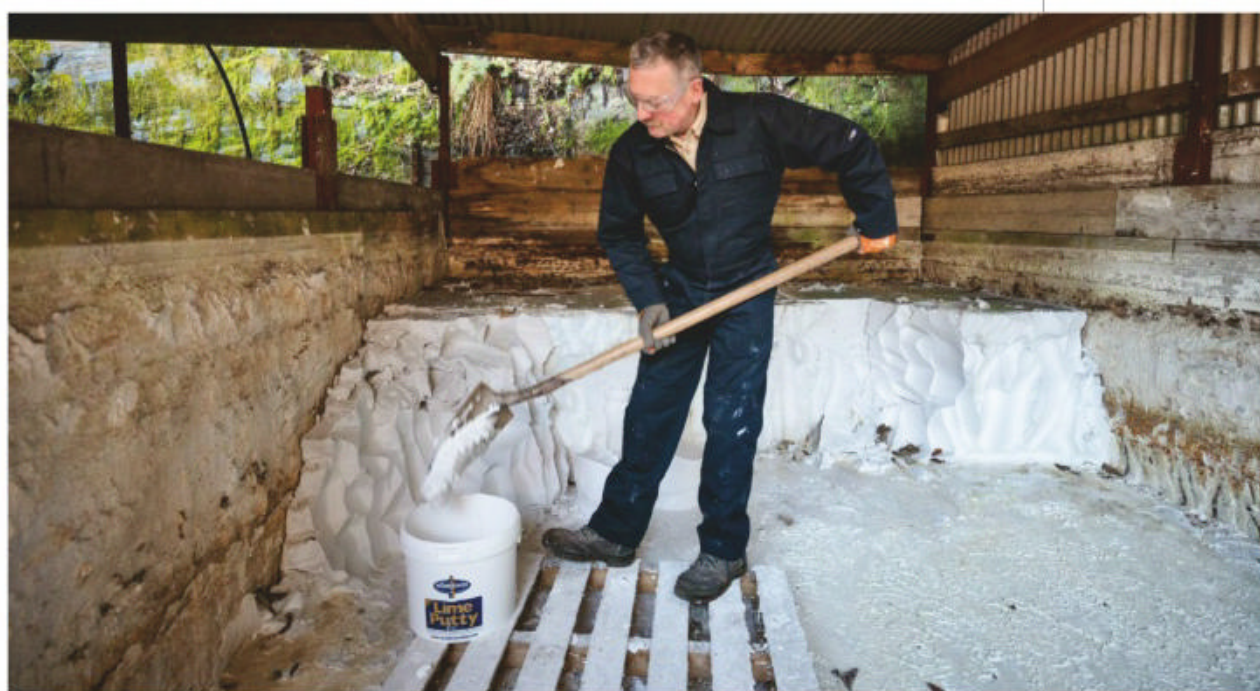
ON-SITE BUSINESS The lime plant set up on site to supply the renovation is now a family business, Roundtower Lime ( www.roundtowerlime.com ).
