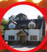
New Build Home
