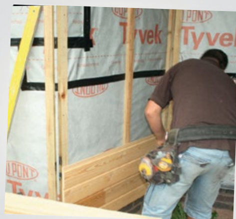
11.30am - Bruce fixes the timber boards
