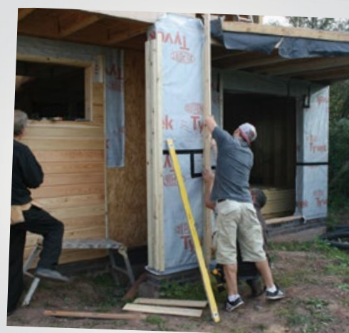
9.43am - Measuring up for the weatherboarding
