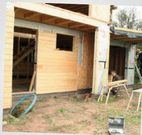
12.53pm - Finishing up the wall before lunch
