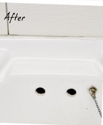
The gap is now neatly sealed.
