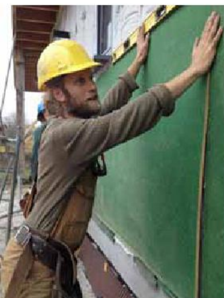
Wood fibre board sheathing can replace OSB and foam insulation with a single installation, and at a thickness of 1.5 inches adds R-4 to the building. This material also sequesters carbon.
