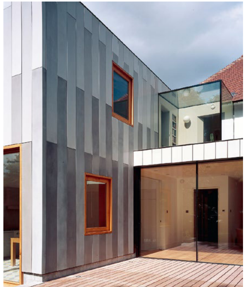
Above: Concrete Cladding
