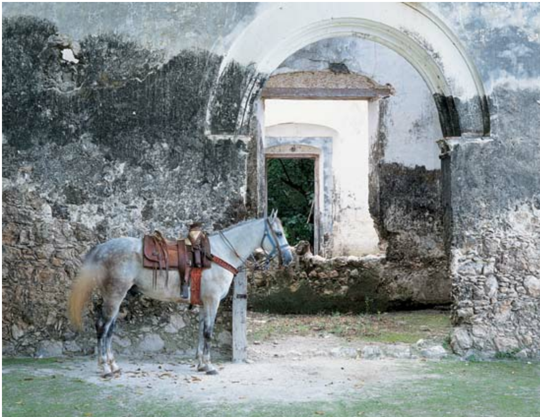
Standing as a testament to its working past, the Casa de Máquina reveals graceful architectural details. Hacienda Uayamón.
