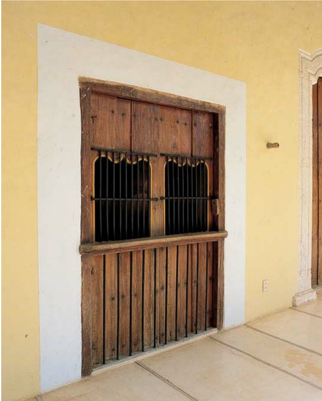
At Hacienda Itzincab Cámara many of the doors feature small window openings for increased ventilation and light. Simple wrought-iron grilles add protection.
