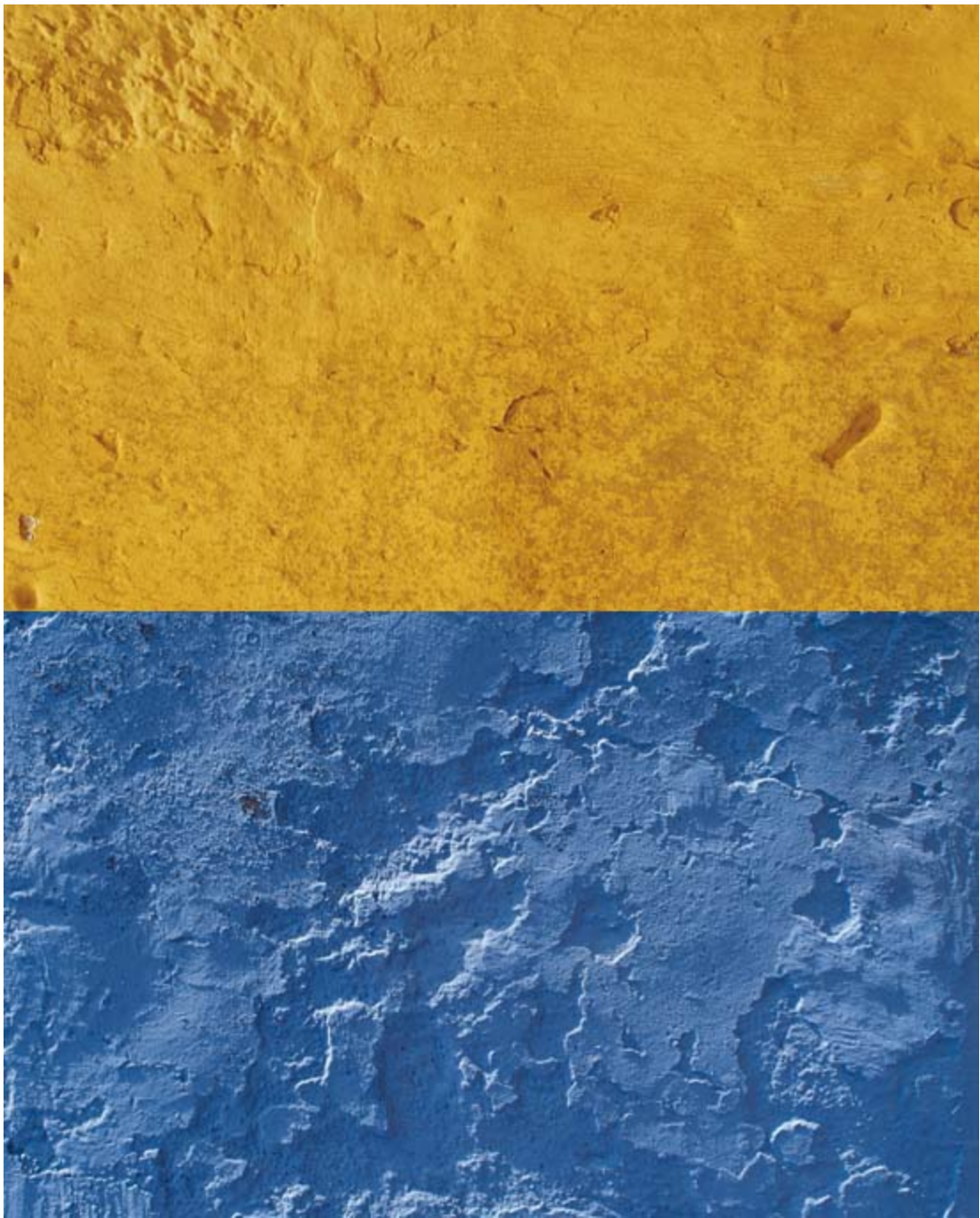
Restored old hacienda walls painted in traditional yellow ocher and Mayan blue tones.
