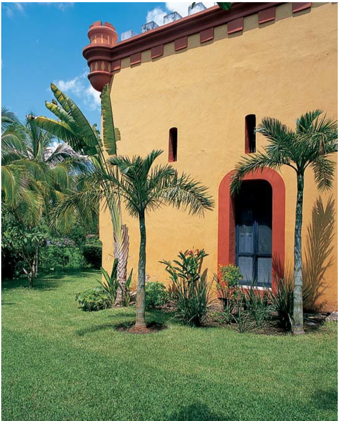
Above and Below: Color enlivens the castellated facade of Casa Nueva. Restoration and design by architect Salvador Reyes Ríos and designer Josefina Larraín. Casa de Máquina de Hacienda Sacchich. Yucatán.
