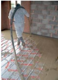
Kenny's liquid screed is perfect for under floor heating, it allows the screed to totally encapsulate the heating pipe leaving no voids around the pipes. Thus giving a much better performance to the heating system than a dry conventional screed.
