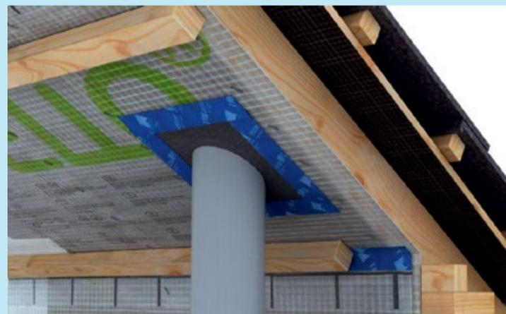
If pipes or cables penetrate an airtight layer they must be securely sealed. One solution is to use **airtightness grommets**, such as the Pro Clima ROLFLEX and KAFLEX, which provide a tight, flexible fit.
