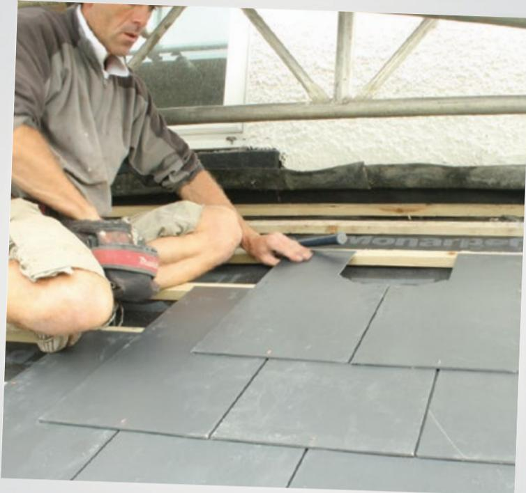
*12.15pm - Two slates are cut ready for the installation of a vent slate*
