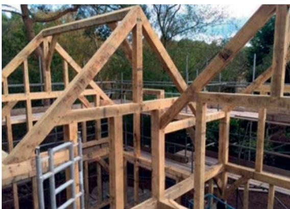
With the frame up, the last couple of weeks have since seen the SIPs (structural insulated panels) installed, extra insulation added, battening begun and the oak frame sandblasted. Oh, and we also planted 1,000 bluebell bulbs in the woods and sowed 20,000 bluebell seeds.
