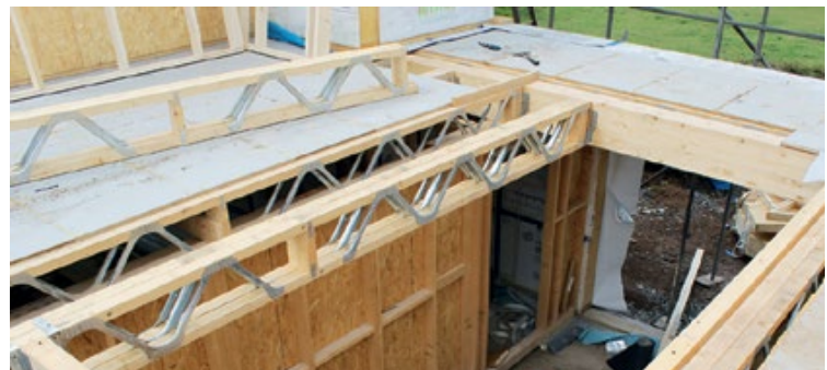
STRUCTURAL TIMBER ASSOCIATION X2
