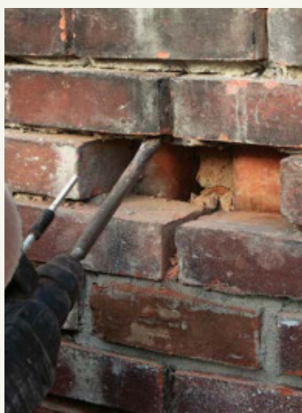
Slice and dice. When removing field bricks, break the brick vertically into 1-in. pieces using a hammer drill chucked with a 1-in. chisel. Only go about as deep as the joints are excavated around the brick to avoid putting pressure on the surrounding bricks. Then break the vertical slices in half horizontally, leaving a grid of small pieces.
