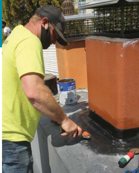
Flash the top. Once the termination bars are in place, we prime the areas around them and cover them with uncured flashing tape, which is more flexible but not as long-lasting as the cured version. It must be rolled like other seams and transitions. The skinny roller in the foreground is for corners.
