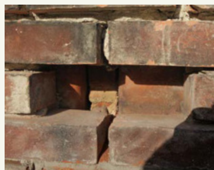
Reason for care. Many chimneys are only one-wythe thick, with the masonry flue right behind it. Be extremely careful not to damage flues, especially if they're in active use.
