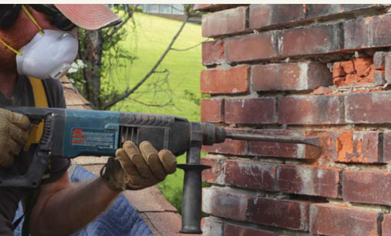
Slice and dice. When removing field bricks, break the brick vertically into 1-in. pieces using a hammer drill chucked with a 1-in. chisel. Only go about as deep as the joints are excavated around the brick to avoid putting pressure on the surrounding bricks. Then break the vertical slices in half horizontally, leaving a grid of small pieces.
