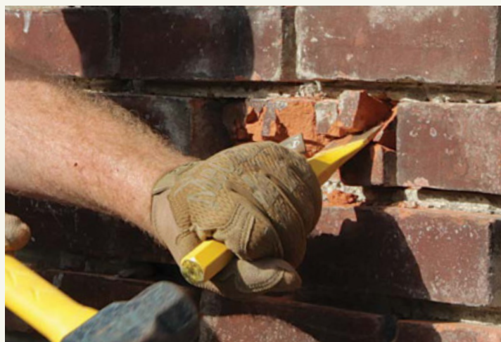
Chisel 'em out. Use a hammer and wide masonry chisel to slice out the pieces of broken brick. Removing the top half of the broken-up brick first provides room and relief to easily remove the bottom half without pressuring and possibly breaking the surrounding brick.
