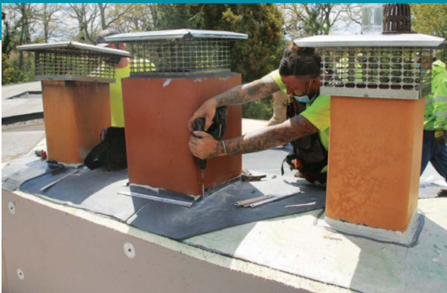
Fix a leaky chimney. The chimney can't be seen from the ground, so it made sense to insulate it and cover it with EPDM so it could be more reliably flashed and in order to reduce thermal bridging. The insulation is held to the masonry with concrete screws. Drive anchors hold the termination bars.
