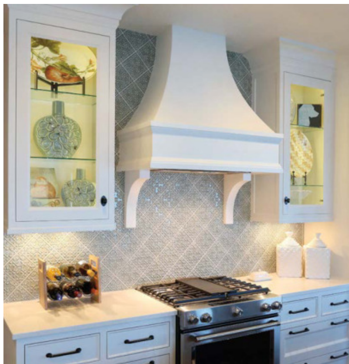
Mind the gap. Code requires at least 30 in. of clearance from the top of a cooktop to combustible materials above it, which can factor into the range-hood design with custom cabinets.
