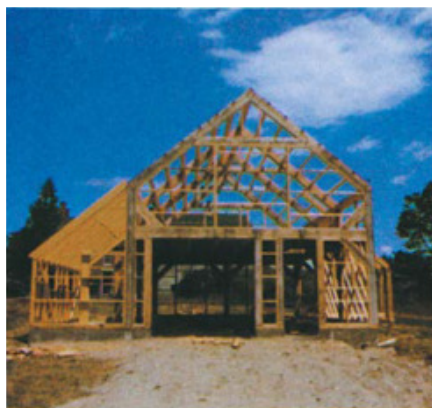
A modern saltbox under construction in upper New York state. Framing is basically traditional, but the common partition between Cape and shed has been replaced by posts and beams to open up the interior. Photo: Patsy Hennin
