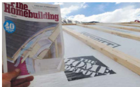
That was fast! Reader Nico Foster has already adopted and completed the insulated roof assembly published just two issues ago on his own build.
