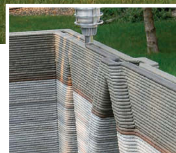
Like icing from a pastry bag. The 3D concrete printer lays down row after row of concrete directly onto the building site.
